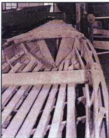
WA-200-7 Interior detail of Cama Beach No. 55
