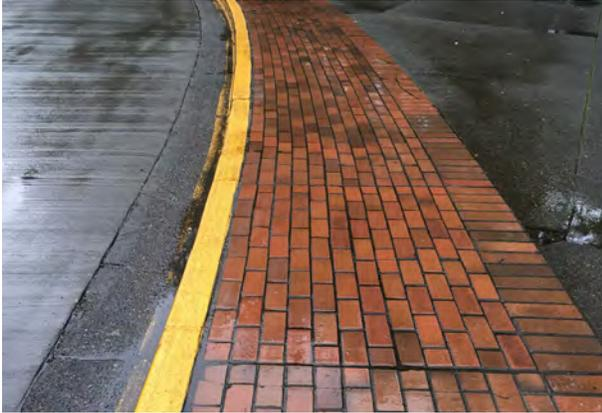
Photo 3.7. (upper left) Example of asphalt paving meeting brick sidewalk.
