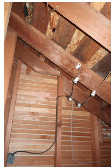
Figure 343. Roof framing access from within closet.
