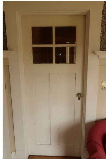
Figure 229. Detail of glass panel door between Hall and Original Dining Room..
