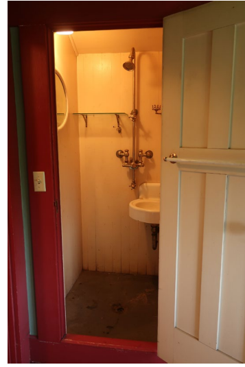
Figure 347. View looking south into Bath 2.
