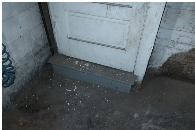
Figure 170. Detail of step and door leading to the Basement Stair.
