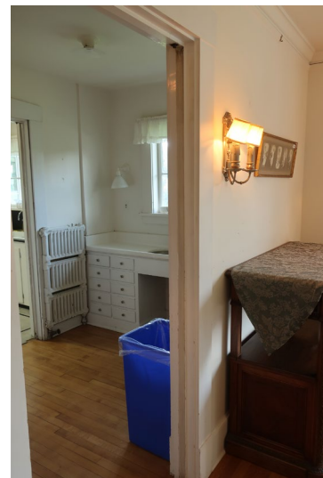
Figure 289. Detail of door opening to pantry with remaining double-swing hinge hardware.
