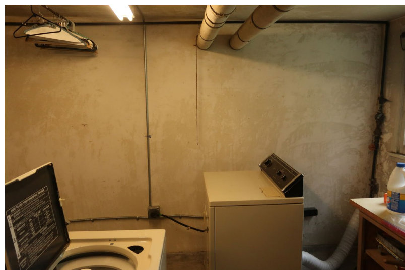
Figure 188. View looking west at north end of the wall.
