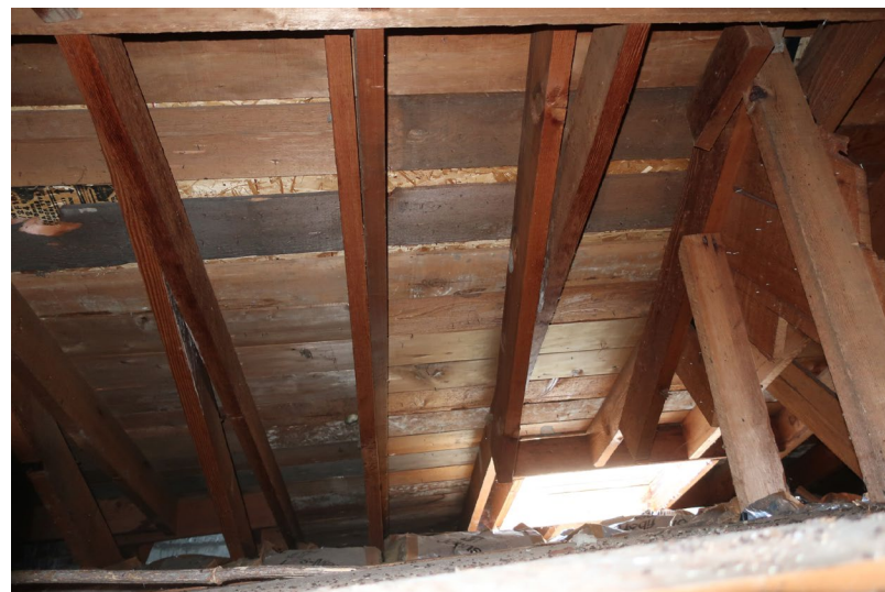
Figure 412. View looking west from inside attic, with skylight visible.
