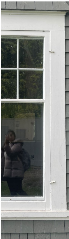
Figure 98. Wood window detail.
