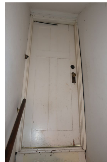
Figure 155. View looking south at the upper door to the Kitchen.
