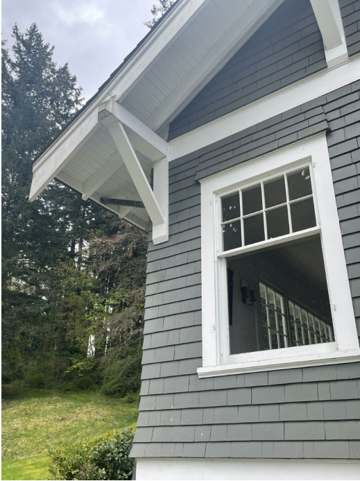
Figure 69. Detail of the northeast corner, showing the typical cedar shingle siding with flared wall base at the water table, flared drip edge cap above a 8:1 double hung wood window, flared barge board at the roof eave, exposed rafters and beadboard soffit/sheathing, and non-structural gable end knee braces.
