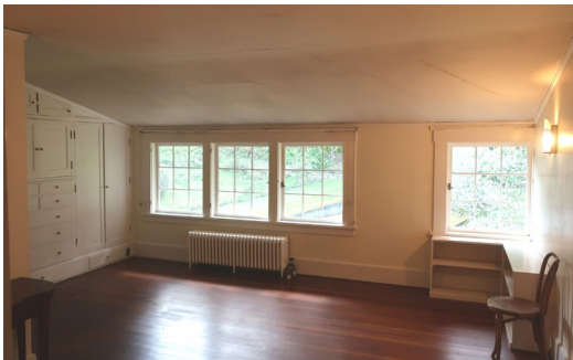
Figure 51. Room 6 looking east with casement windows, sloped plaster ceiling, and built-in wardrobe.
