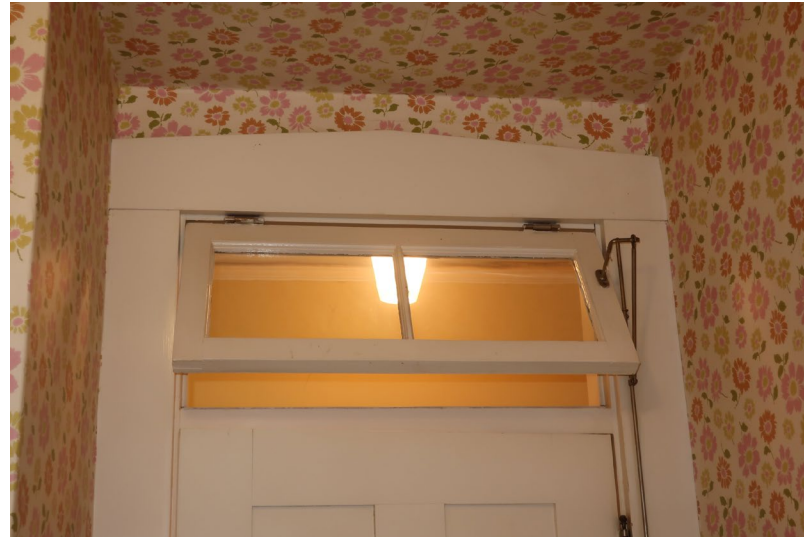
Figure 242. Detail of operable glass transom.
