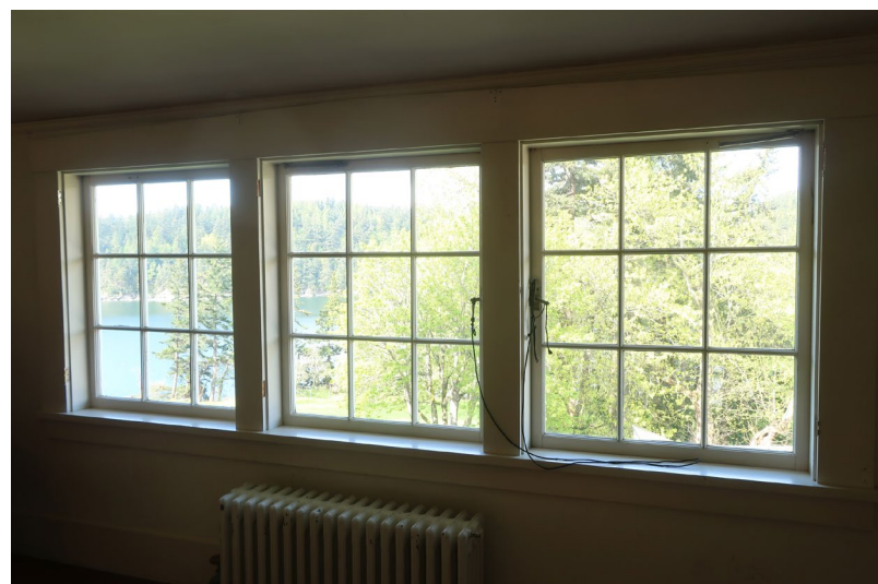
Figure 376. Detail of ganged casement dormer windows.
