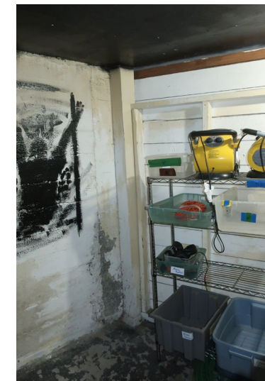
Figure 207. View looking southwest.
