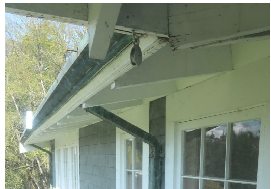
Figure 60. Detail of west facade dormer, with copper gutter and downspout.
