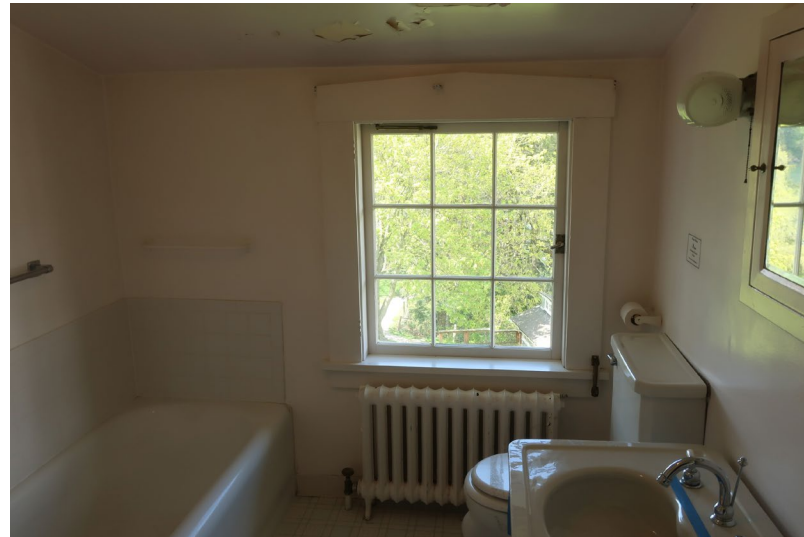
Figure 361. View looking west at dormer window, radiator, and original plumbing fixtures.
