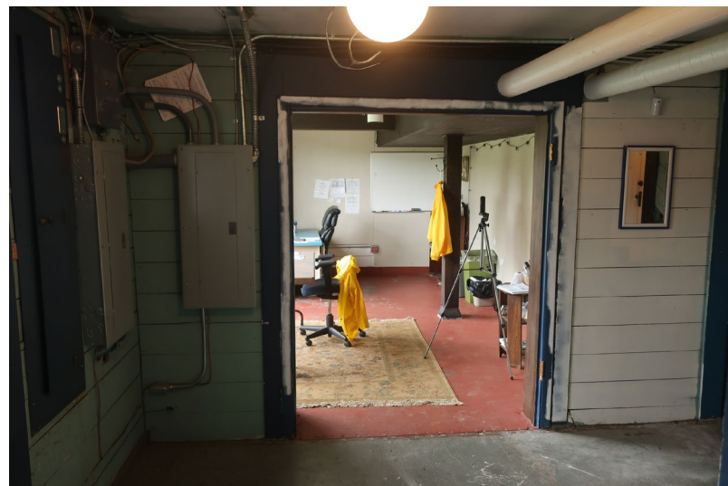
Figure 159. View looking north at the double door opening into the Office. Note exposed insulated radiator piping at the ceiling, which extends into plywood soffits in the Office.
