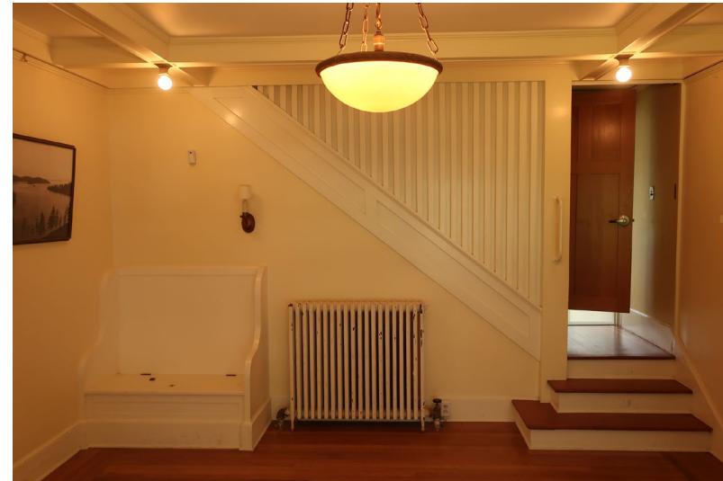
Figure 211. View looking west, showing the firewood dumbwaiter bench, radiator, and stair. The open door has been replaced, and former double-swinging door is missing. The wall behind the bench was originally an opening to the top of the basement stair.
