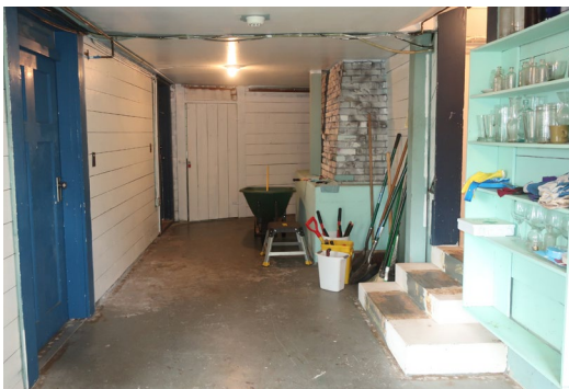
Figure 80. Bare, smooth concrete floor at Basement Hall. Note the remnant of a stair carpet runner on the concrete steps leading through the original north wall at right.
