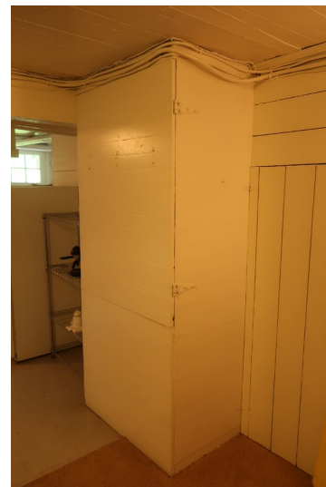
Figure 111. Detail of firewood dumbwaiter chase (secured shut).
