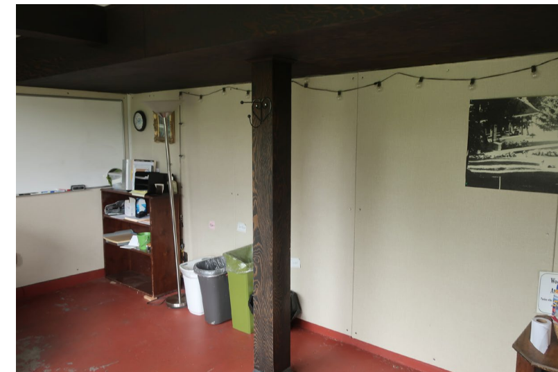
Figure 178. View looking northeast. Floor is painted concrete (ca. 2007, per Farm Records on City Website).
