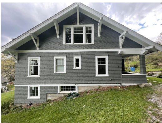
Figure 44. South facade, looking north.
