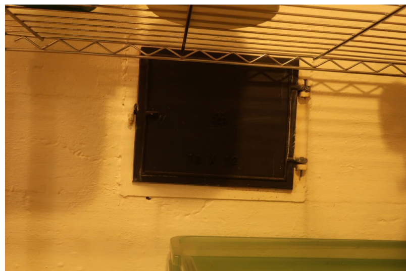
Figure 110. Detail of chimney ash access.
