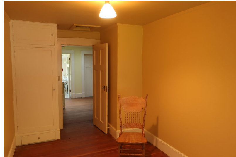
Figure 408. View looking west, with built in wardrobe at left, hall door at center, and the chimney flue from the Entry Hall chimney to the right of the door. There is a flue damper vane on the wall behind the door. Also note attic access scuttle above the door.
