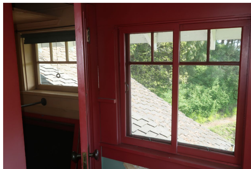
Figure 358. View looking south at stepped windows along sloped roof.
