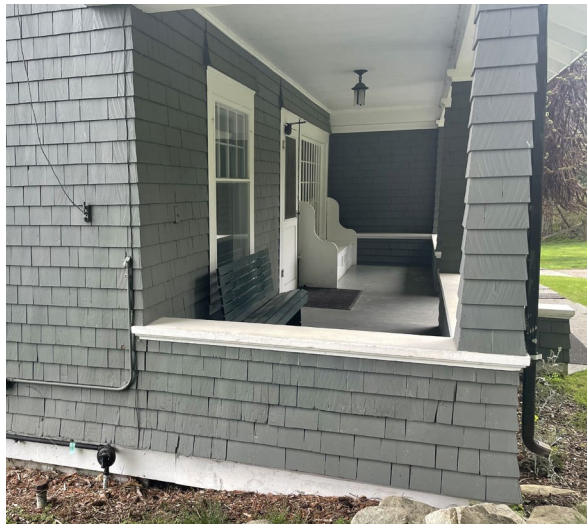
Figure 73. Detail of the East Entry Porch looking south, with original ceiling light fixture, bench, and front door and screen.
