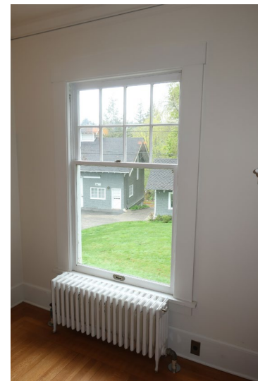
Figure 298. Detail of typical window and radiator.
