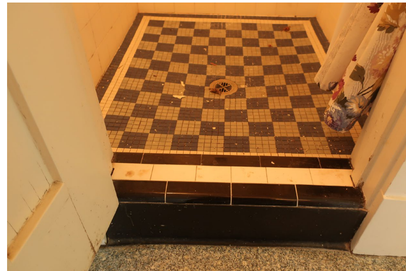
Figure 384. Detail of tiled floor and curb of shower room.
