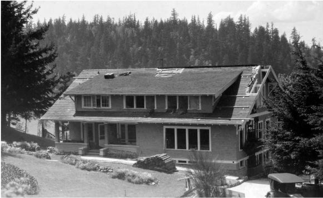
Figure 24. ca. 1923 exterior, looking southwest at the east and north facade during construction of the addition. Wood shingle combing is visible at the ridge. (Courtesy CPNWS, Gates Family Papers)
