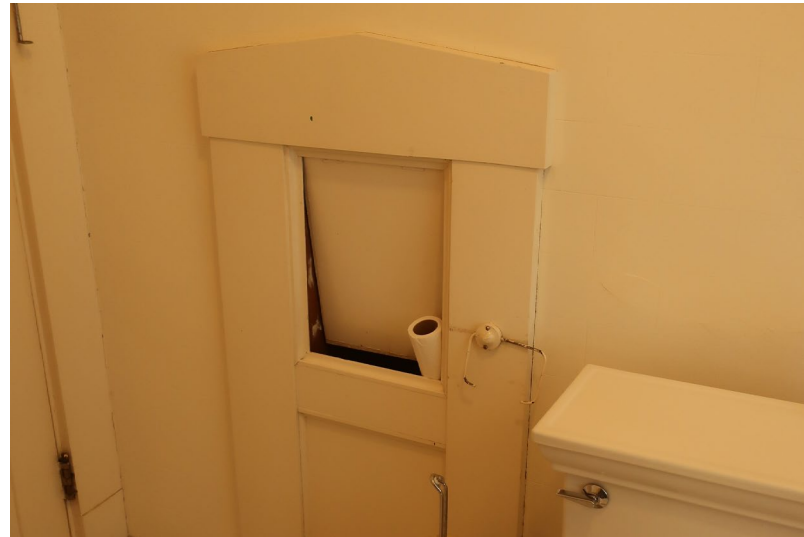
Figure 239. Detail of linen chute door on south wall behind the door.
