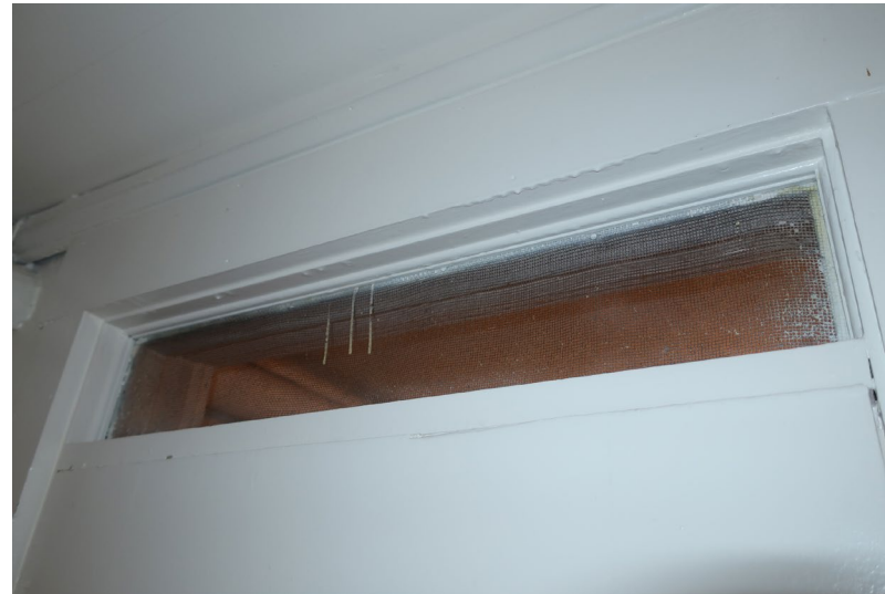
Figure 123. Detail of screened transom above door.
