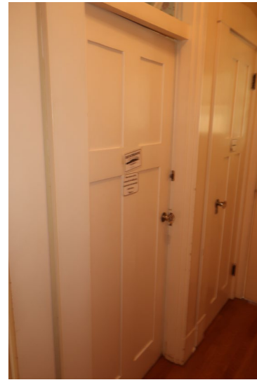
Figure 230. Detail of Washroom door.
