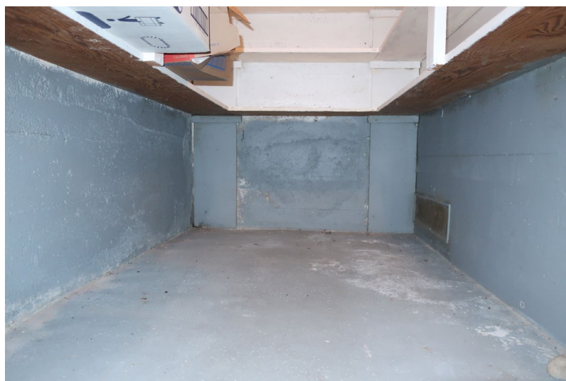
Figure 126. Detail of painted concrete floor and exterior wall base.
