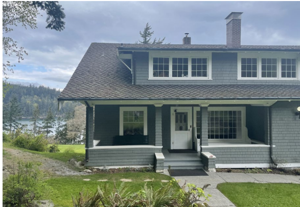
Figure 72. View of the East Entry Porch.
