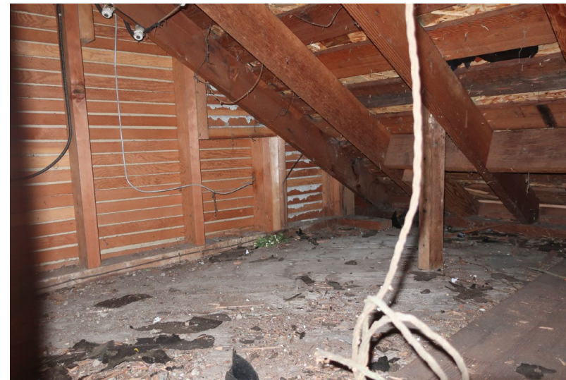
Figure 340. Roof framing access from within closet.
