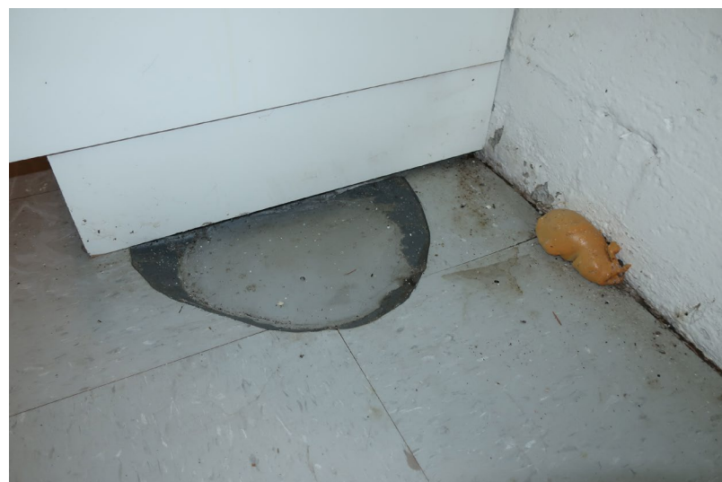
Figure 118. Detail of VCT flooring with floor drain sealed shut.
