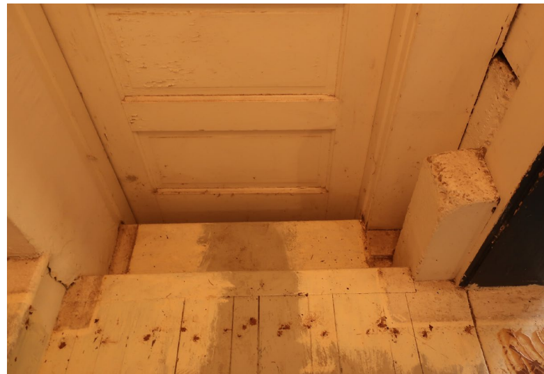
Figure 151. View looking west at the step down into the Utility Room.
