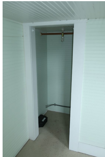
Figure 136. Detail of closet opening
