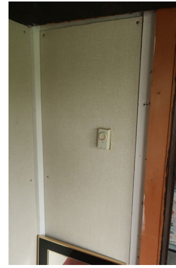
Figure 176. Detail of acoustic office furniture panelling typical of the wall surfacing.
