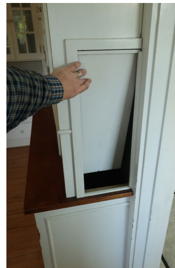
Figure 282. Detail of linen chute door.
