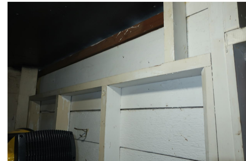
Figure 205. View looking southwest at wall framing and shiplap siding.
