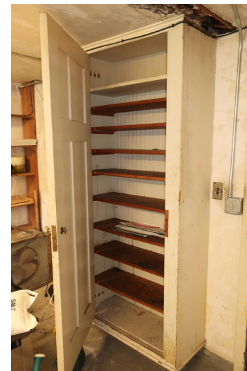
Figure 190. Detail of built-in cabinet with raised floor, and small circular vents in side wall.
