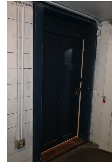
Figure 198. Detail of exterior side of door.
