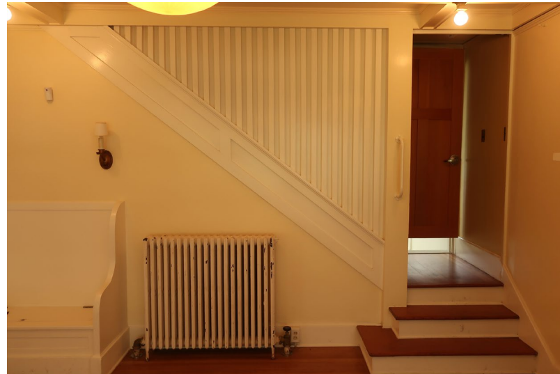
Figure 301. View looking west at the cascading bottom steps, and 2" balluster with infill panel behind..
