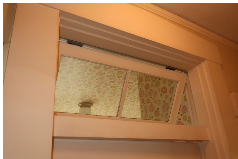
Figure 235. Detail of Washroom door operable glass transom.
