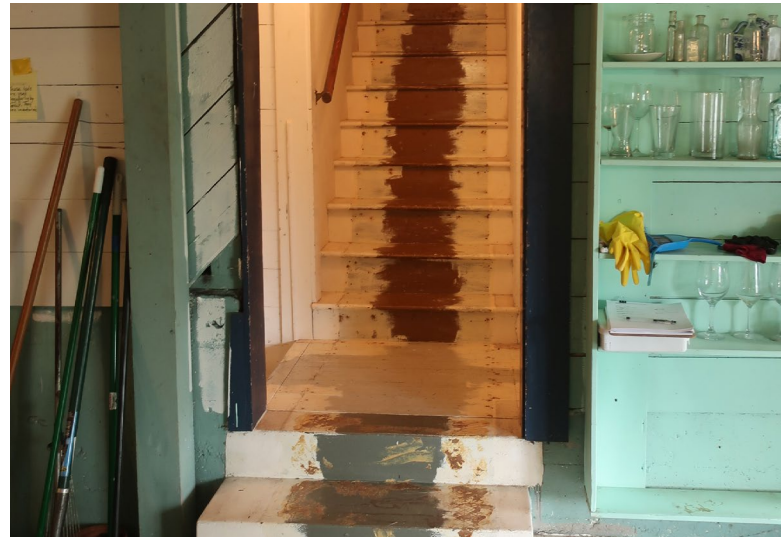
Figure 148. View looking south, door opening was cut through original exterior wall.
