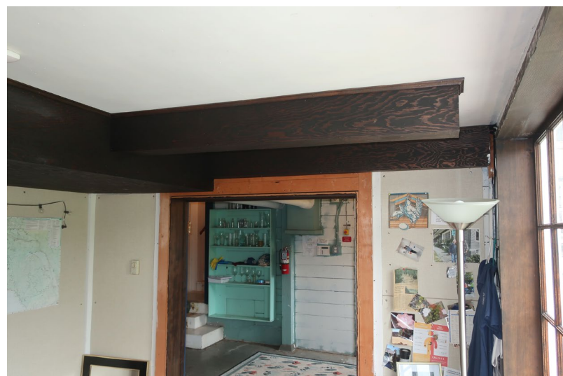
Figure 179. Detail of retained plywood soffits.
