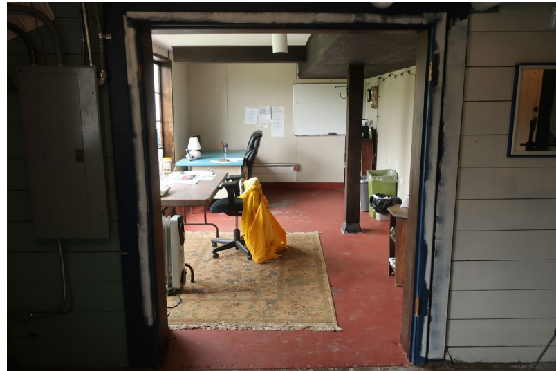
Figure 174. View looking north through double door opening.
