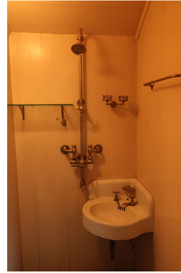
Figure 348. View looking south at the sink and shower assembly.
