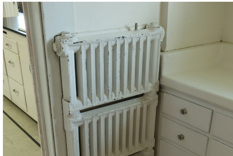
Figure 278. Detail of wall mounted, stacked cast iron radiators.
