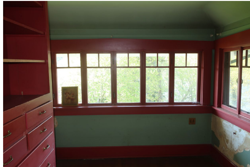
Figure 353. View looking west.
