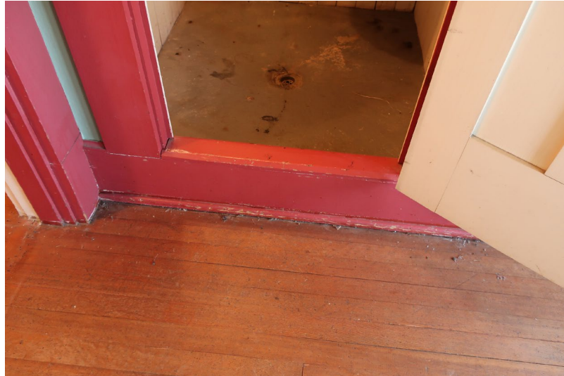
Figure 346. Detail of wood curb into shower stall.
