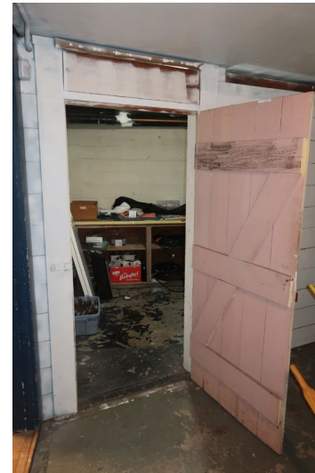
Figure 203. Detail of door.
