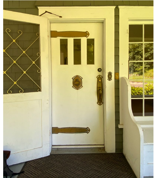
Figure 57. Detail of east entry door, with decorative hardware and grillework screen door. (Courtesy City of Bellingham, Michelle _____)
