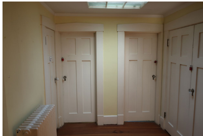
Figure 312. View looking west at doors to the janitor closet on left (south) wall, Bath 3, Bath 4, and double closet doors. The skylight laylight is visible above..
