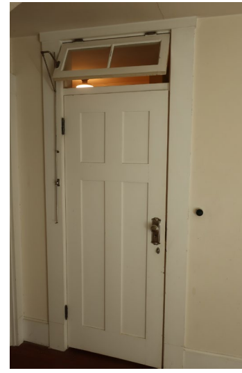
Figure 321. Detail of hall door with glass transom.
