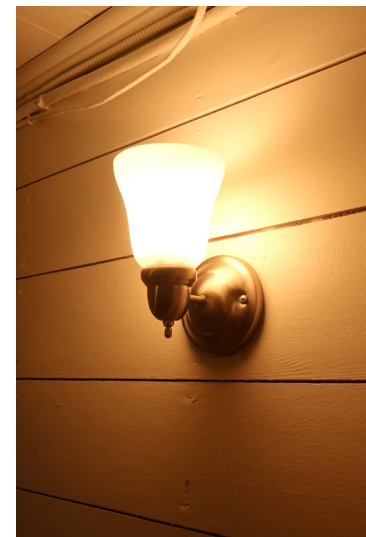
Figure 112. Detail of original wall sconce light fixture.
