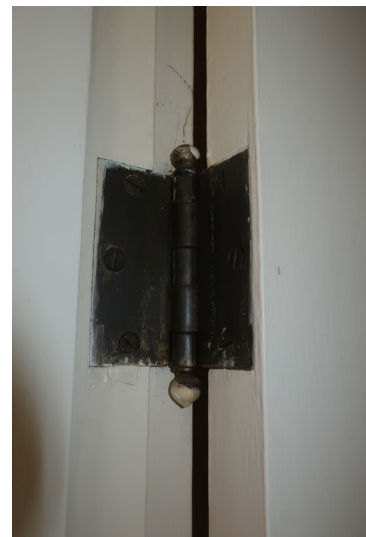
Figure 236. Detail of door hinge.
