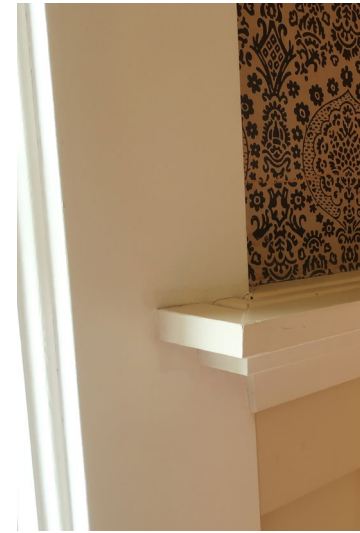
Figure 250. Detail of plate rail top cap at the wood panel wainscot.
