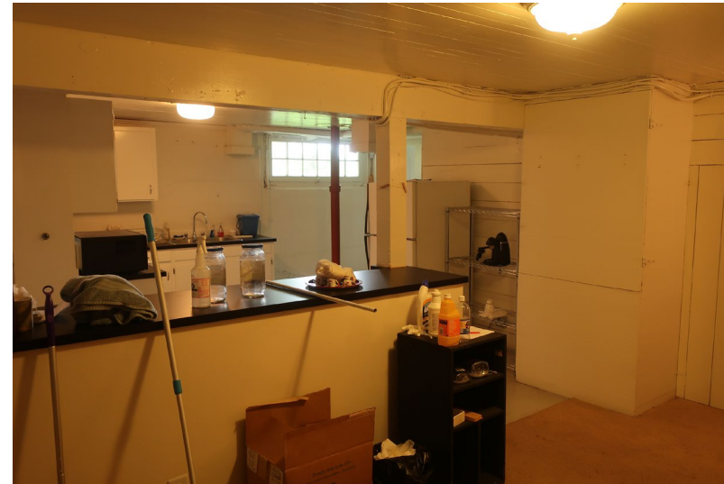
Figure 106. View looking southwest. The cabinet at right reportedly contains a dumbwaiter for firewood.
