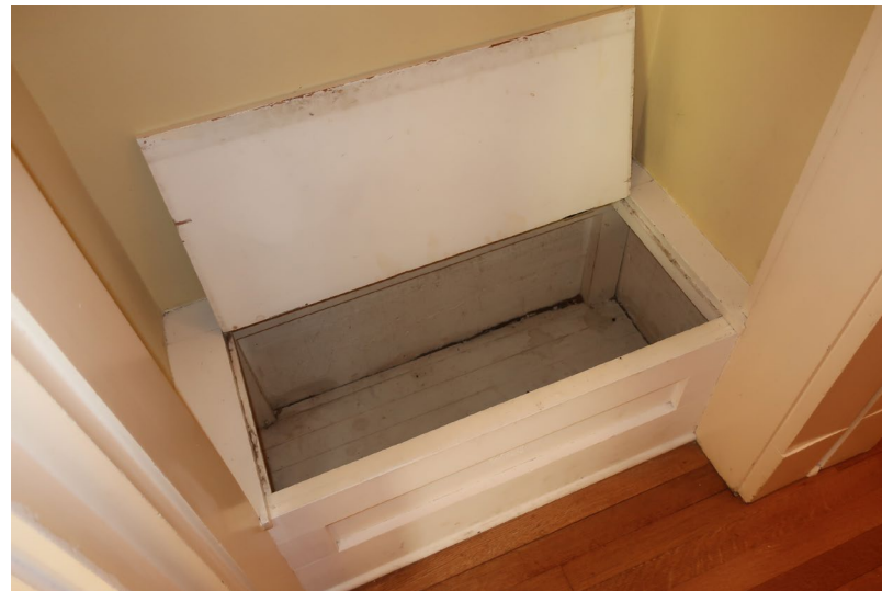
Figure 233. Detail of storage hatch in bench under coat closet niche.
