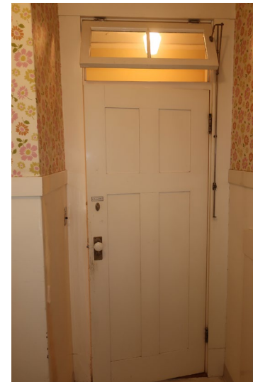
Figure 246. Detail of interior side of door.
