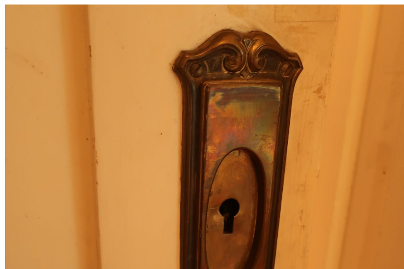
Figure 224. Detail of door hardware.
