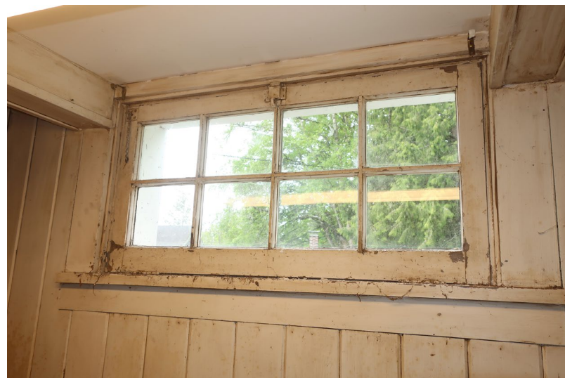
Figure 197. Detail of operable window.
