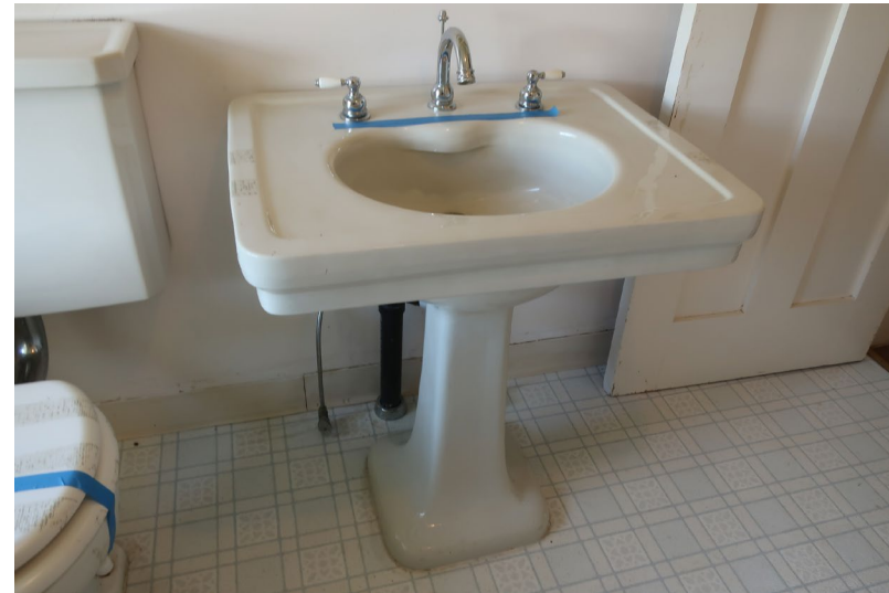
Figure 362. Detail of decommissioned sink and toilet.
