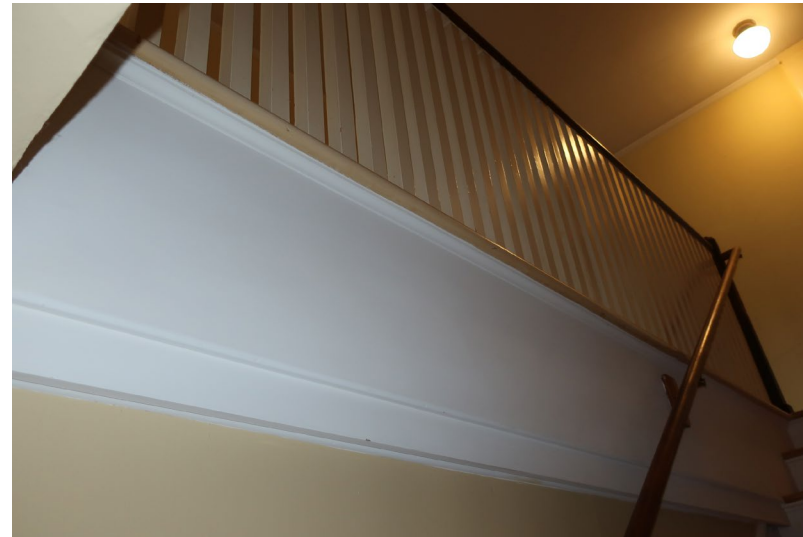
Figure 302. Detail of trim and railing at Second Floor level.
