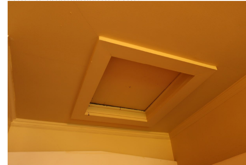
Figure 411. Detail of attic access scuttle.
