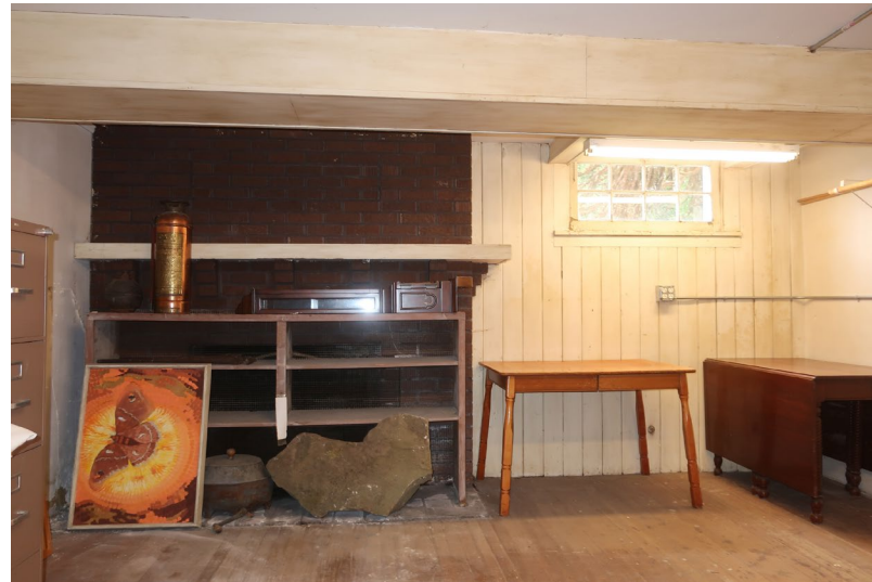
Figure 192. View looking north, with brick fireplace behind storage at left, and operable window at right.
