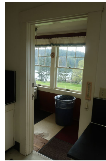
Figure 268. View looking southwest into the Back Porch from the Kitchen.
