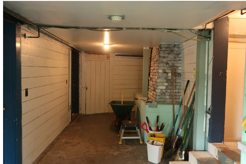
Figure 157. View looking east. Original exterior north wall is at right, with battered brick chimney.
