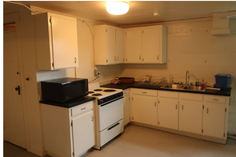
Figure 115. View looking southeast at the counter and cabinetry, which is not original.
