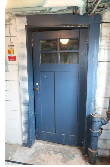
Figure 167. Detail of Utility Room door.
