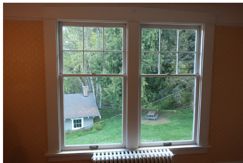
Figure 395. Detail of wood windows.
