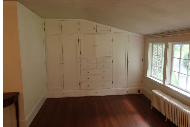
Figure 400. View looking north at built-in cabinetry.
