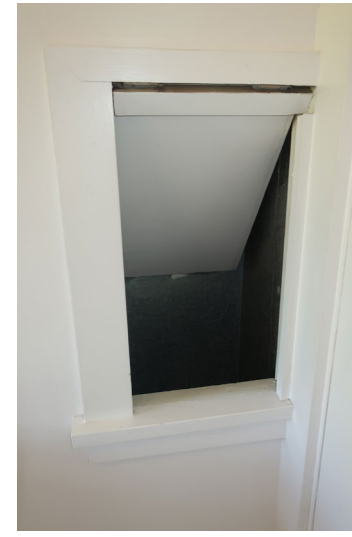
Figure 363. Detail of linen chute door.
