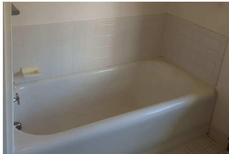
Figure 364. Detail of tub.
