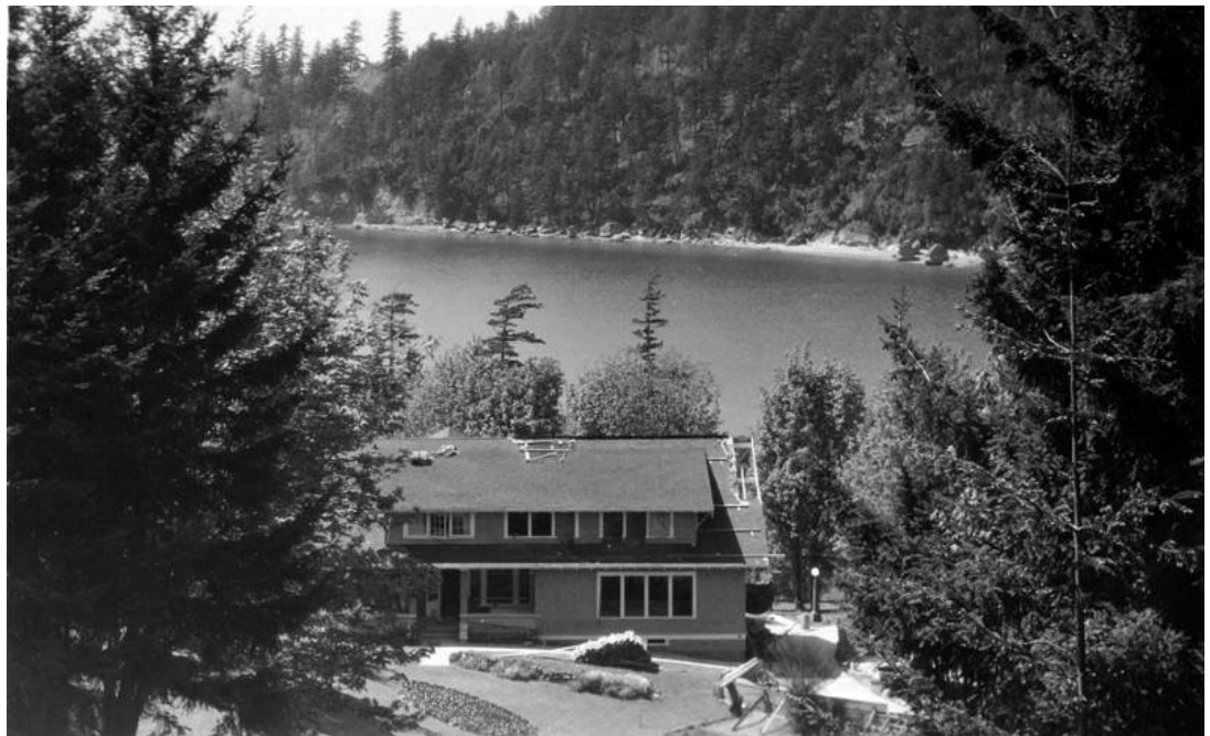
Figure 23. ca. 1923 exterior, looking west, at the east facade during construction of the addition. (Courtesy CPNWS, Gates Family Papers)
