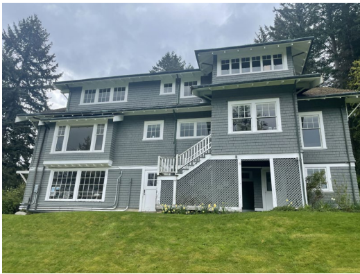
Figure 43. West facade, looking east.
