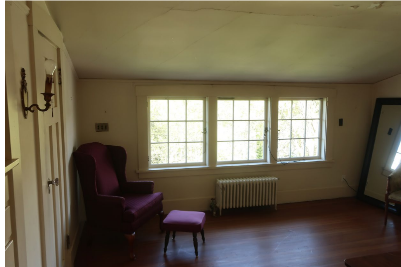
Figure 370. View looking west at dormer windows and radiator.
