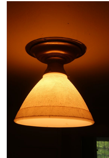
Figure 413. Detail of original light fixture.
