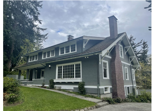
Figure 36. Looking southwest at the primary east and north facades and concrete walkway from the concrete driveway.
