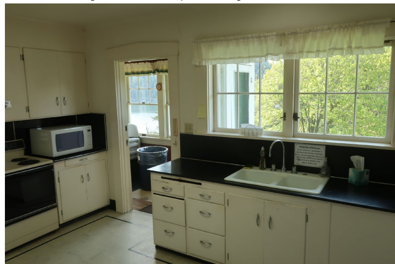
Figure 262. View looking west at laminate countertops and operable casement windows.
