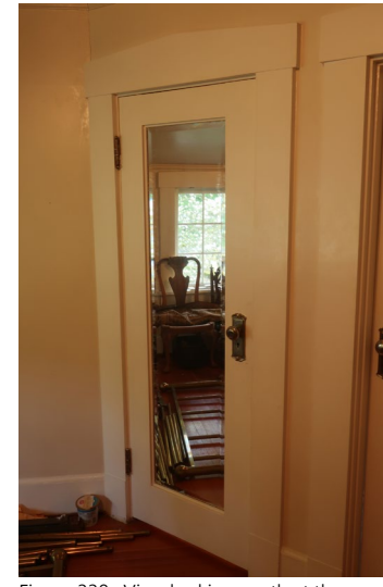
Figure 338. View looking south at the mirrored closet door.
