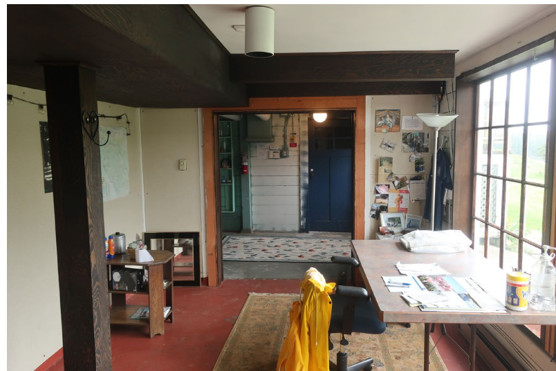
Figure 177. View looking south. Dark stained plywood soffits conceal radiator piping. There is new rough framing for a double door, without leaves.
