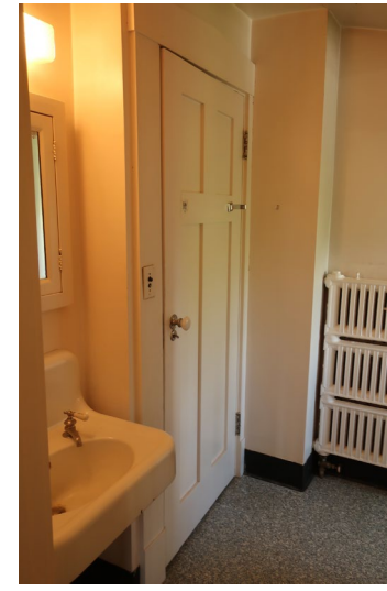
Figure 382. View looking southwest with wall mounted radiators, and hall door.
