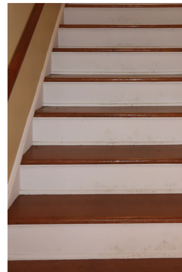
Figure 305. Detail of painted risers and stained fir treads.
