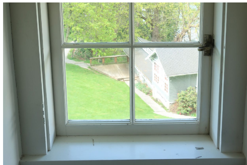
Figure 383. Detail of casement window.
