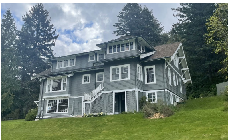
Figure 58. West facade, with hip-roofed "tower," and operable strip windows.
