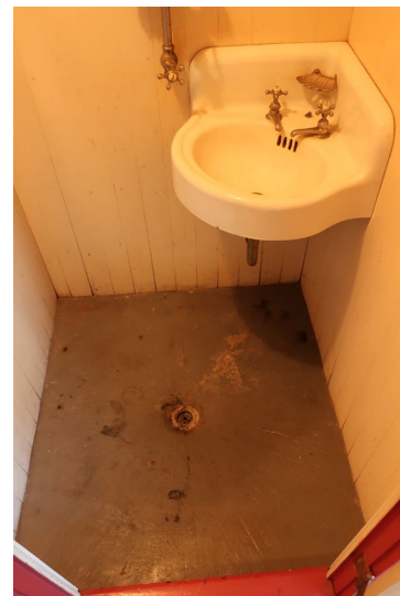
Figure 352. Detail of cementitious floor..
