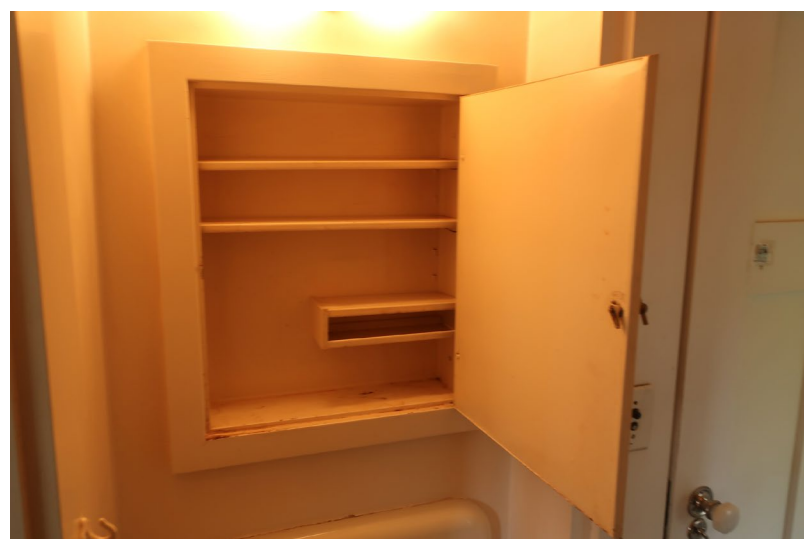
Figure 386. Detail of medicine cabinet.
