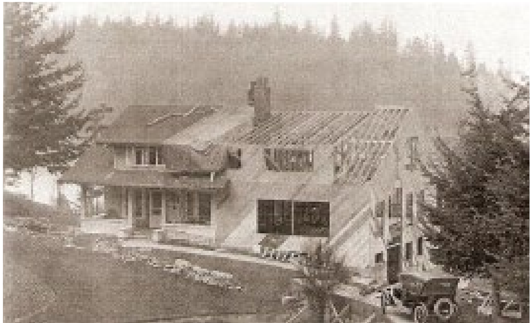
Figure 22. ca. 1923 exterior, looking southwest at the east and new north facade during construction of the addition. The wood framing and diagonal wood wall sheathing are visible on the addition (Courtesy CPNWS, Gates Family Papers)
