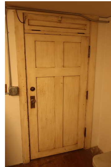
Figure 199. Detail of interior side of door, with operable solid panel transom.
