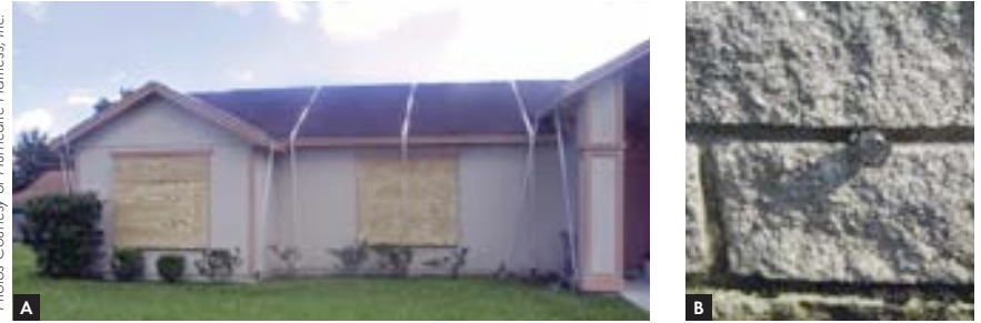
A) Roof straps installed on a home.; B) Roof strap anchor.
