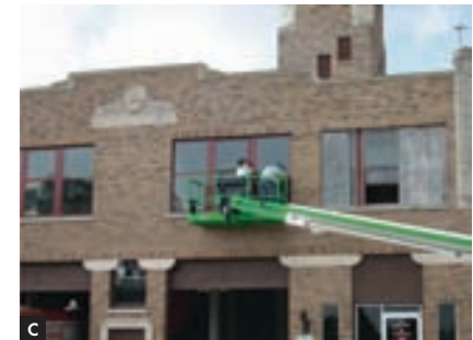
A) North-Window; B) West Wall After New Window; C) Window Installation on Facade
