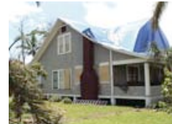
A roof tarp provides temporary stabilization.
