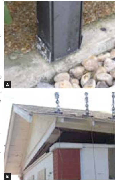
A) This column is held down by two rusty tech screws.; B) This porch on an older Florida house was enclosed. Note that the roof was resting on the brick columns with no anchor to hold the roof down.; C) Porch Roof Connection.
