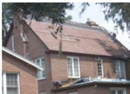
Installation of an asphalt shingle roof.
