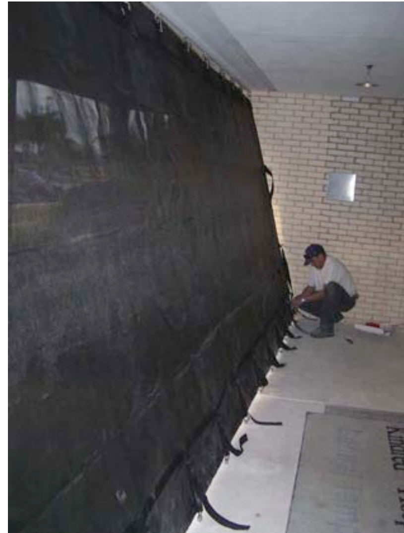
Flexible wind abatement system installation.
