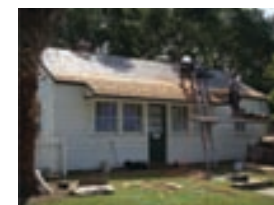
Historic photo verifies historic use of wood shingles on the roof of a 1942 WWII Coast Guard Barrack, Florida Air Museum
