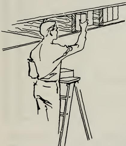
Plywood sheets (2' x 8' x 1/2" cut to fit) should be securely fastened to the joists using 2 inch, #8 screws 10 inches apart. Bricks or blocks are then packed as tightly as possible into the openings between the joists. Be sure to fill as much space as possible. To get the most protection out of this improvement, one-quarter of the basement ceiling over the best corner should be filled with bricks or solid concrete blocks.
