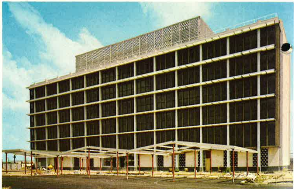
building Columbia Gulf Transmission Company Office Building location Houston, Texas architect Douglas Orr associate architect Pierce and Pierce contractor Linbeck Construction Company
