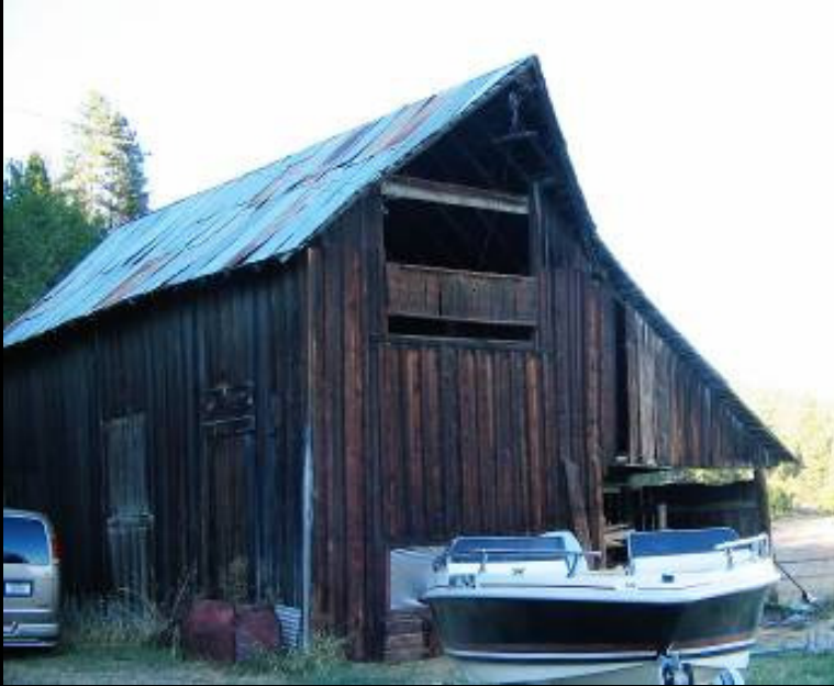
Carlstrom Barn – c.1910
