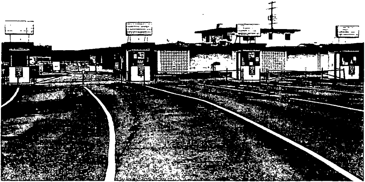
Example of the Drive-In Theater Property Type: Valley "6", Auburn, WA. PS1-133. Roll 73/Neg 1.
