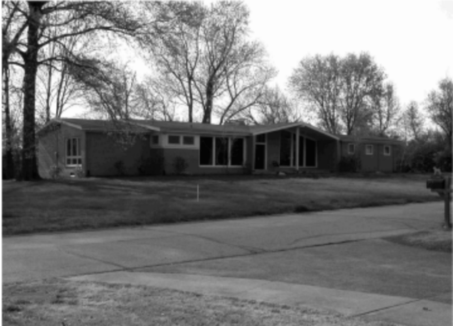
Figure 33: #11 West Ladue Estates Drive, Ladue Estates Photo by Suzanne Walch, July 15, 2008
