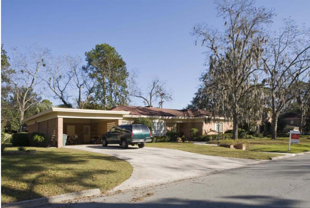
Figure 24: Lawndale Road, Nos. 1234; photographer facing west. Photo by Robert Ciucevich
