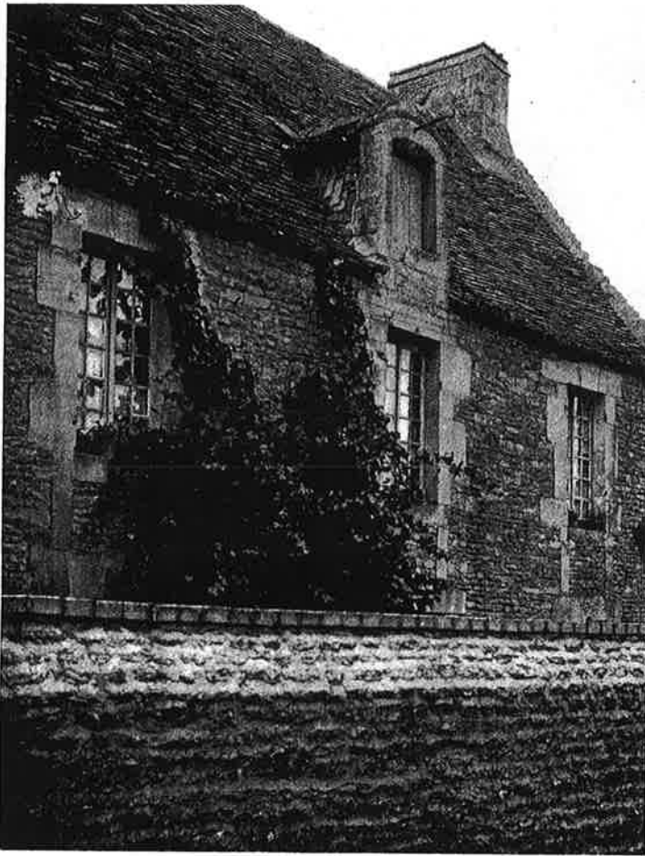
Above—A section of a small manor house of a family in better circumstances in its day than the peasant class.
