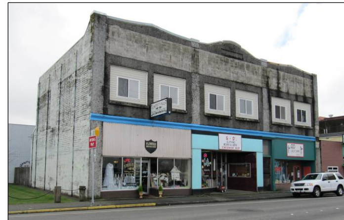
Example showing partial infill of original window openings at second story
