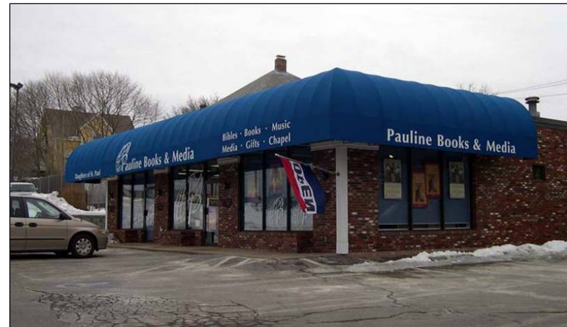
Example of an inappropriate awning, due to domel/convex shape and expanse of the single awning across multiple openings (not in Hoquiam)
