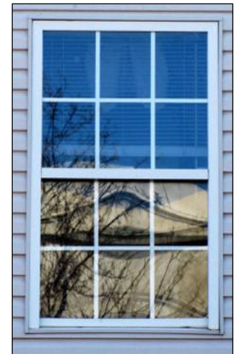
False divided lights or "snap in" muntin/mullions, which are not permitted in the District (Source: oldhouseguy.com)
