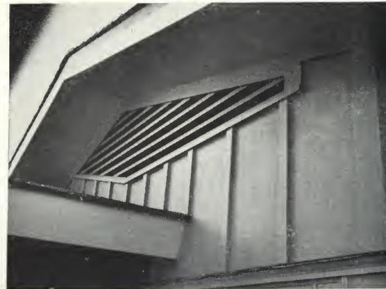
*Bedrooms are cooled in summer by big attic fan circulating air through ceiling louvers (right). In winter, Exterior plywood sheets (right, below) close louvers as ventilation for coolness is not required, although some circulation of air in attic is prerequisite to good construction. Note interesting texture contrast between smooth plywood soffits and plywood and batten siding.*
