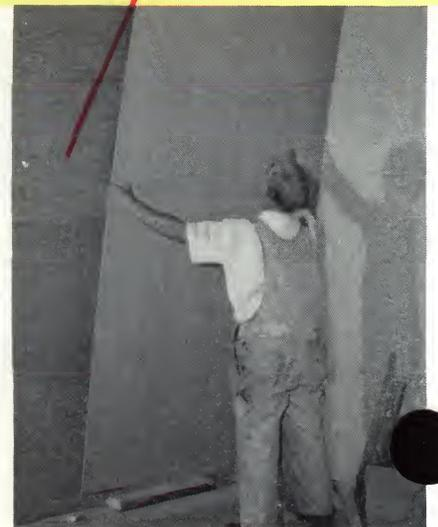
**5** Plypanel provides a firm, solid backing for finish wall surfaces, adds rigidity
