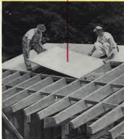
**4** Plyscord roof sheathing is easy to apply, provides superior base for roofing
