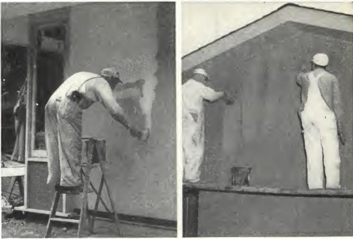
Exterior plywood siding first got a white priming coat (above), then a solid coat of flat apple green. After second coat was dry, a coat of earthy brown was applied. Before it was dry, it was dry-brushed to permit green to show through. Trim got a standard 3-coat paint job.
