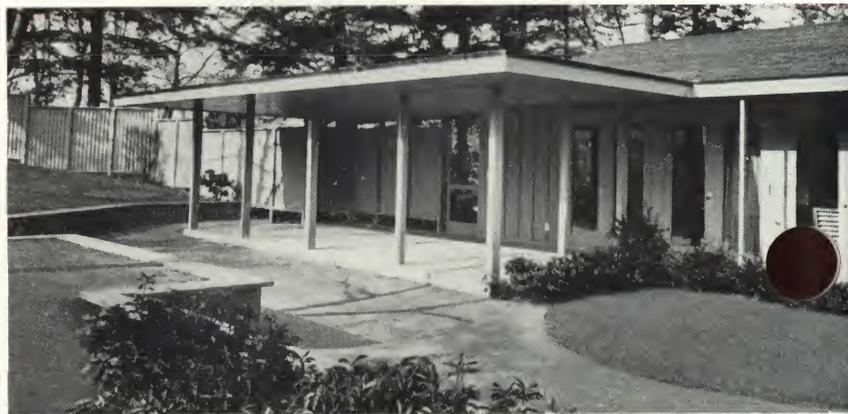
*Smooth, unbroken line of Exterior Plyshield porch ceiling continues out into soffits under eaves (above).*
