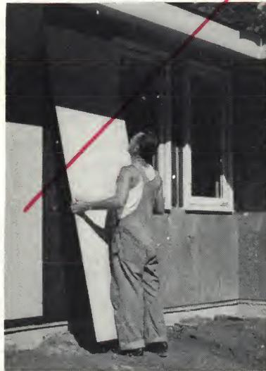
**3** Plyscord wall sheathing adds warmth, extra strength and rigidity, saves labor
