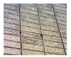
Unusual and textured masonry surfaces were utilized. Often as a contrast to smooth metals and sheets of plate glass. Brick was often stacked in a vertical bond. This provided clean vertical lines for the modern aesthetic.
