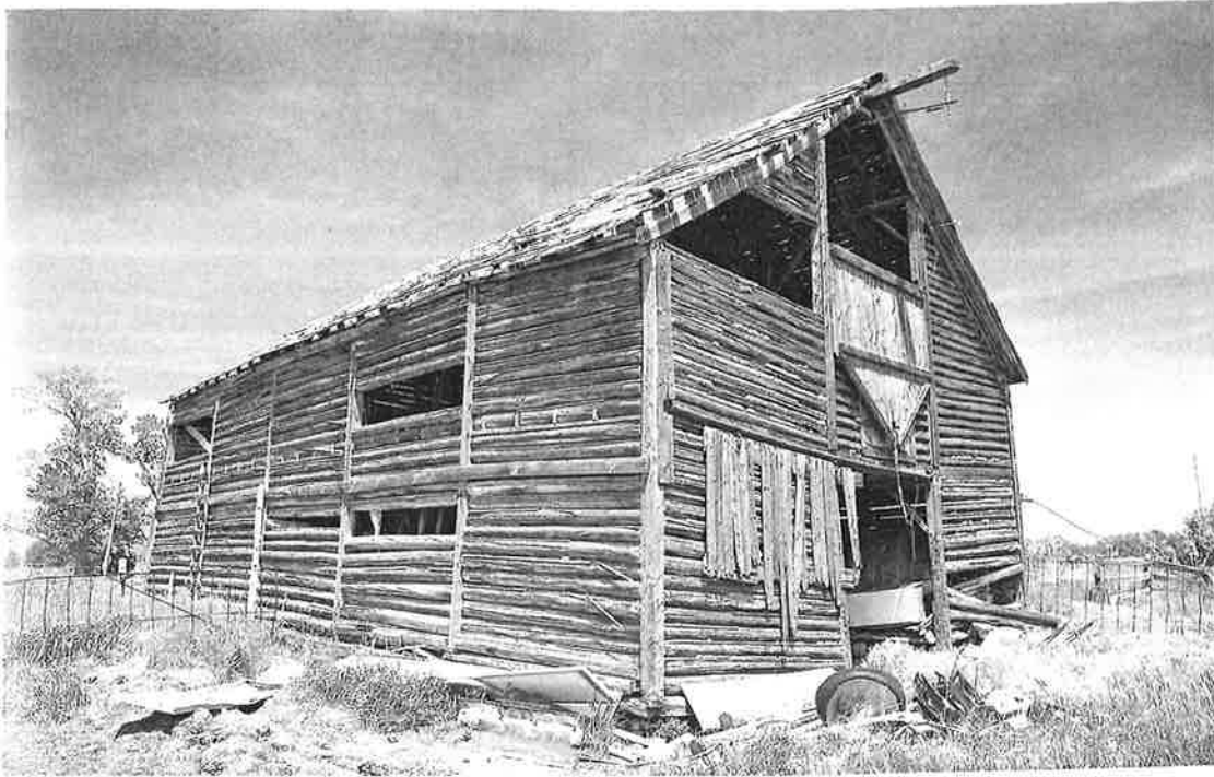
Figure 4. Log infill barn located about six miles southwest of the Montana State Agricultural College Experiment Station in Bozeman, circa 1895. Photograph by Maire O'Neill Conrad, 2017.
