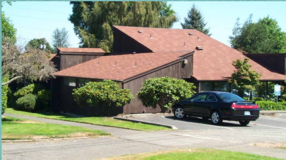
J Street Medical Office Tacoma, 1976
