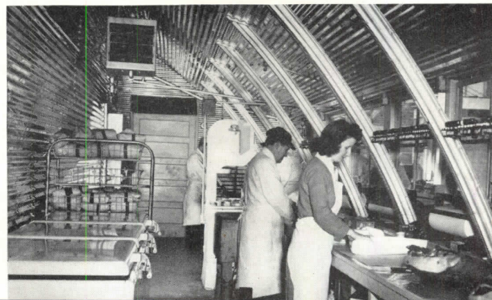
Processing room of a frozen-food locker plant in New Jersey has aluminum interior sheathing to reduce deterioration and maintenance. Note dormer and preparation-counter space so organized that arched ribs do not interfere.
