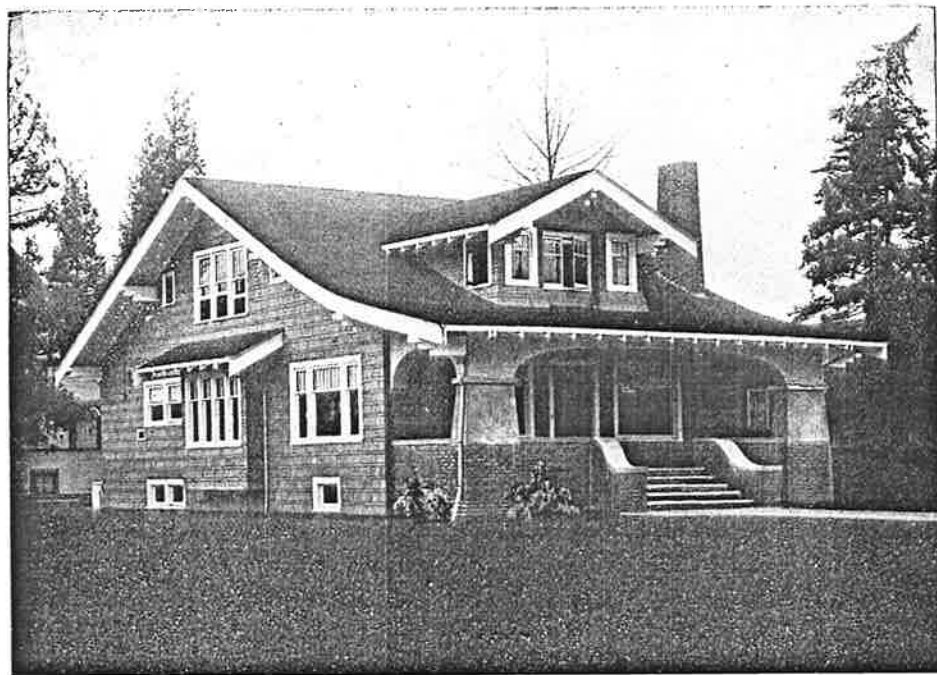
524—Another extremely popular design of five rooms on the ground floor with two bed rooms, one 14 by 14 feet, the other 10 feet 6 inches by 14 feet and sleeping porch of ample size on the second floor. The fireplace is enclosed in an angle nook with seats on either side. Large, roomy closets are provided for all the bed rooms and the bath room is located convenient to all rooms. The plan calls for a brick flue in the kitchen for kitchen range and laundry stove. The furnace flue is in the fireplace chimney.
