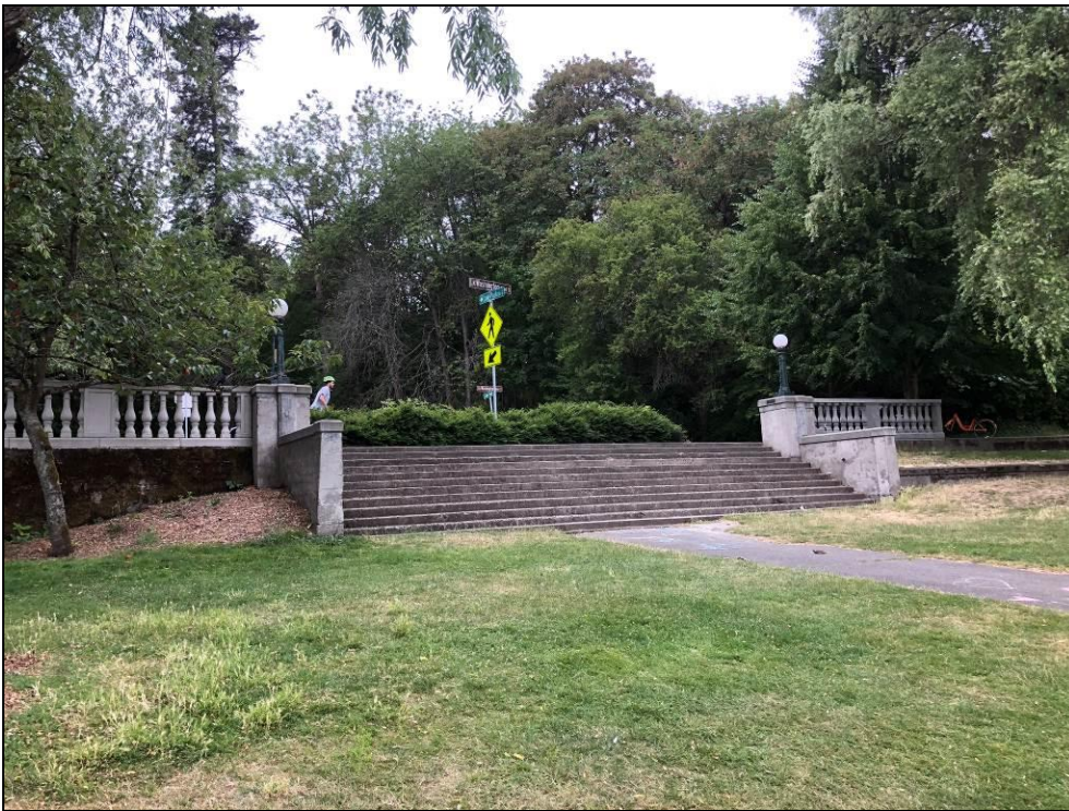
Figure 24, looking northwest from the Mt. Baker Beach area toward the entry steps, and concrete retaining walls with decorative balustrades, July 18, 2018.
