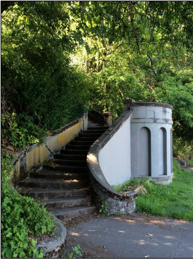
Figure 20, lower landing, Dose Terrace Stairs, June 15, 2018.
