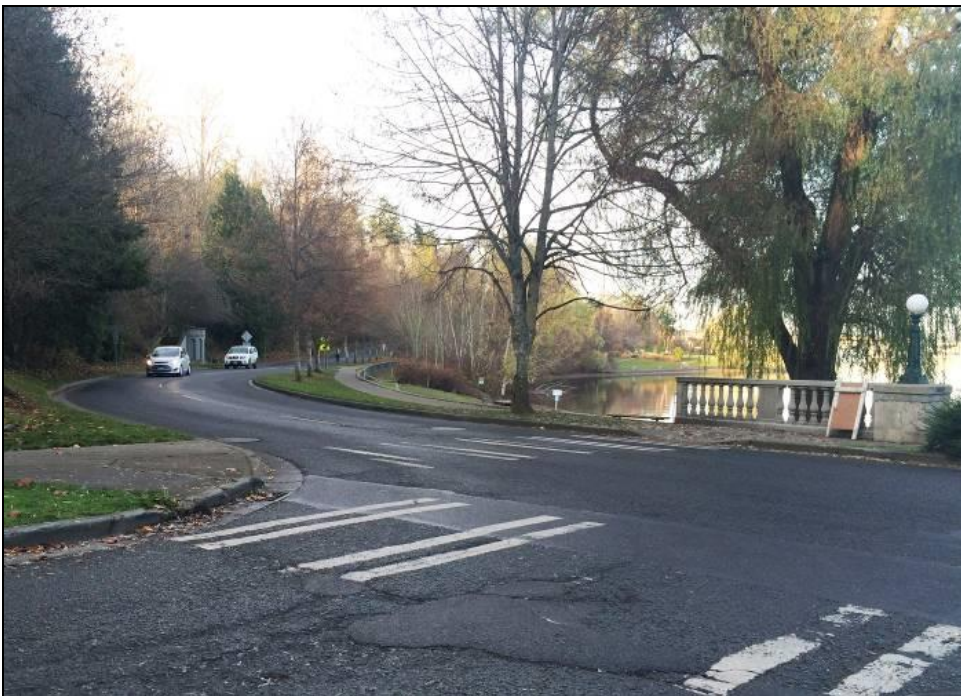
Figure 21, looking north from the intersection of Lake Washington Boulevard S and Lake Park Drive S with a portion of the balustrade wall of the Mount Baker Beach area, November 20, 2017.
