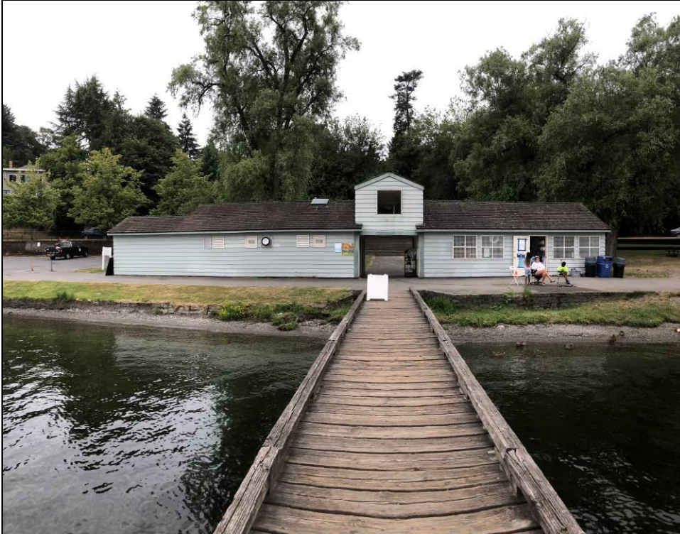
Figure 23, looking southeast from the pier at the Mount Baker Bathhouse, July 18, 2018.
