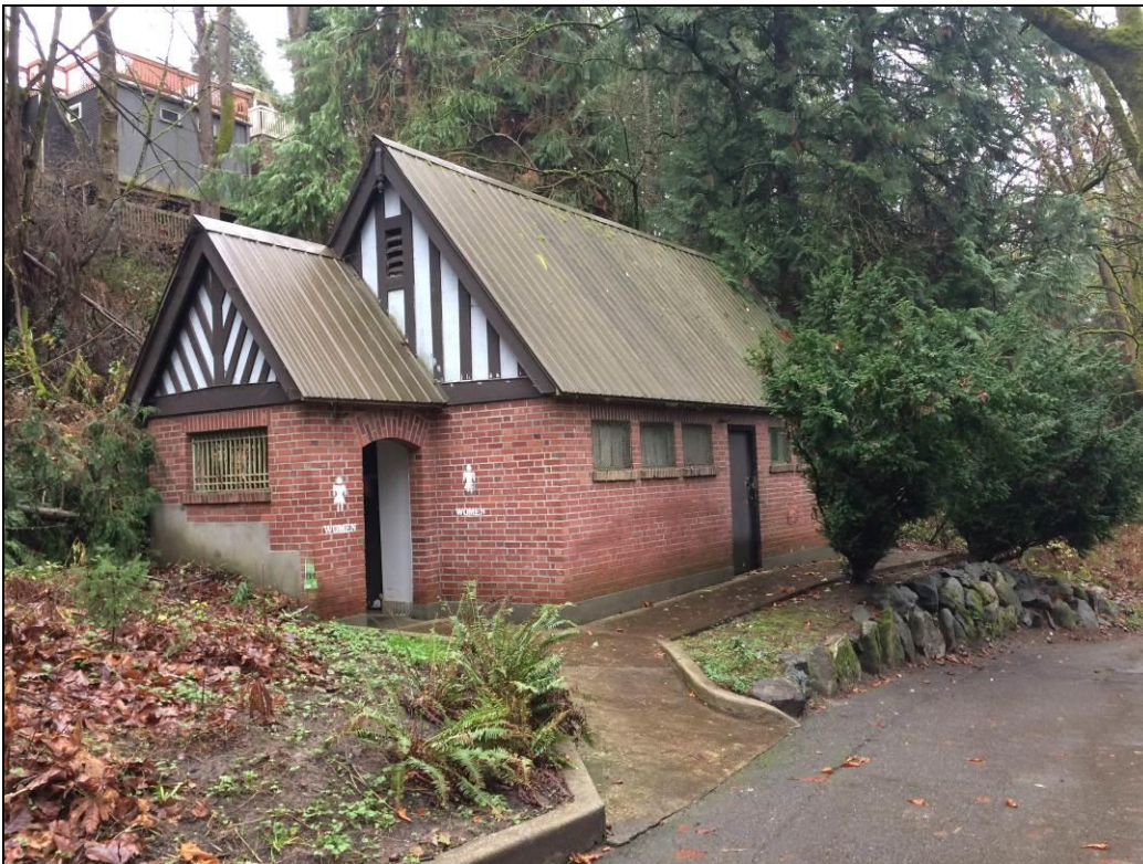
Figure 11, looking southwest at the 1928 Comfort Station, south and east facades, December 18, 2017.
