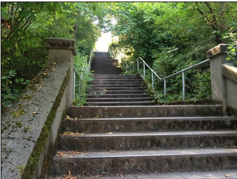
Figure 19, looking east at the Dose Terrace Stairs, June 15, 2018.
