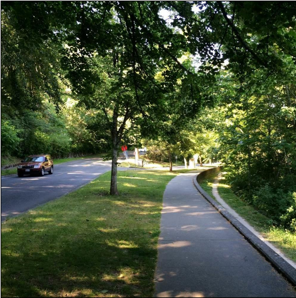
Figure 18, looking north along the sidewalk and retaining wall in Mount Baker Beach area toward the gate and entry drive to the Colman Park shoreline area, June 15, 2018.
