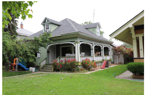
Figure 15. Hip Roof Example. 509 North Naches Avenue (ca. 1912), front southwest corner.
