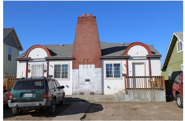
Figure 11. Stucco Example. 604 South Naches Avenue (ca. 1920), front east facade.
