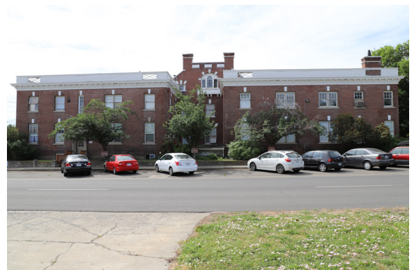
Figure 16. Flat with Parapet Roof Example. 115 North Naches (ca. 1930), side north facade.
