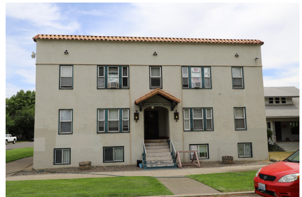
Figure 9. Low-rise Apartment Block Form Example. 415 North Naches Avenue (ca. 1925), front west facade.
