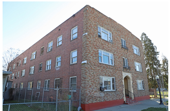
Figure 12. Brick Example. 211 South Naches Avenue (ca. 1930), front northwest corner.
