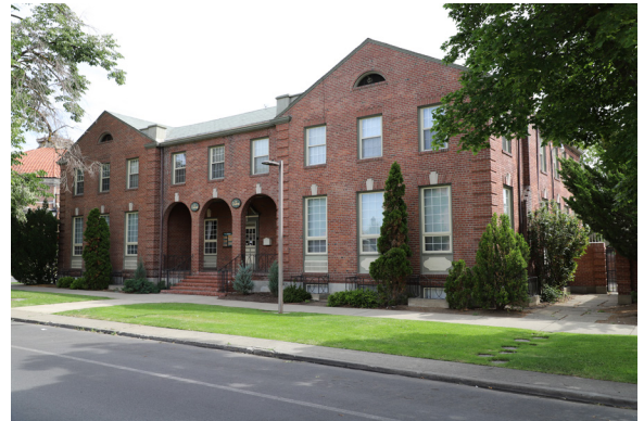
Figure 8. Facade Break Example. 15 North Naches Avenue (ca. 1934), front west facade showing the middle facade portion recess.
