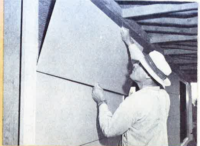
Special pre-cut siding widths are available for wide lapped siding, other uses.
