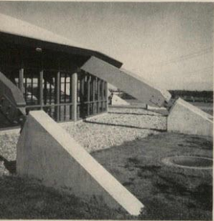
The exuberant shapes of the gymnasium and cafeteria add an air of individuality to this economical, court-yarded school. The separation of these noisier areas from the main block reduces the sound level and abets the possibility of their use for community activities
