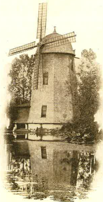
An Old Dutch Mill in the State of Washington—Covered with Red Cedar Shingles
