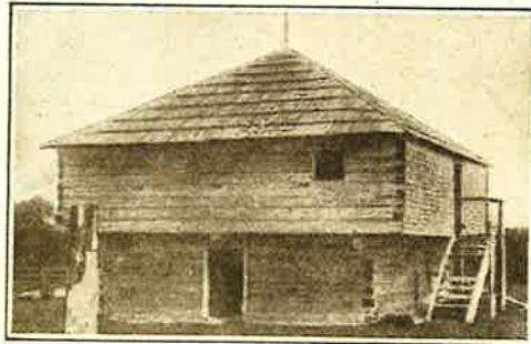
The old Fort Borst Block House here shown was built in 1845, and the split shingles on the roof are as sound today as the day they were put on
