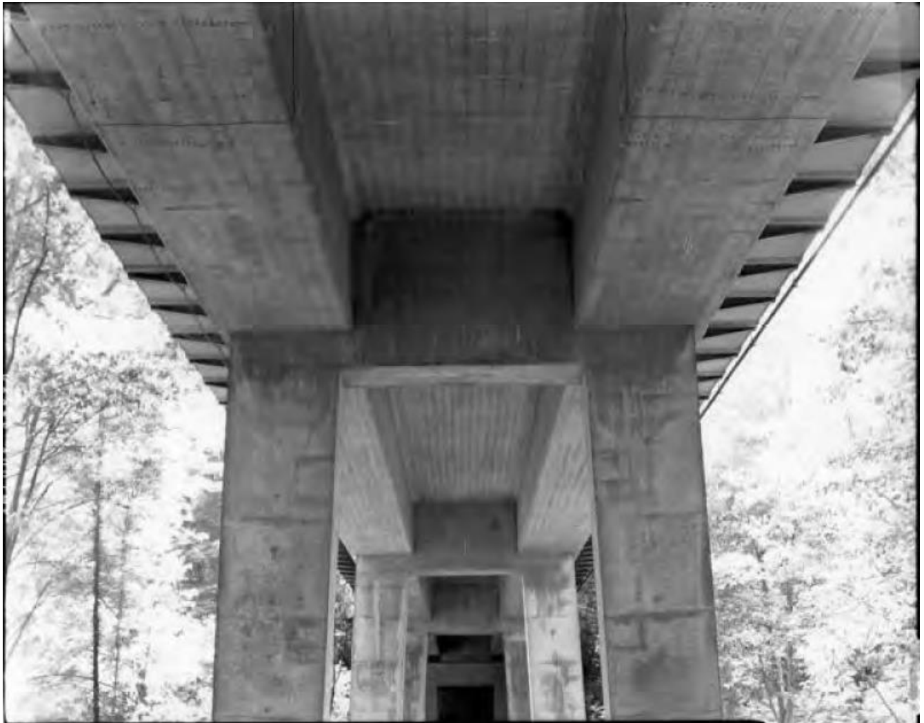
Figure 6. View of piers and hollow box girders, 15 th Avenue Bridge (1949), Seattle, King County, Washington. Photograph found in Mishkar, et. al. 2009. Box girders consist of twin separate rectangular cells.
