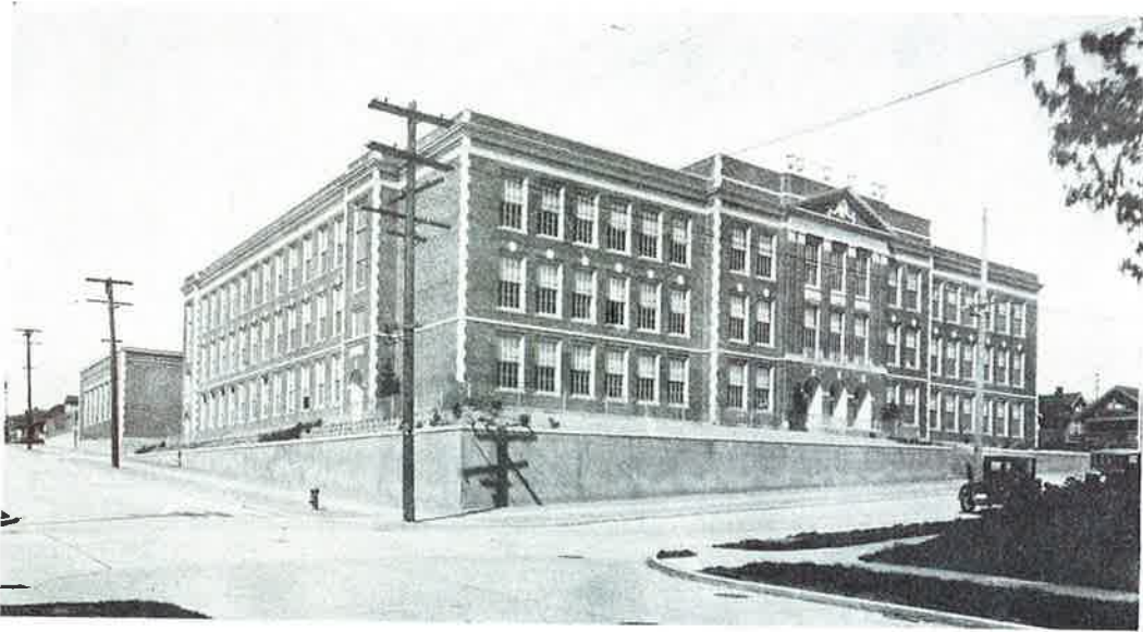
Alexander Hamilton Junior High School, Seattle. This Building was Designed by P. A. Naramore, Architect.
