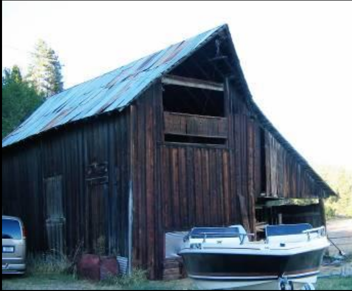
Carlstrom Barn – c.1910
