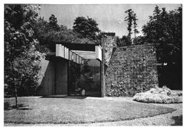
CONCRETE WALL at right is 5½ inches thick, has interesting surface texture with rocks hand-placed when slab was formed. It was poured at the site—tilted upward to vertical position; surface inside house similar.
