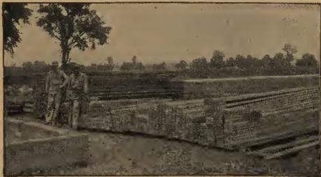
1 All framing lumber cut to exact length and shape, ready to be nailed in place. No time lost in measuring, cutting and fitting.
