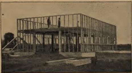
2 74 Hours' carpenter labor shows the framing of barn rapidly nearing completion.
