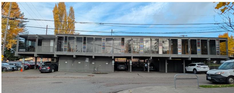
[Figure 15] Seattle, WA. Kirk, Wallace McKinley, AIA, and Associates Office (2024).
