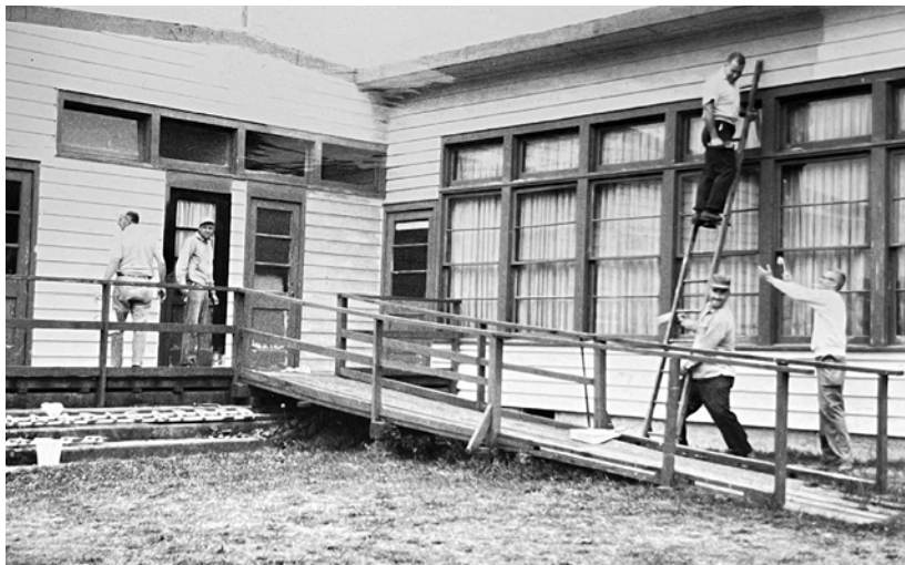
[Figure 12] Seattle, Wa. Renovation of Seattle Handicapped Center's first building, including the construction of a ramp (June 1968). Ida Daly and other leaders with disabilities led the project and vision for the site.
