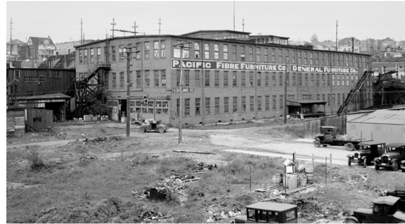
[Figure 3] Seattle, WA. Goodwill Industries building (1931).
