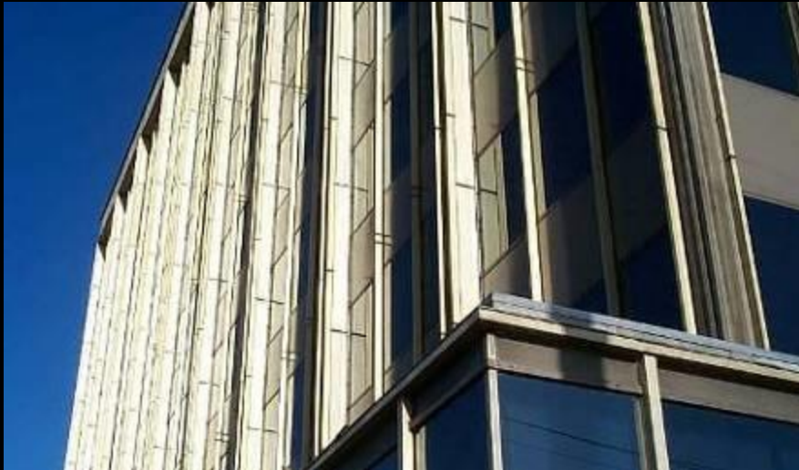
Capitol Center Building Bennett & Olson, Olympia 1966
