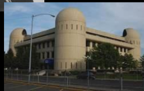
Spokane Co. Social & Health Services Bldg. Built: 1977
