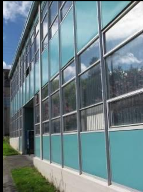
1007 Washington Building Olympia, 1959
