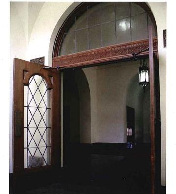
West Vestibule: This is the main entry vestibule. It contains three risers with a terrazzo floor and inset mat. The base is black marble. The walls are plaster with textured paint they contain a cast bronze tablet and grills. The ceiling, at almost 13', is vaulted plaster. The exterior doors are square paneled mahogany with four leaded glass lights. The interior doors are mahogany with a single arched top light with leaded glass. Both doors have steel half round transoms above.
