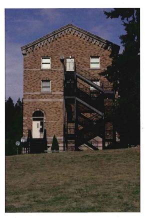
The South fire escape added in 1979, is not compatible with the historic character of the building and should be removed. It is, however, currently serving as the second means of egress for two residences on the Second and Third Floors. It must be maintained until interior egress systems are reworked to provide an alternative second means of egress. It may be possible to remove it sooner if the residences are unoccupied – this decision would be at the discretion of the Building Official.
