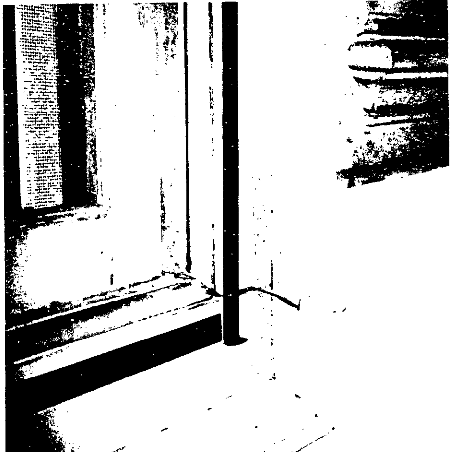
Figure 7(a) In cases where there were no stools and also where a split unit was used to facilitate self-storage, small "shelves" were made in the vertical steel strips to deter creeping. Photograph shows a 90 degree angle at the bottom of the vertical steel strip in a situation where there was no stool. Photo: Tom H. Taylor. (b) The adjacent drawing shows the two "shelves" used with split units as well as a top safety catch formed at the end of the steel strip. Drawing: Christina Henry.
