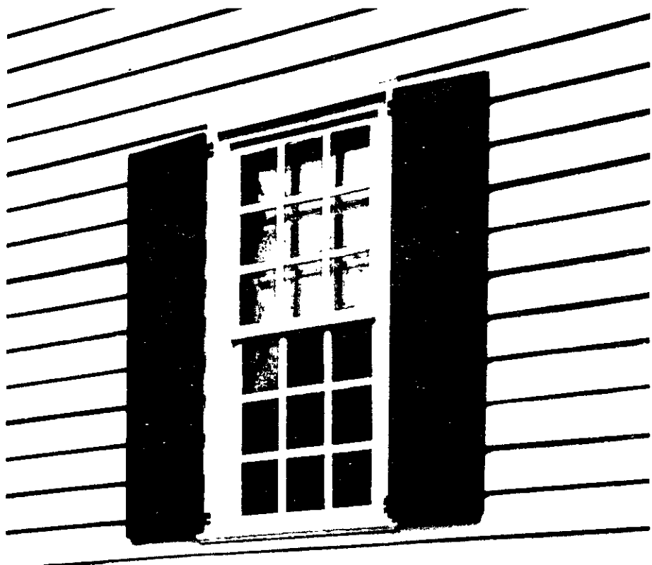
Figure 8. The unobtrusive interior storm window required no physical damage or exterior visual alteration to the original window. Photo: Tom H. Taylor.
