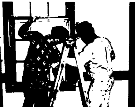
Figure 5. The meeting bar of the split storm unit was located adjacent to the historic meeting rail in windows where the upper and lower sash were the same size. Photograph shows the installers checking to make sure the lower unit will properly align. Photo: Tom H. Taylor.
