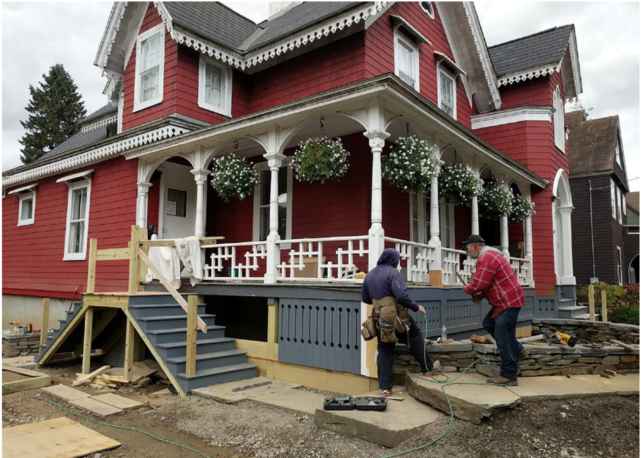
The low elevation mitigation of this dwelling in Owego, New York of four-feet included adding slatted wood panels under the porch, new hand rails and stairs.
