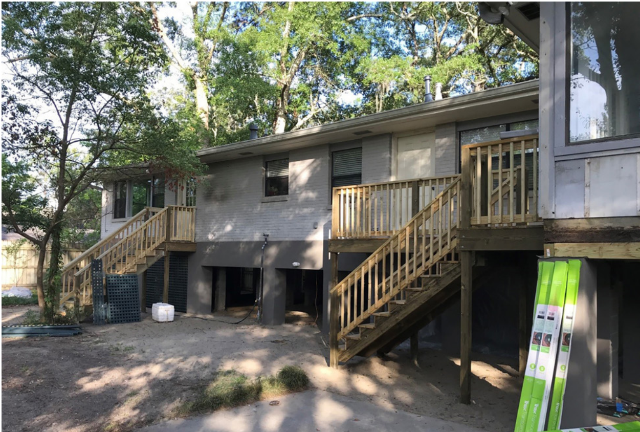
This ca. 1963 Ranch style dwelling in Mandeville, Louisiana required raising its concrete slab along with the rest of the house to meet the Base Flood Elevation of four feet.
