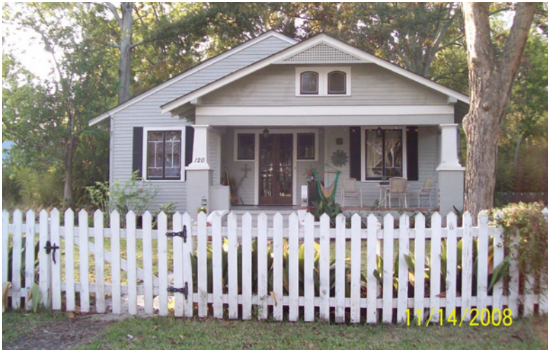
Example of a high elevation project in Mandeville, Louisiana. This Bungalow dwelling was built on a brick foundation.
