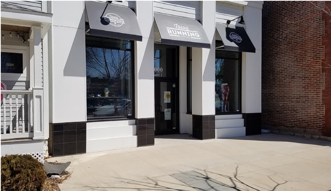
Example of infill construction that is flood proofed. In the event of a flood, a flood gate will be installed across the door opening.
