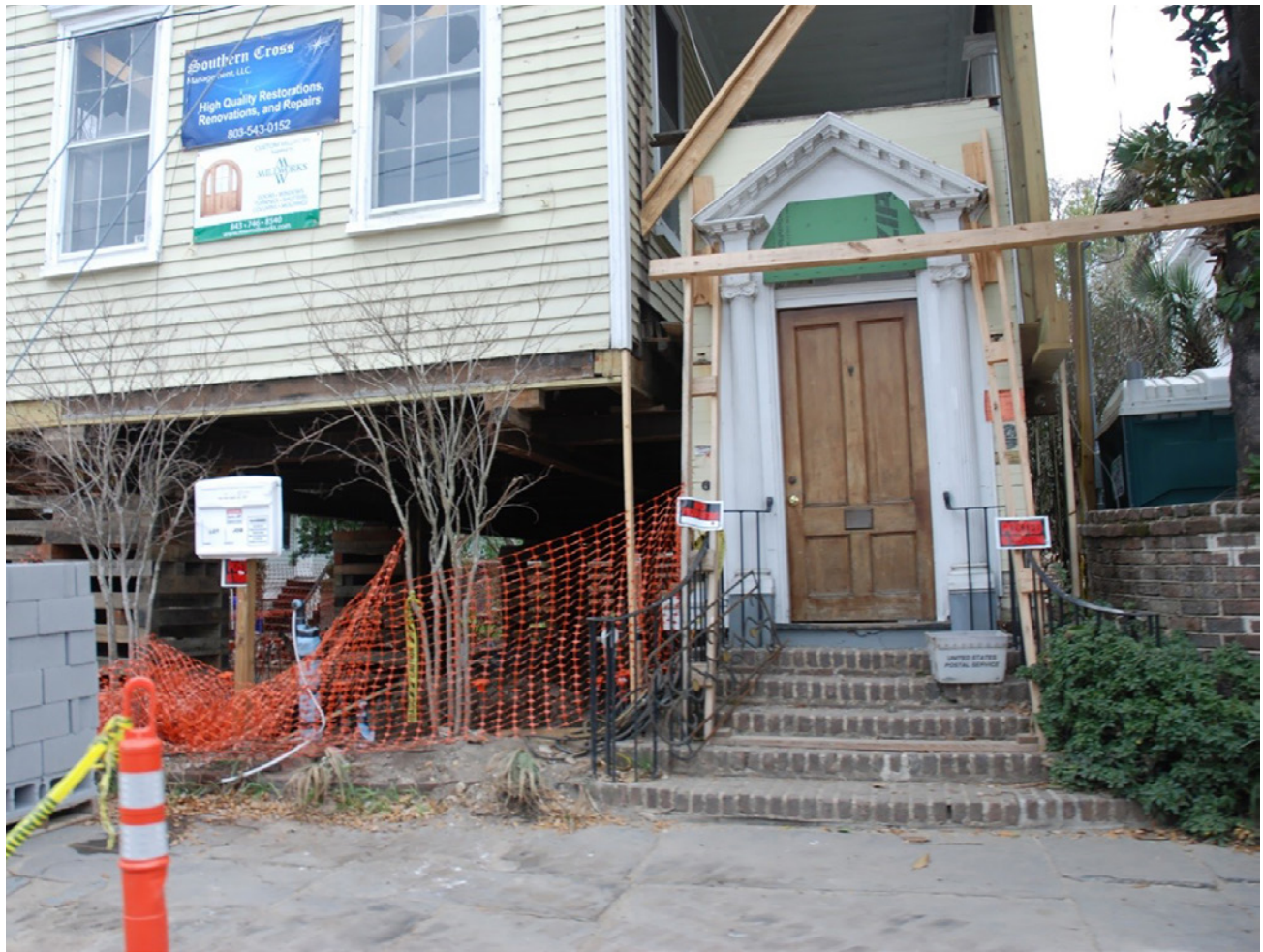
A Category 2 dwelling in the process of an elevation meeting the Guidelines.
