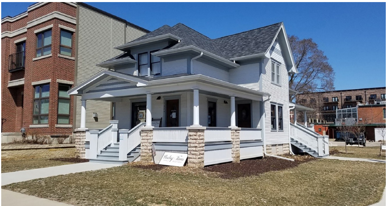
A relocated single family home that now has commercial on the elevated main floor and residential above. This house was moved one lot to the southeast to create a larger, contiguous site for new development and elevated approximately two feet
