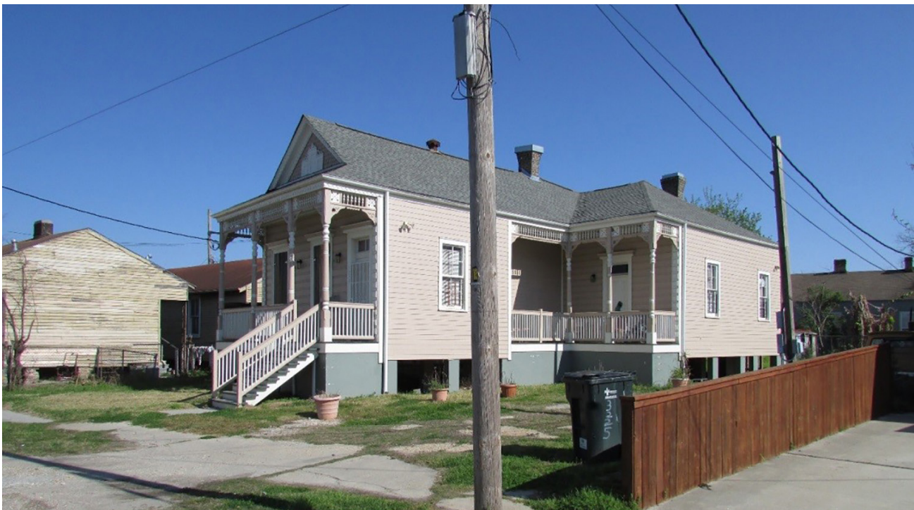
The same dwelling after being elevated 3.5 feet on both a solid and open pier concrete foundation. New stairs and a safety railing to match the original railing were added. This was a project completed for Rebuild Together New Orleans.
