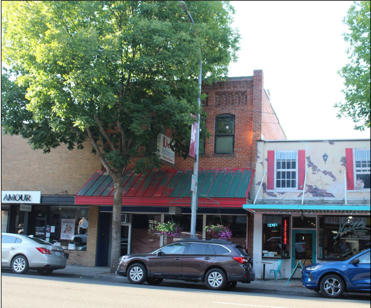
Figure 25: 226 E. Main Street today (2023) Photo by Diana Painter
