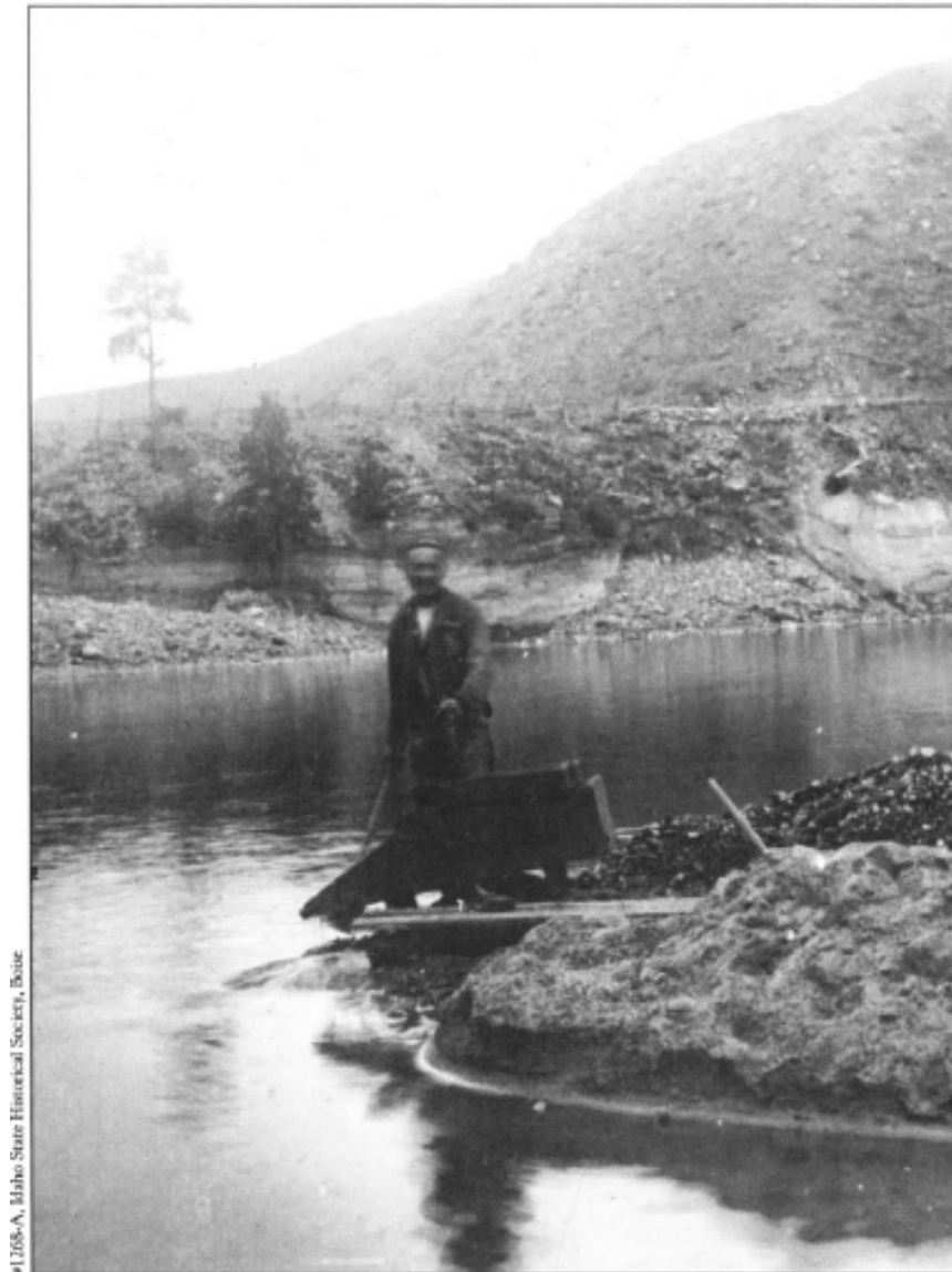
Figure 4: Chinese miner near Freedom, Idaho with rocker for placer mining Source: “Outsiders in the ‘Land of the Free’”
