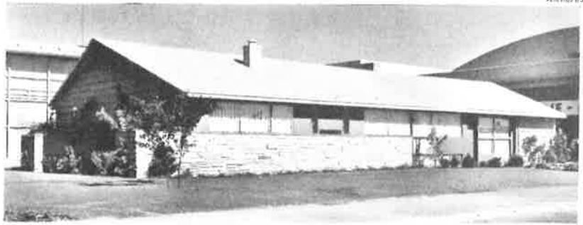
Seattle, Wash., Houses by builder Albert La Pierre were designed by W. A. Wallander
