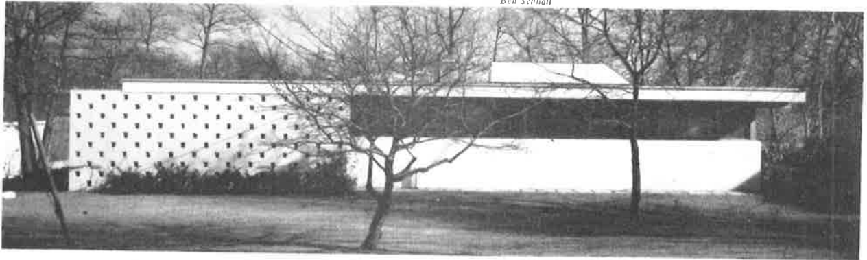
Tuck House, Scarsdale, N. Y. Marcel Breuer, architect. Horizontality achieved with strong fascia, even sill line
