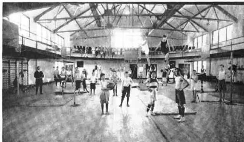
Boys' Gymnasium, Deerfield-Shields Township High School Joseph C. Llewellyn Co., Architects
