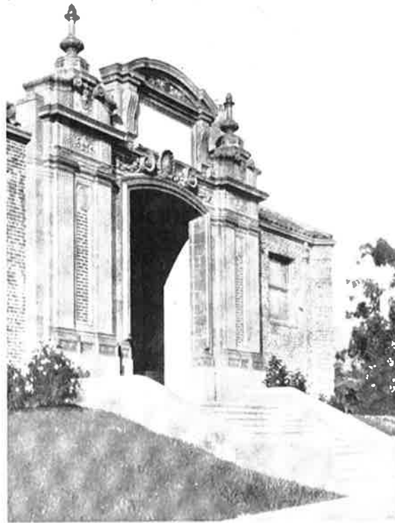
Detail of Entrance
