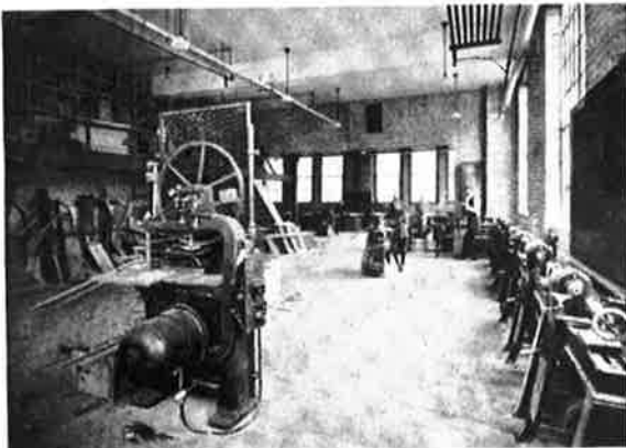
Woodworking Machinery Room Deerfield-Shields Township High School
