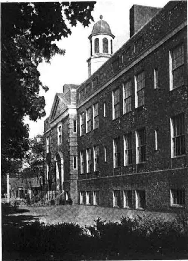
VIEW OF ENTRANCE FRONT
