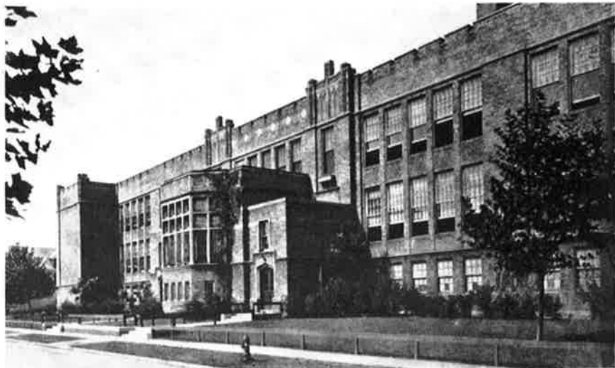
Entrance Front of Empire School, Cleveland
