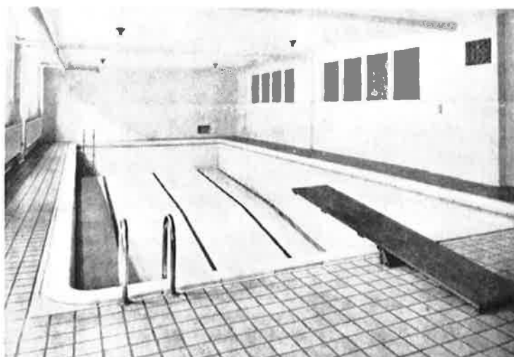
Swimming Pool, Hixon Annex, High School, La Crosse, Wis. Note drain in floor to tile overflow of pool Joseph C. Llewellyn Co., Architects
