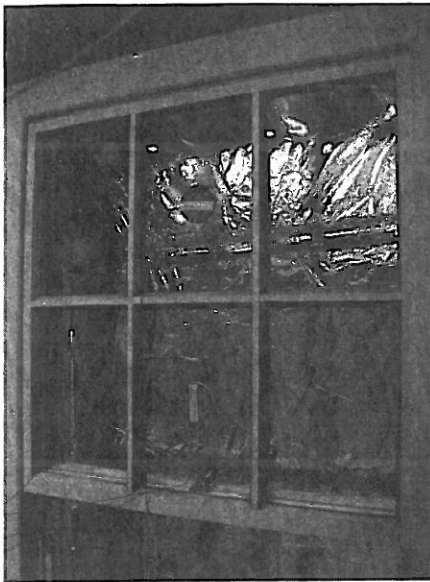
Fig. 9. Low-e foil on the side of the roller blind facing the Historic Scotland window.
