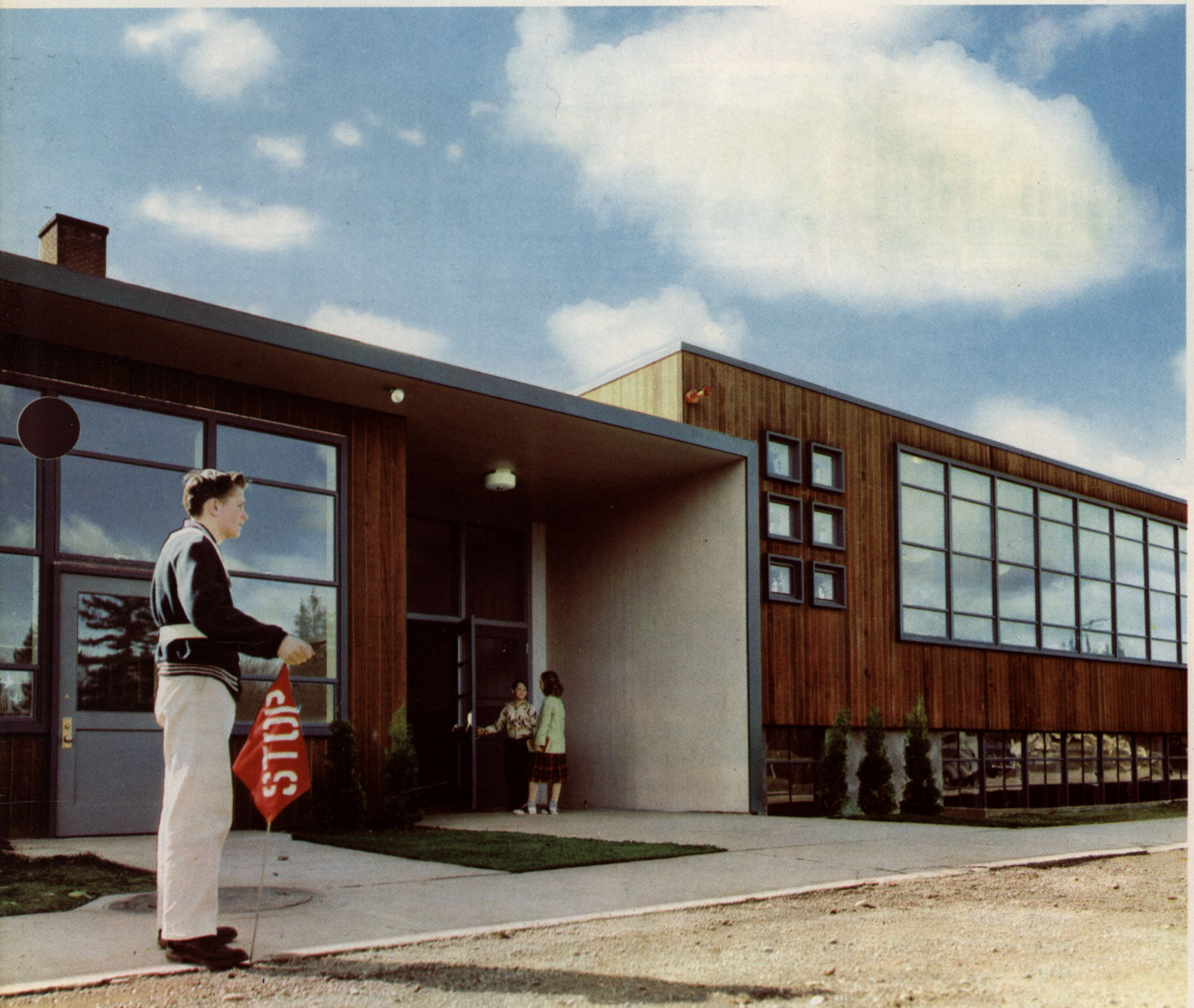
Wilkes School, Portland, Oregon • L. E. McCoy, Architect
