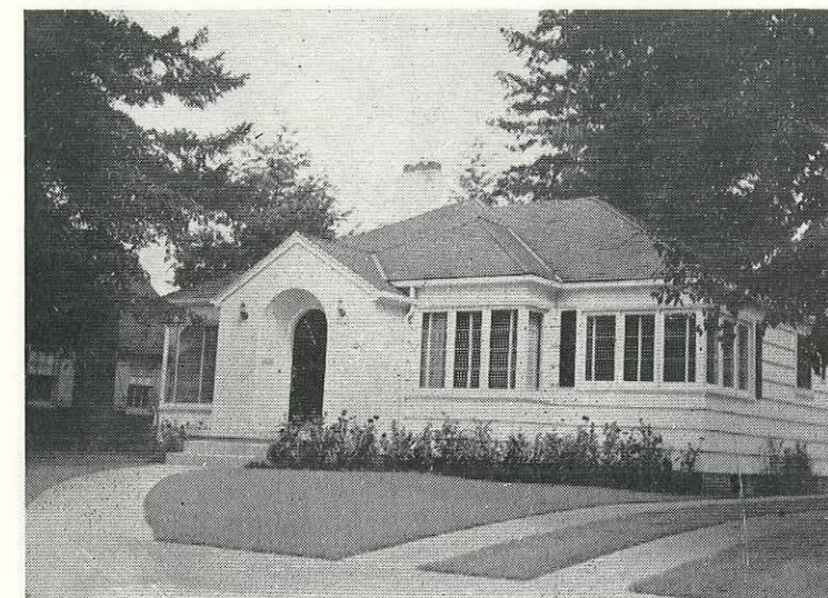
PLAN No. 5039 Size 37'-6" x 30'-0" — Area 1128 sq. ft. A tremendous amount of light is furnished by the larger corner windows in this house which has a partitioned full basement.
