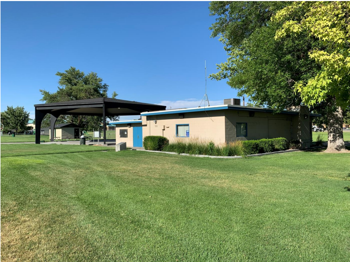
WA_FranklinCo_KurtzmanPark_0001. Looking northeast to the Kurtzman Park Youth Center from the intersection of Wehe Ave. and Alton St.
