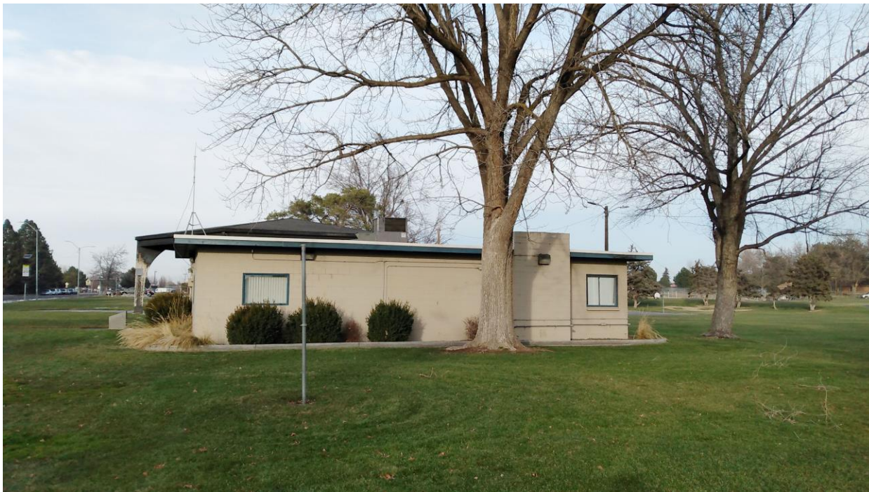
WA_FranklinCo_KurtzmanPark_0006. Looking north to the south (rear) wall of the youth center.
