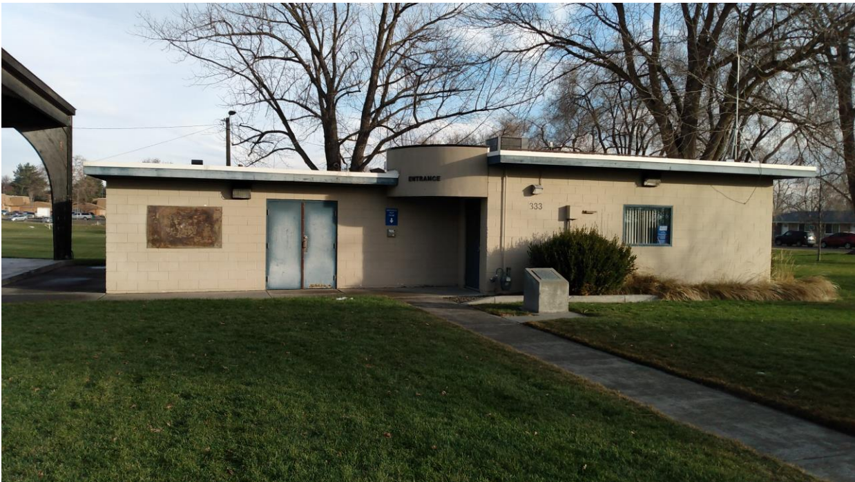
WA_FranklinCo_KurtzmanPark_0003. Looking east to the west (side) wall of the youth center. Original volume to right, addition to left.
