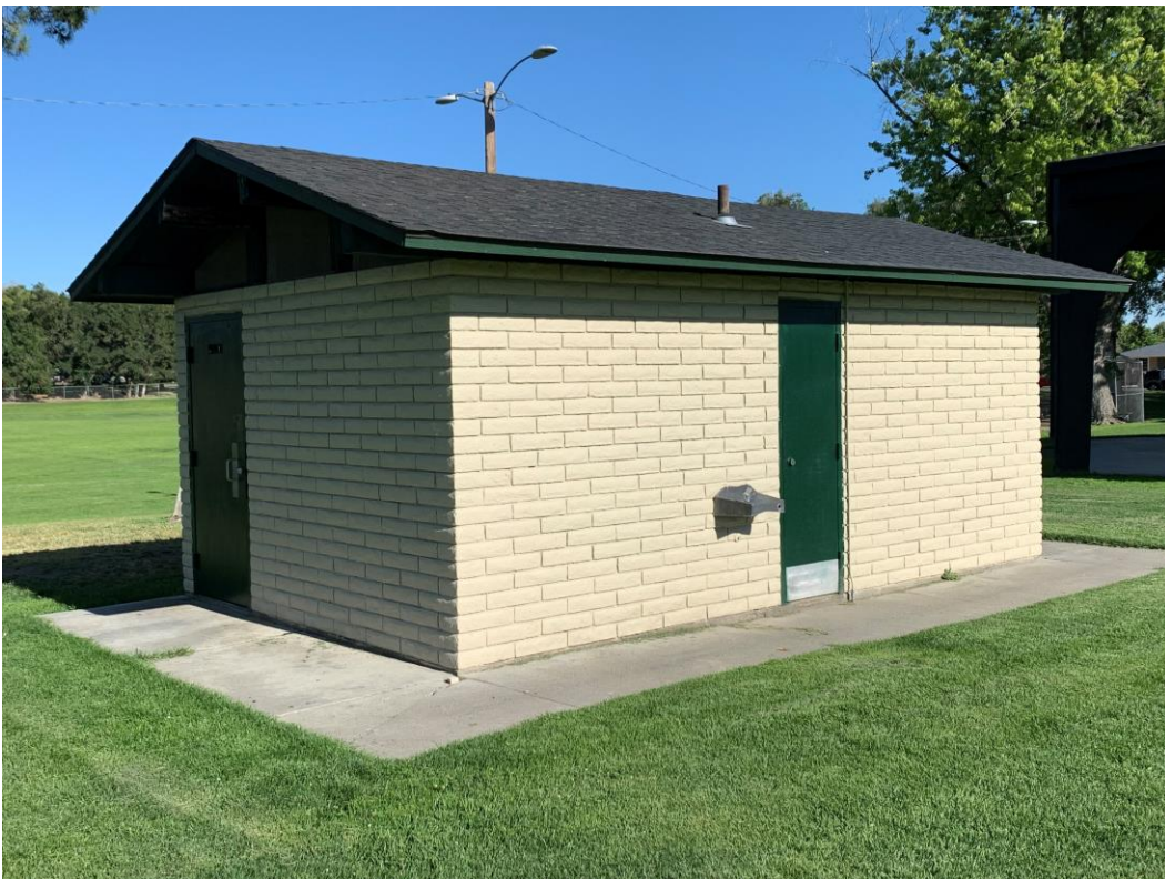
WA_FranklinCo_KurtzmanPark_0009. Kurtzman Park Comfort Station.
