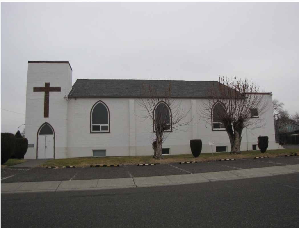
WA_Franklin_MorningStarBaptistChurch_0003. Looking north to the south (side) wall of the church.
