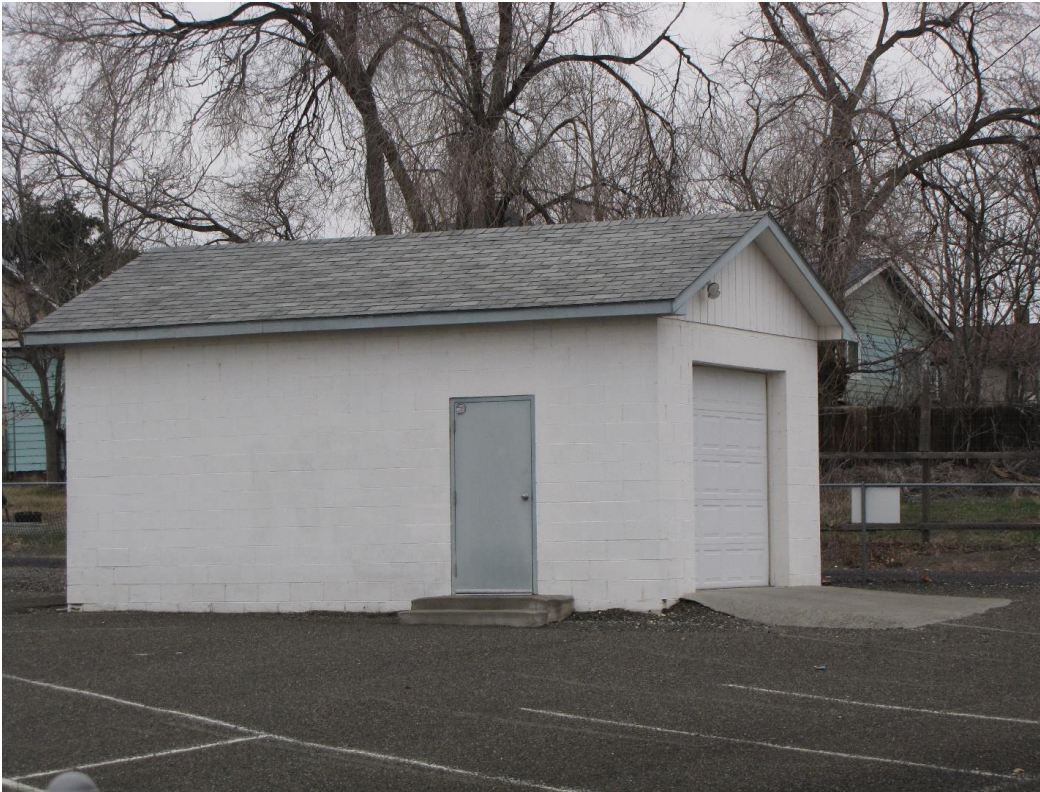
WA_Franklin_MorningStarBaptistChurch_0014. Looking east-northeast to the west (side) and south (front) walls of the garage.
