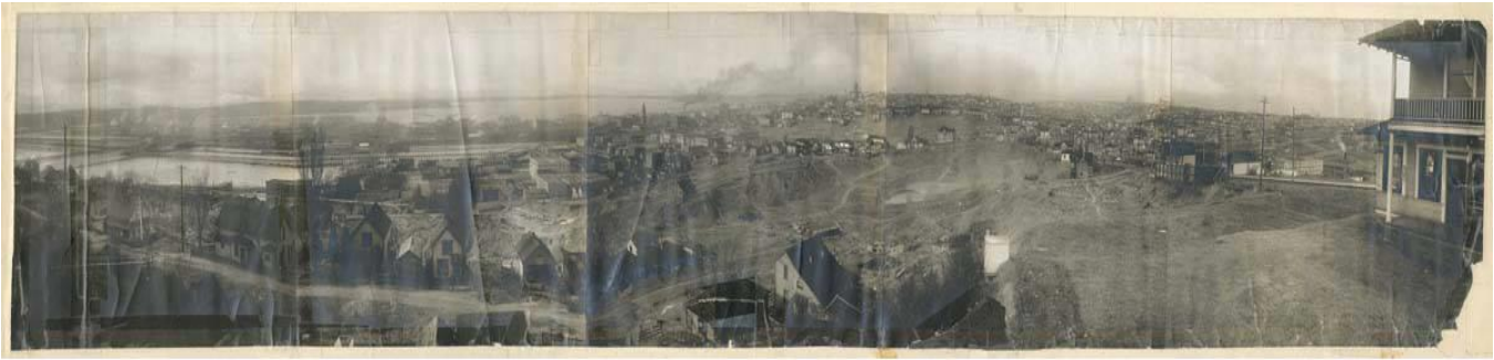
View of Jackson Street regrade (of north Beacon Hill), 1910. Future location of Dr. José Rizal Park is at lower center of photograph. Courtesy Museum of History and Industry.
