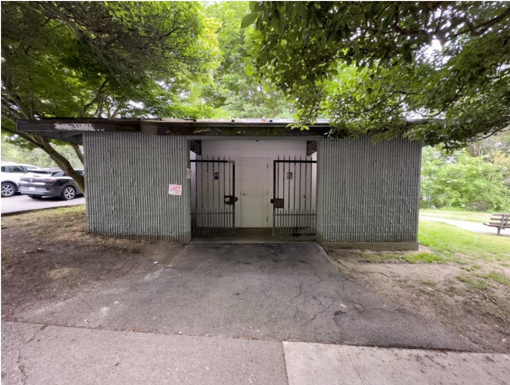
WA_King County_Dr. Jose Rizal Park_0017. Restroom looking west.
