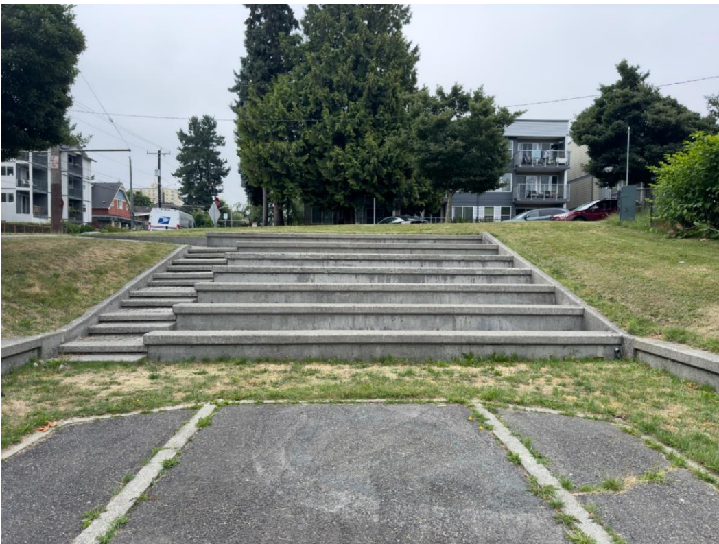
WA_King County_Dr. Jose Rizal Park_0004. Amphitheater looking south.
