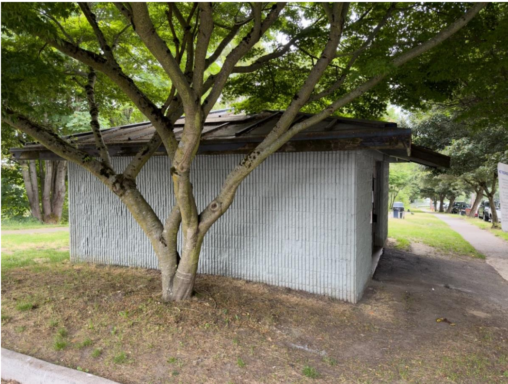
WA_King County_Dr. Jose Rizal Park_0018. Restroom looking north.
