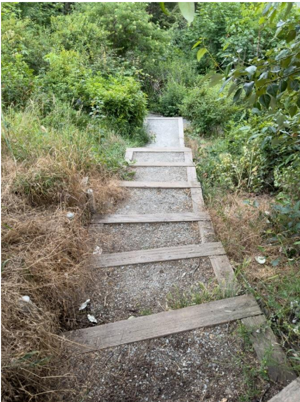
WA_King County_Dr. Jose Rizal Park_0022. Stairway detail looking southwest.
