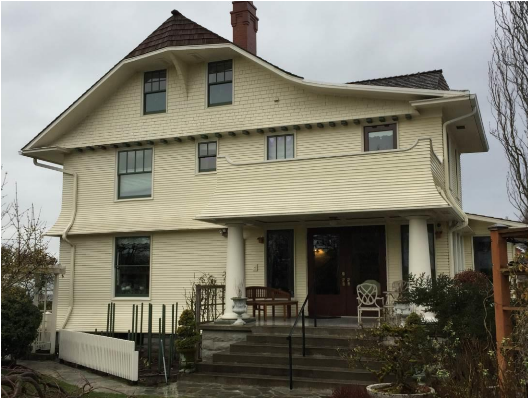
4 of 11. South facade
