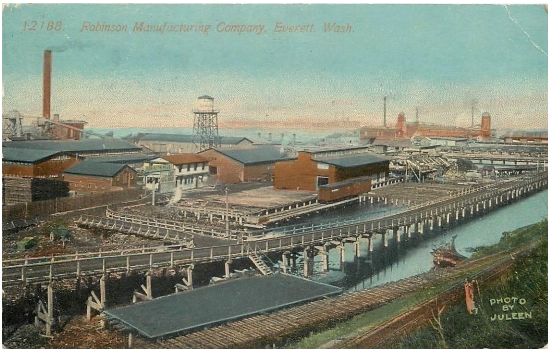
Robinson Manufacturing Co. Plant – Everett – c. 1915
