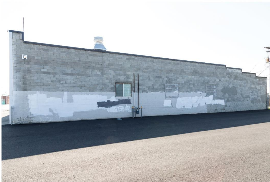
WA_Yakima County_Yakima Valley Filipino Community Hall_0006. West facade.
