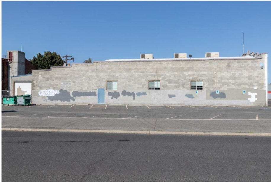
WA_Yakima County_Yakima Valley Filipino Community Hall_0003. Side east facade.
