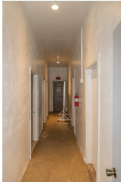
WA_Yakima County_Yakima Valley Filipino Community Hall_0017. Hallway, east of the stage, looking south.
