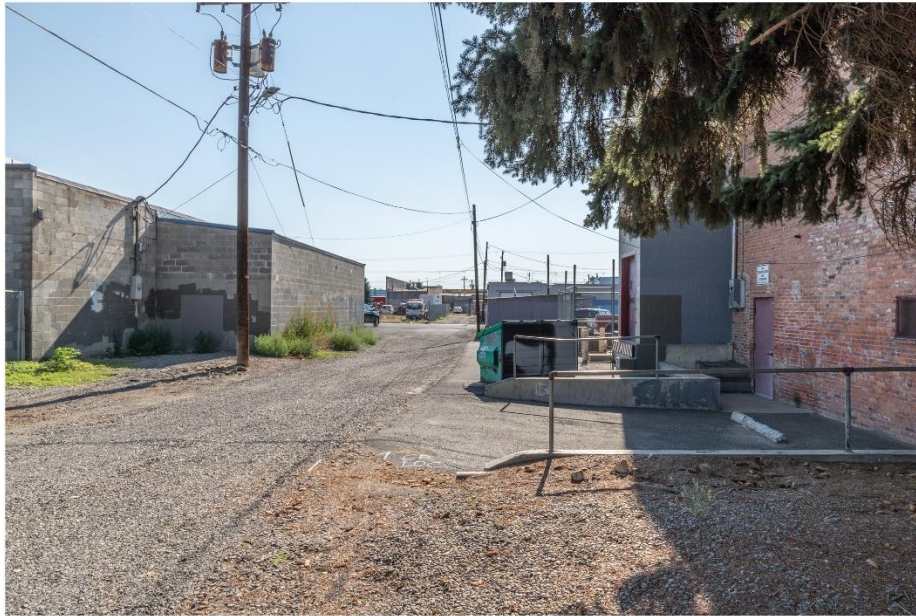
WA_Yakima County_Yakima Valley Filipino Community Hall_0011. Looking east along the alley.
