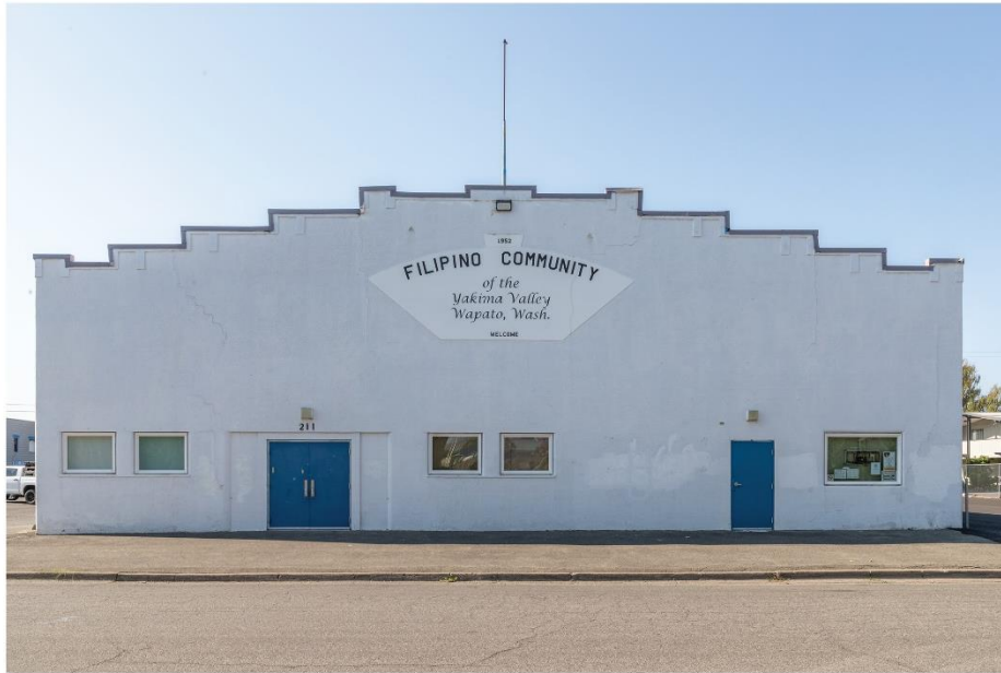
WA_Yakima County_Yakima Valley Filipino Community Hall_0001. Front north facade fronting W Second Street.
