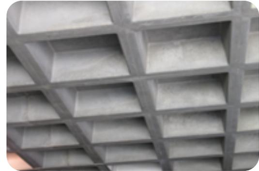
features include the use of waffle slabs for floor and roof systems. As the name implies this cast-in-place building system utilized continuous pour of concrete with a coffered underside to reduce the weight of the slab. Such slabs were often left exposed.
