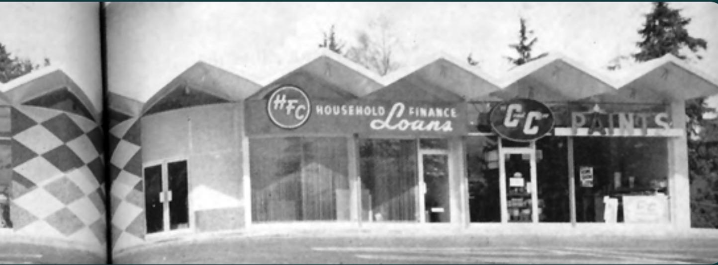
The choice of a thin shelled concrete roof for this building reduced the total construction costs by 25 cents a square foot compared with wood or steel. The shell is only 2-1/2 to 3-inches thick. Forms were moved along the length of the building to create the shape. Jentoft and Forms, builders, Welton Becket and Associates, architect and engineers. Source: *American Builder Magazine*, January 1958.
