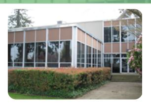
with colored ceramic. The Pittsburg Plate Glass Company manufactured the glass panels under the trade name "Spandrelite." The Libbey-Owens-Ford Corporation sold sixteen colors options under the "Vitrolux" brand. Later, spandrels were available in other materials such as composite metal panels containing lightweight insulation cores, precast concrete panels, during the 1950s and 1960s was Fentron Industries.
