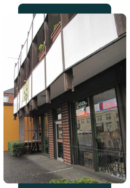
(left): Masonite catalog cover from 1935; (above): Fiberboard panels on a commercial building, Auburn (c. 1970).
