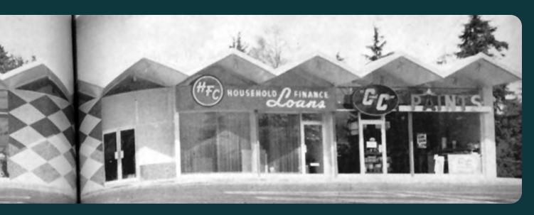
The choice of a thin shelled concrete roof for this building reduced the total construction costs by 25 cents a square foot compared with wood or steel. The shell is only 2-1/2 to 3-inches thick. Forms were moved along the length of the building to create the shape. Jentoft and Forms, builders, Welton Becket and Associates, architect and engineers. Source: American Builder Magazine, January 1958.
