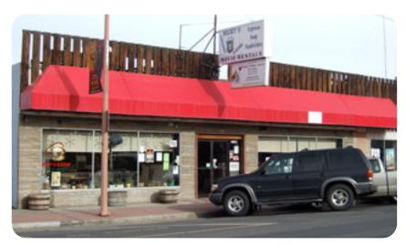
(upper): Concrete simulated stone veneer. This was installed in a bed of mortar similar to tile; (lower): Simulated stone storefront, Prosser. Image courtesy DAHP.
