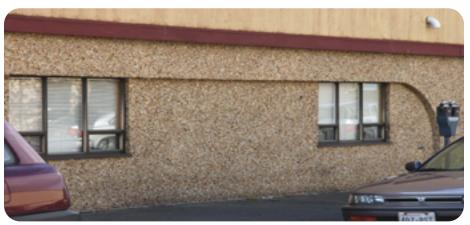
(left): Detail of pebbledash on wire lath backing; (upper right): Pebbledash panel within a curtain wall; (lower right): Pebbledash as full building cladding. Images courtesy DAHP.
