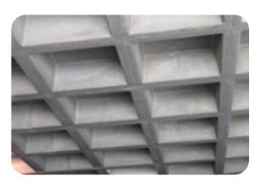
features include the use of waffle slabs for floor and roof systems. As the name implies this cast-in-place building system utilized continuous pour of concrete with a coffered underside to reduce the weight of the slab. Such slabs were often left exposed.
