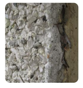
material poured into a mold and then the finish aggregate applied to the surface. In both cases, floats are then used to tamp the aggregate, seating the stones firmly in the cementitious layer and pressing them to the desired finish depth. A sealer or glaze is then applied to seal the masonry and highlight the aggregate color.
