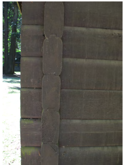
CORNER DETAIL OF A TYPICAL PAN-ABODE STRUCTURE SHOWING THE TONGUE-AND-GROOVE CONNECTION AND LAPPED CORNERS. SOURCE: ARTIFACTS CONSULTING, INC.
