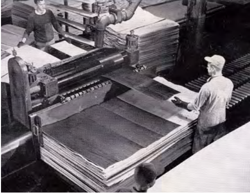
CA. 1950 GLUE APPLIED TO CROSS-BANDING VENEER. SOURCE: COUR, ROBERT M. (1955). PLYWOOD AGE. BINFORDS AND MORT: PORTLAND.
