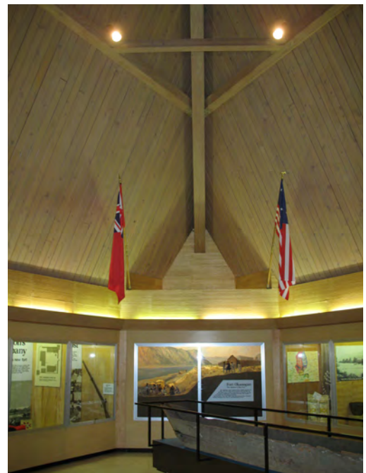
INTERIOR VIEW OF THE FORT OKANOGAN INTERPRETIVE CENTER'S UPPER PYRAMIDAL ROOF PORTION. NOTE THE LIGHT, PIGMENTED STAIN EMPLOYED ON THE INTERIOR WOOD SURFACES. ORIGINAL DISPLAY CASES LINE THE WALLS BELOW. SOURCE: ARTIFACTS CONSULTING, INC.
