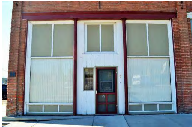
Main facade east storefront, 2021. View to south.
