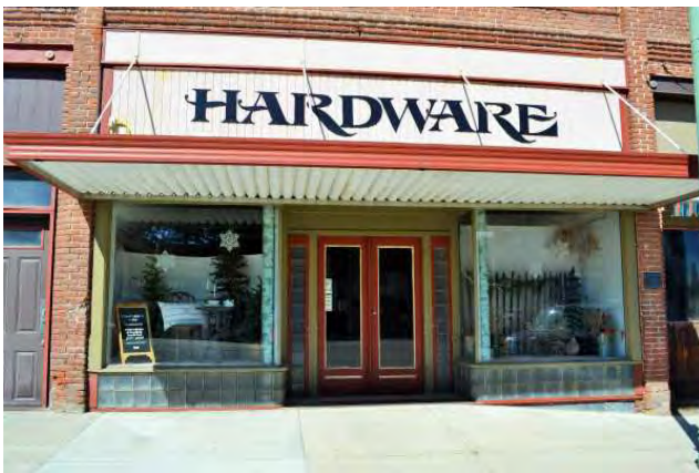
East storefront, 2021. View to NE.
