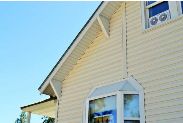
Covered knee braces in north gable, 2021. To SE.
