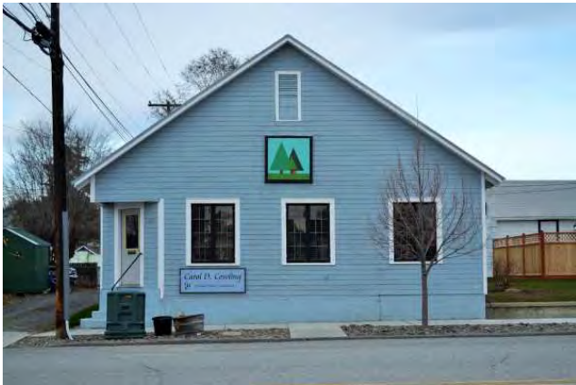
East (front) elevation, 2021. View to west.
