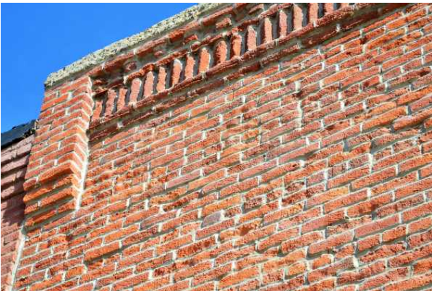
Brickwork at SW corner main facade, 2021. View to NW.
