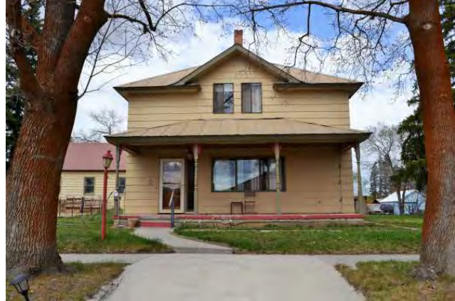
South (front) elevation, 2021. View to north.
