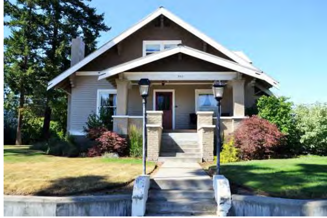
South (front) elevation, 2021. View to north.
