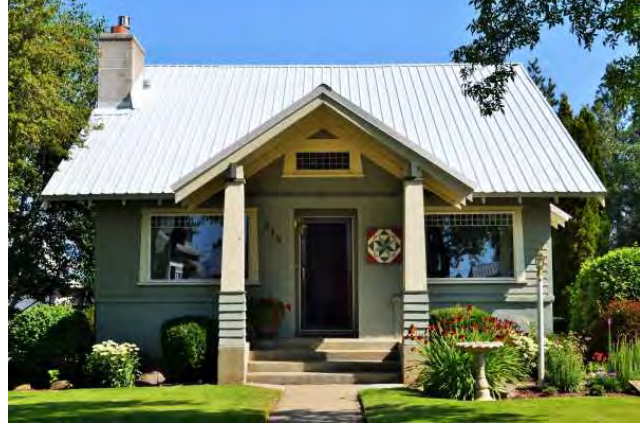
South (front) elevation, 2021. View to north.
