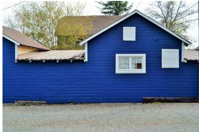
North (rear) of second cabin from west, 2021. To south.
