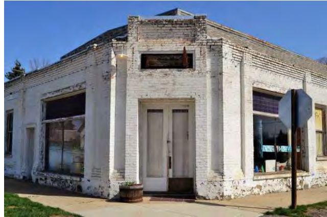
Main (SW corner) entrance, 2021. View to NE.
