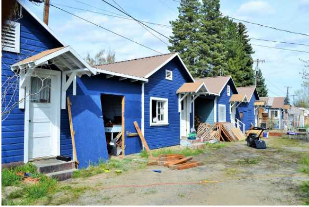
South (front) and west sides, 2021. View to NE.
