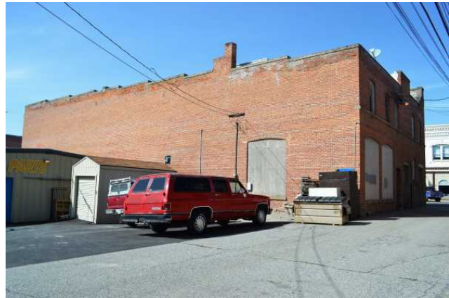
South and east sides, 2021. View to NW.
