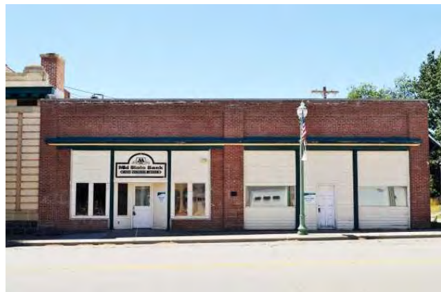
Annex, east (front) side, 2021. View to west.
