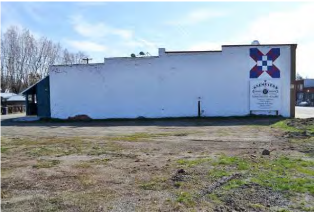
West elevation, 2021. View to east.
