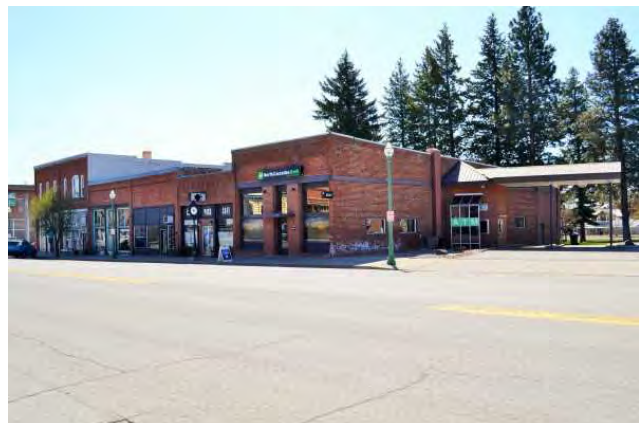
Overview from Locust St., 2021. View to SE.
