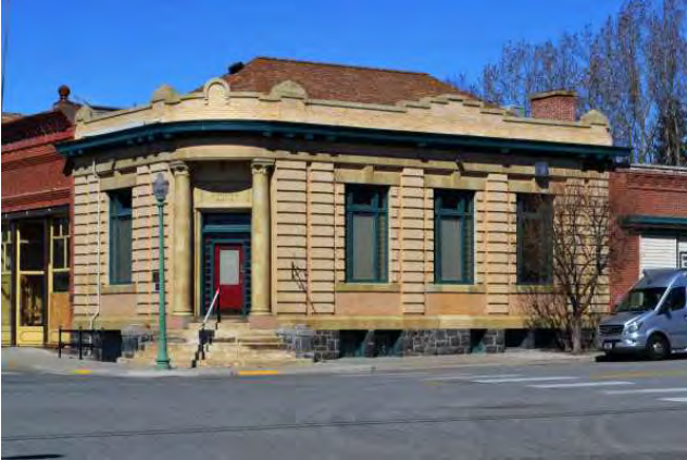
South and east sides, 2021. View to NW.
