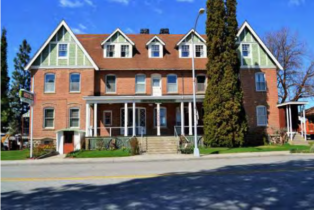
East (front) elevation, 2021. View to west.
