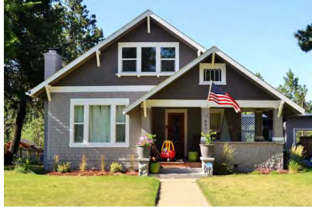
South (front) elevation, 2021. View to north.
