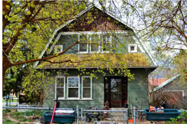
South elevation, 2021. View to north.
