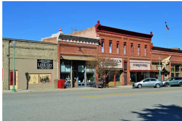
Overview from Locust St., 2021. View to NE.
