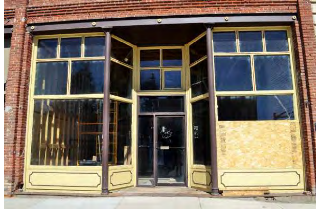
East storefront, 2021. View to north.
