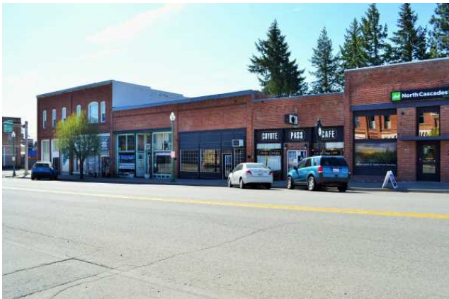
Overview from Locust St., 2021. View to SE.
