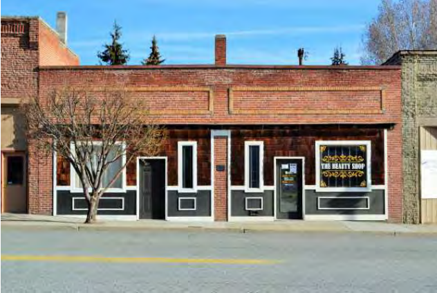
South (front) elevation, 2021. View to north.
