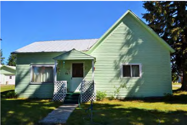
South (front) elevation, 2021. View to north.
