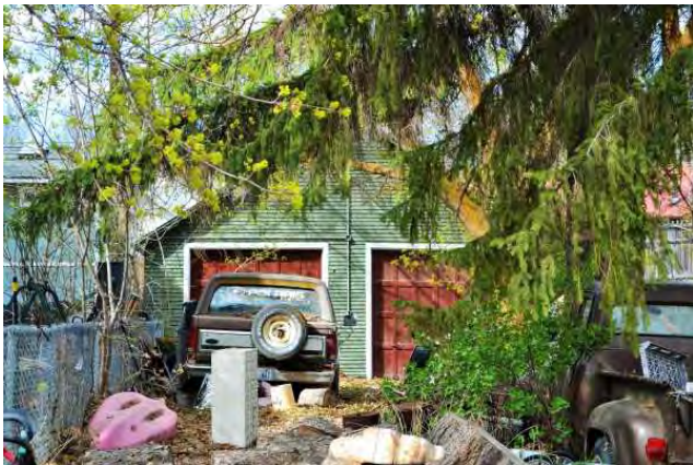
Garage, south (front) side, 2021. View to north.
