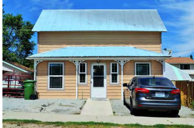
South (front) elevation, 2021. View to north.
