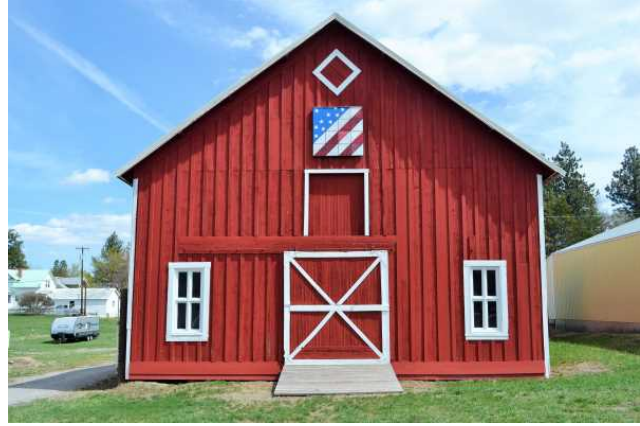
West (front) elevation, 2021. View to east.
