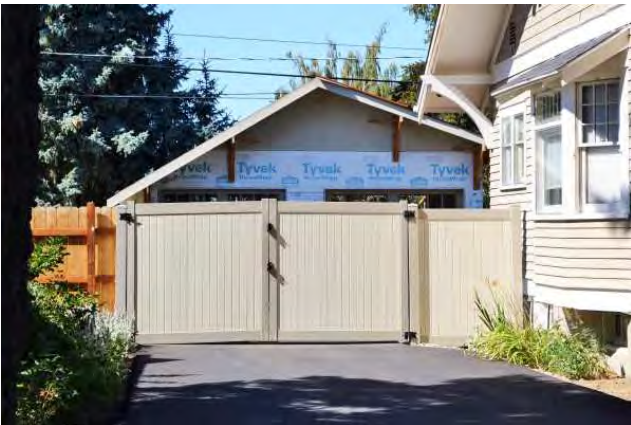
Garage, south (front) side, 2021. View to north.
