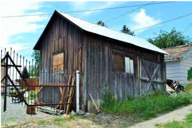
Outbuilding, east and north sides, 2021. To SW.
