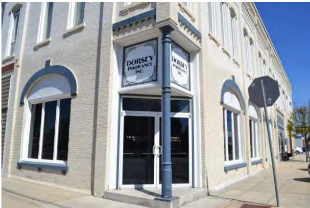
Main entrance at SW corner, 2021. View to NE.
