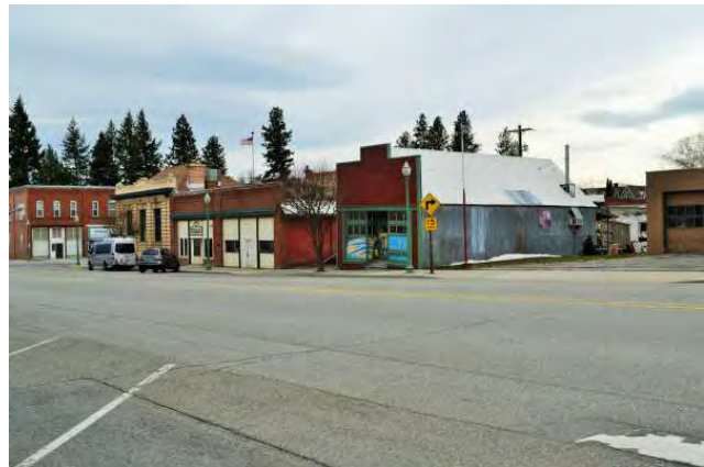
Overview from Chelan Ave./Hwy. 2, 2021. View to SW.
