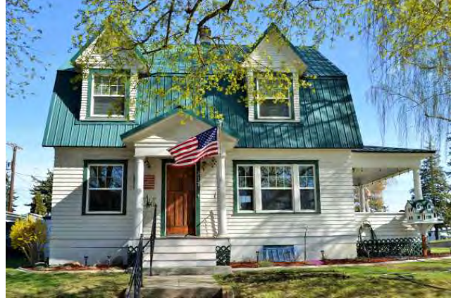
South (front) elevation, 2021. View to north.
