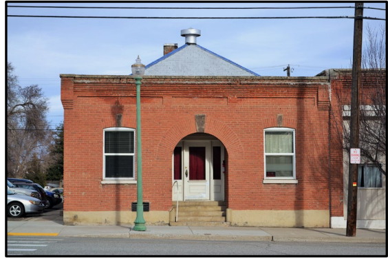
Figure 13. Simple 1913 Renaissance Revival hospital (Inventory Property #4); view to the east.
