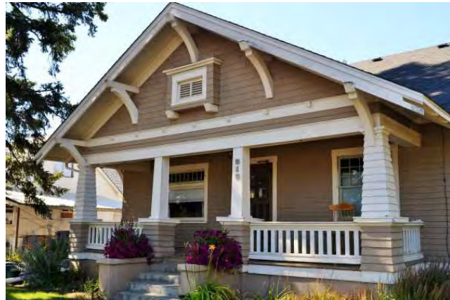
Front (south) porch, 2021. View to NW.
