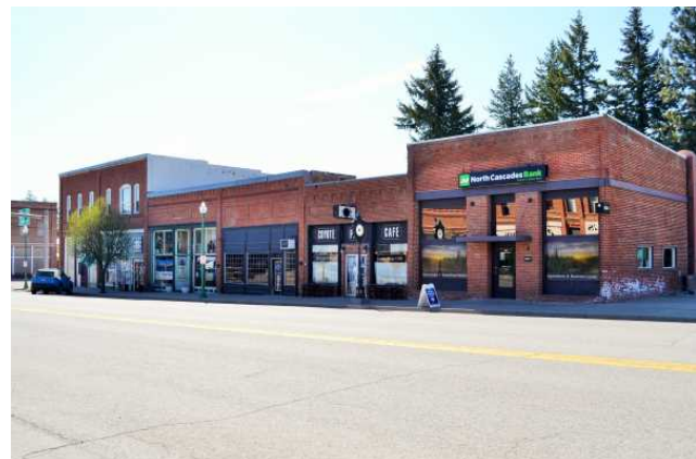
Overview from Locust St., 2021. View to SE.
