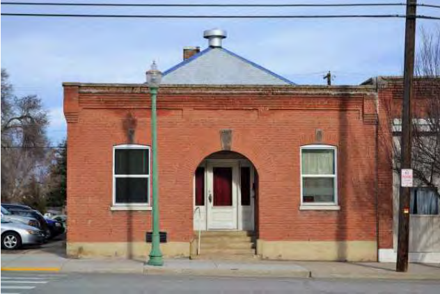
West (front) elevation, 2021. View to east.
