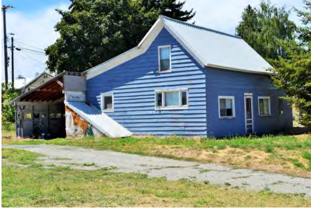
East and north (front) sides, 2021. View to SW.
