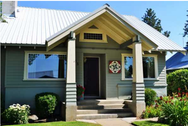
Front porch and windows, 2021. View to NE.
