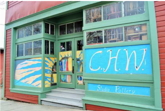
Main entrance and storefront, 2021. View to SW.
