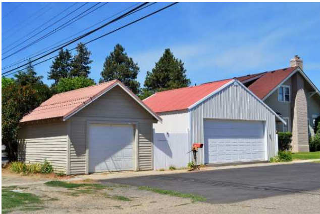
Historical and modern garages, 2021. View to NW.
