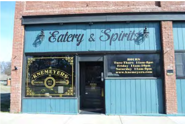
West storefront and entrance, 2021. View to north.
