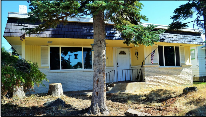
Figure A-14. Mansard style: Inventory Property #45, south/front side (the style represents a façade remodel; the original building's gables, dormers, and chimney remain readily visible from the sidewalk and street).
