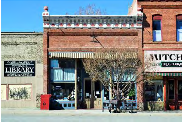
South (front) elevation, 2021. View to north.
