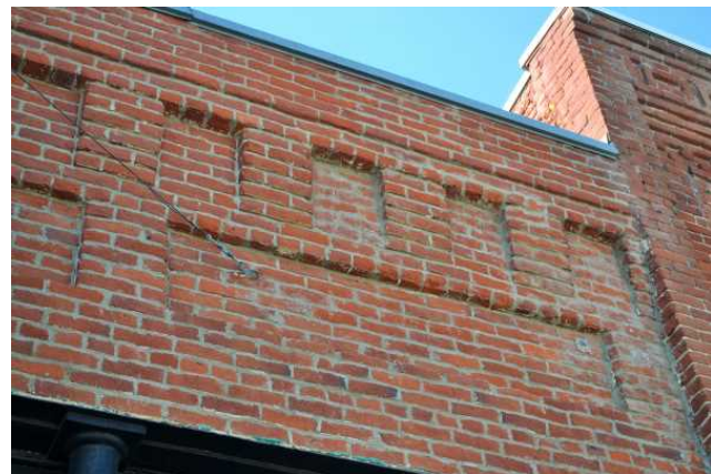
Brickwork, cornice, and parapet, 2021. View to SW.
