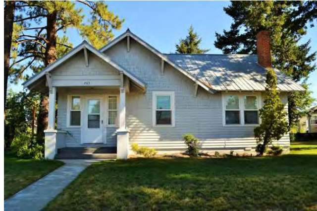
South (front) elevation, 2021. View to north.
