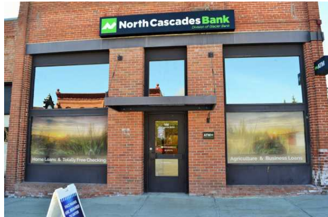
Modernized storefront, 2021. View to south.
