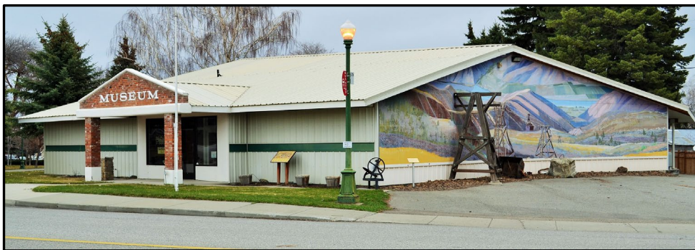
Figure A-12. Undifferentiated Modernist architecture: Inventory Property #29, northwest/front and southwest sides (the 1959 building has been extensively remodeled).
