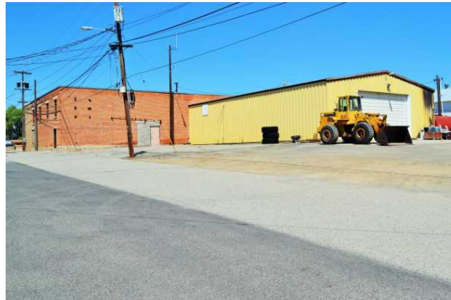
West and south (rear) sides, 2021. View to NE.
