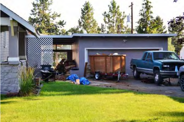
Garage, south (front) side, 2021. View to north.
