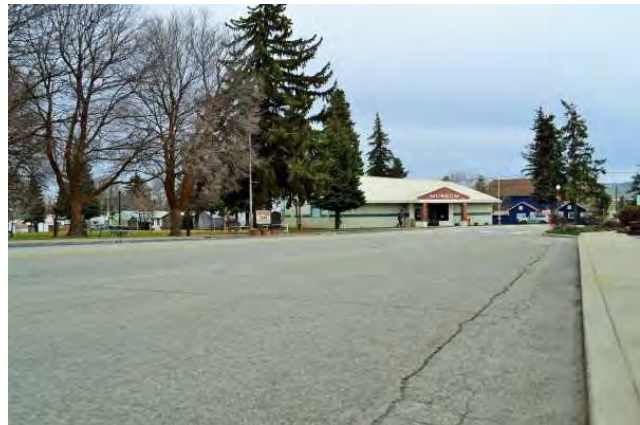
Overview from Central Ave./Hwy. 2, 2021. To south.
