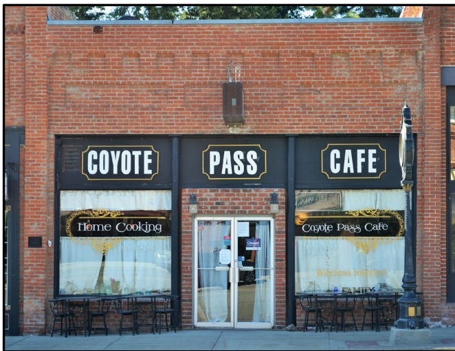
Figure A-9. Commercial Vernacular form: Inventory Property #19, north/front elevation (recessed entry has been rebuilt).
