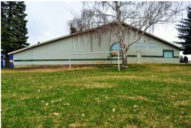
NE and SE sides (rear), 2021. View to SW.
