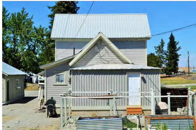
South (rear) elevation, 2021. View to north.
