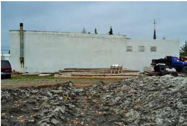
West elevation, 2021. View to east.
