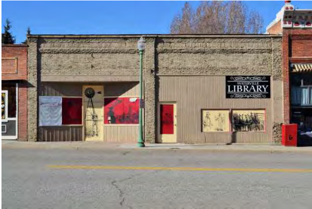
South (front) elevation, 2021. View to north.
