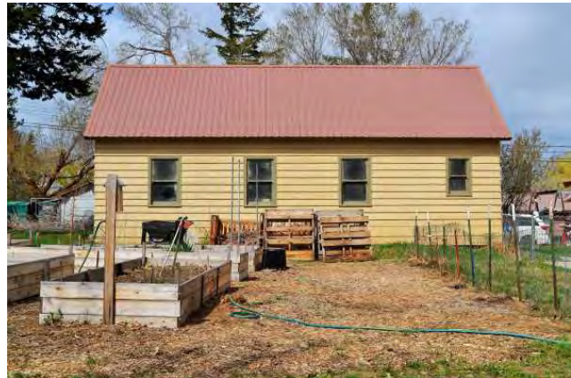
South elevation, 2021. View to north.
