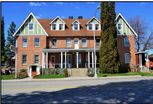
Figure 18. 1903 Tudor Revival hotel (Inventory Property #17); view to west.
