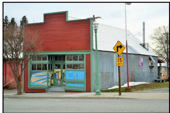
Figure 15. Ca. 1907 wood frame false front commercial building (Inventory Property #7); view to the southwest.
