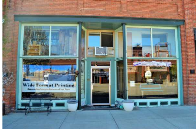
Storefront and entrance, 2021. View to south.
