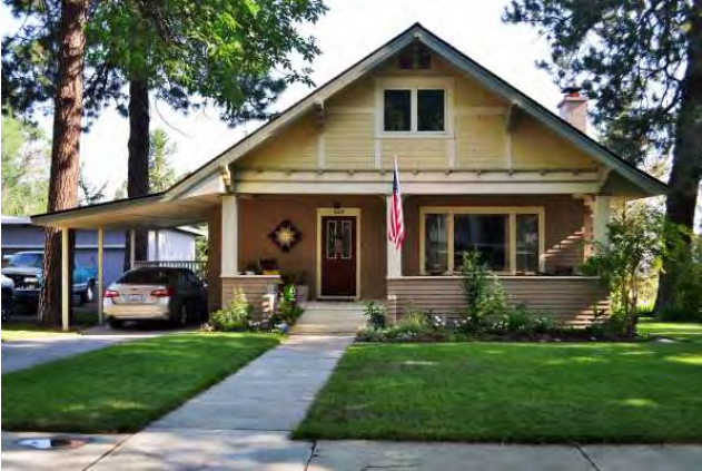
South (front) elevation, 2021. View to north.
