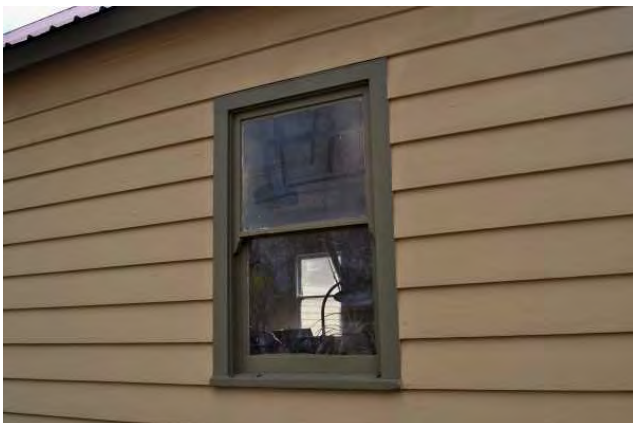
Window on north side, 2021. View to SE.
