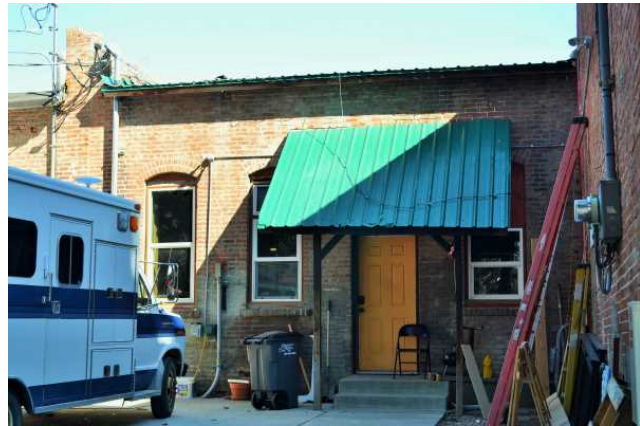
South (rear) elevation, 2021. View to north.
