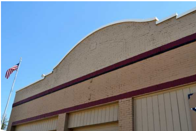
East shaped parapet, 2021. View to SE.
