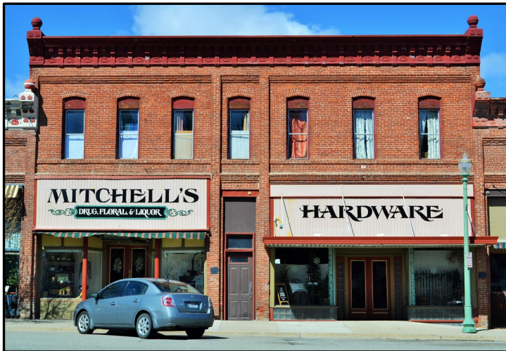
Figure A-1. Italianate style: Inventory Property #11, south/front facade.
