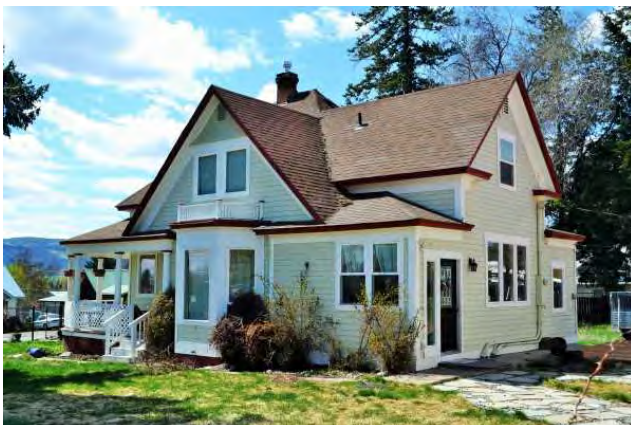
East and north (rear) sides, 2021. View to SW.
