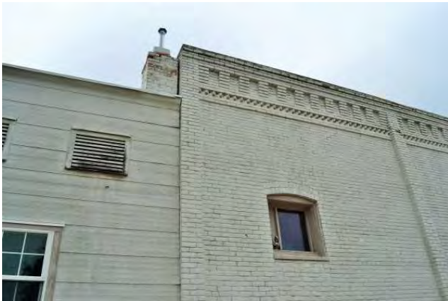
Original building (R), addition (L), 2021. View to NW.
