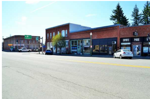
Overview from Locust St., 2021. View to SE.
