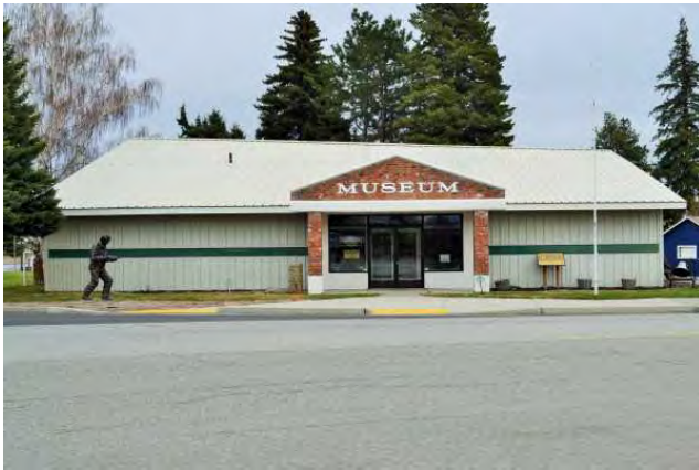
NW (front) elevation, 2021. View to SE.
