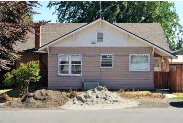
North side and cross-gabled extension, 2021. To south.
