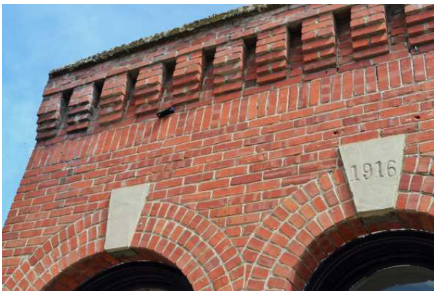
Brickwork, cornice, and parapet, 2021. View to NE.
