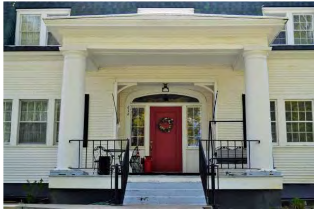
Front porch and door, 2021. View to south.
