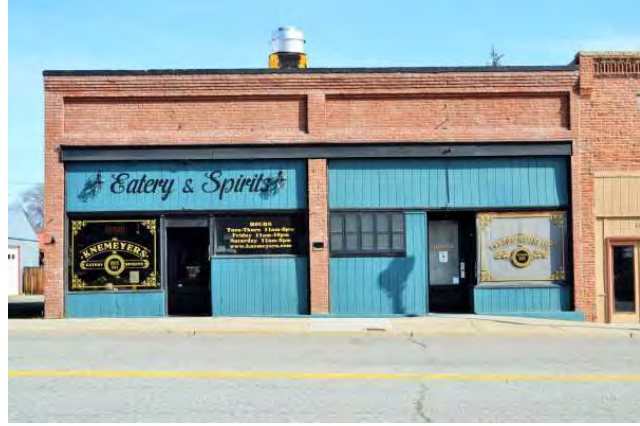
South (front) elevation, 2021. View to north.
