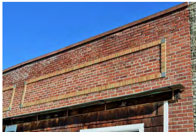
Upper wall brickwork and parapet, 2021. View to NW.
