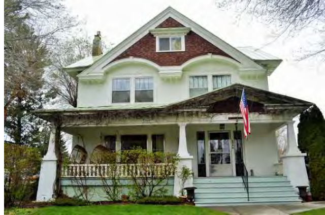
East (front) elevation, 2021. View to west.
