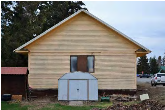
South elevation, 2021. View to north.
