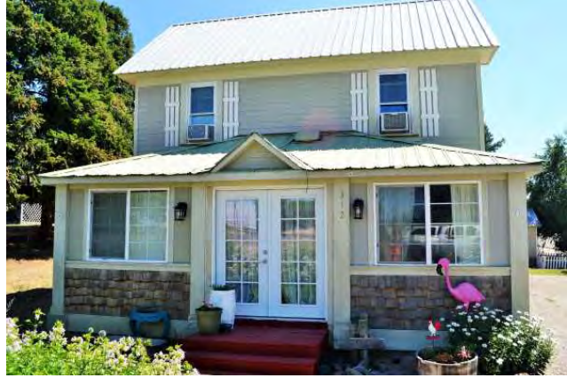
North (front) elevation, 2021. View to SE.
