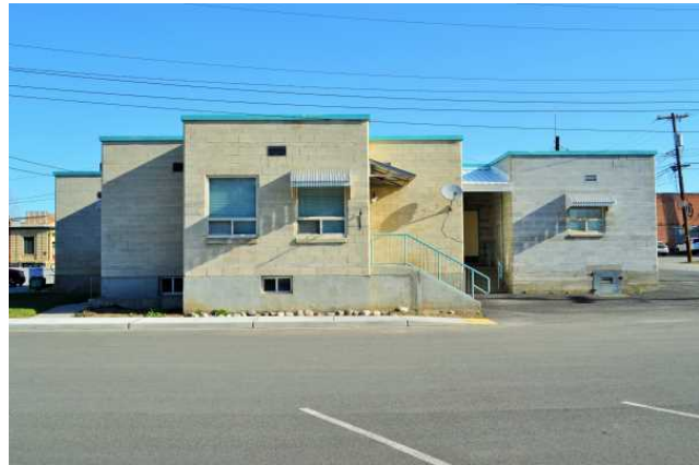
South elevation, 2021. View to north.
