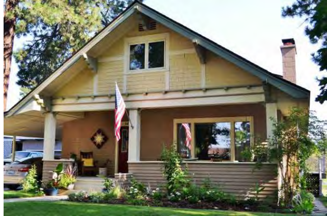
Detail of main (south) facade, 2021. View to NW.
