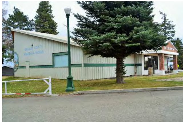
NE and NW (front) sides, 2021. View to south.
