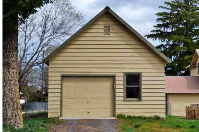
West (front) elevation, 2021. View to east.
