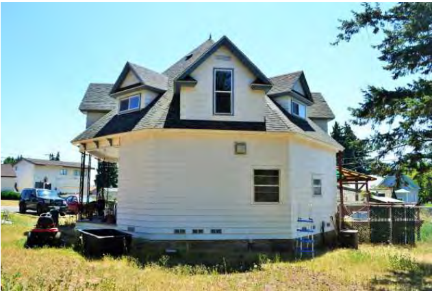
NW side, 2021. View to SE.
