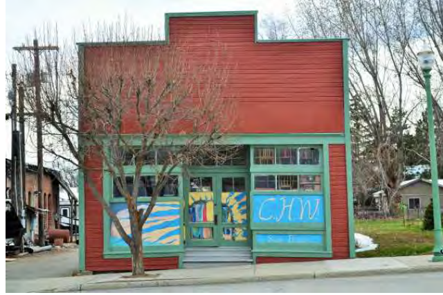
East (front) elevation, 2021. View to west.
