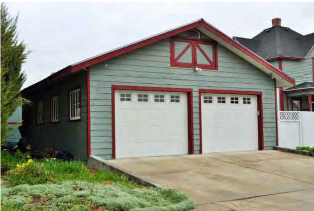
Garage, west and south (front) sides, 2021. View to NE.
