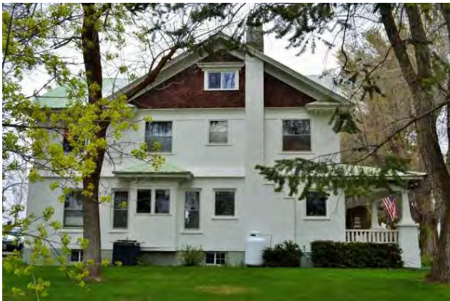
South elevation, 2021. View to north.
