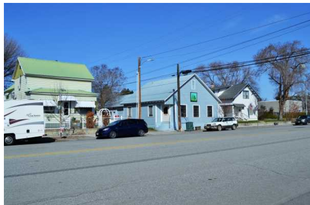
Overview from Chelan Ave., 2021. View to NW.
