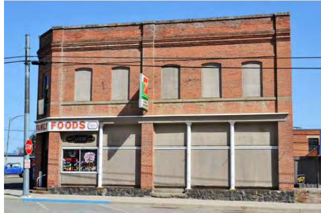
West side, 2021. View to east.
