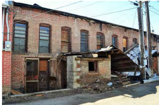
North (rear) side, 2021. View to SW.
