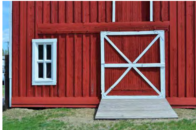
Front (west) door and window, 2021. View to east.
