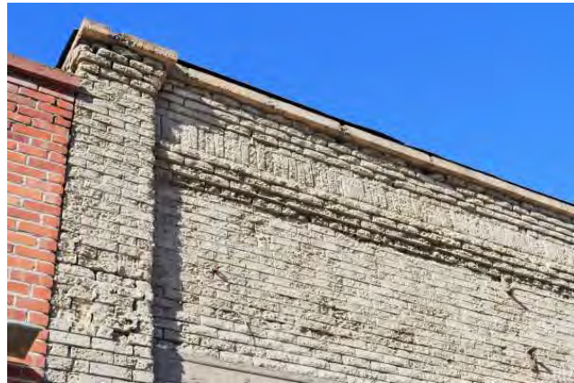
Upper wall and parapet, 2021. View to NE.
