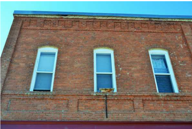
Main facade windows and cornice, 2021. View to south.
