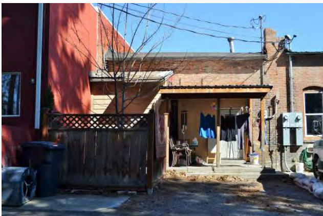
South (rear) elevation, 2021. View to north.
