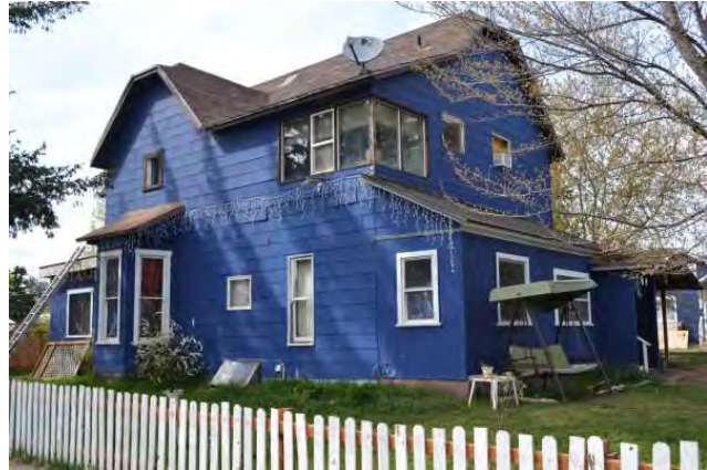
South and east (rear) sides, 2021. View to NW.
