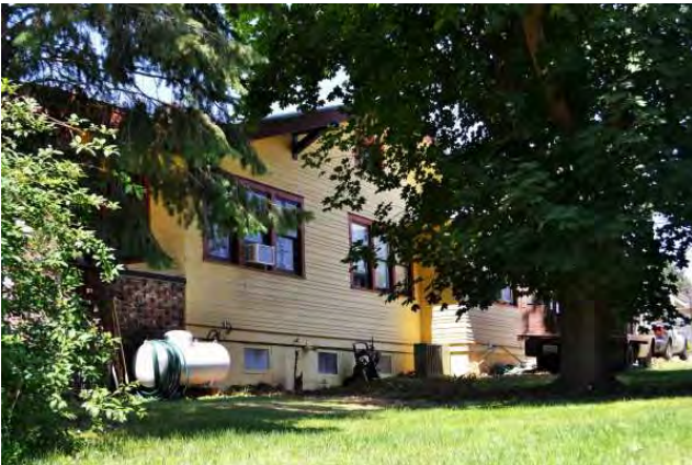
East side, 2021. View to NW.
