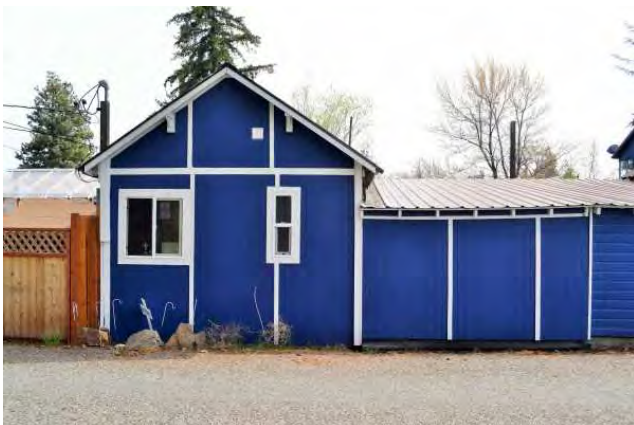
North (rear) of fifth cabin from west, 2021. To south.
