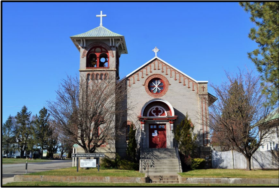
Figure 12. 1916 Romanesque Revival church (Inventory Property #1); view to the north.
