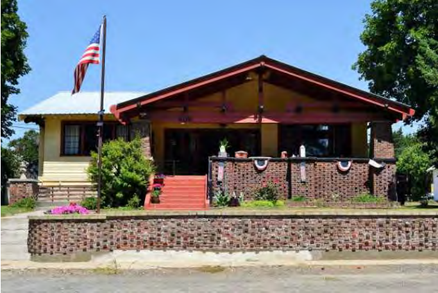
South (front) elevation, 2021. View to north.
