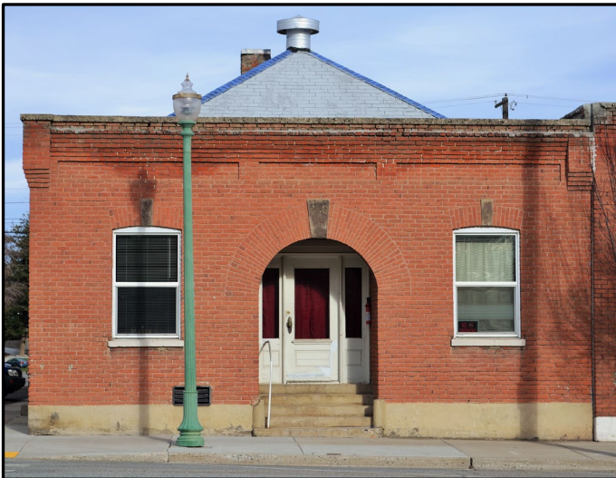
Figure A-6. Renaissance Revival style: Inventory Property #4, west/front elevation.
