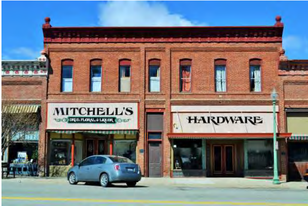
South (front) elevation, 2021. View to north.
