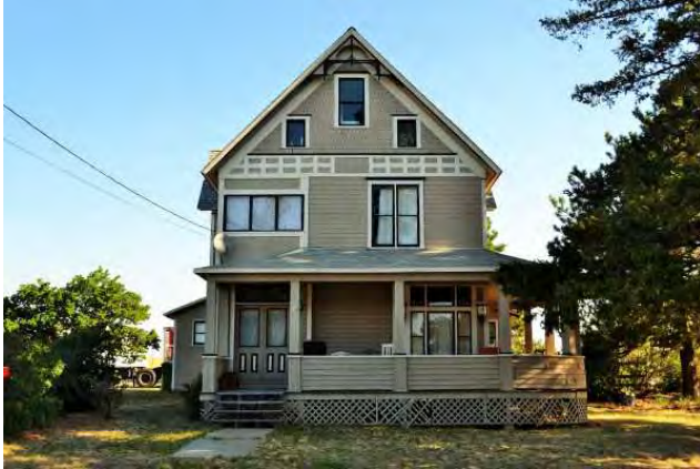
South (front) elevation, 2021. View to north.
