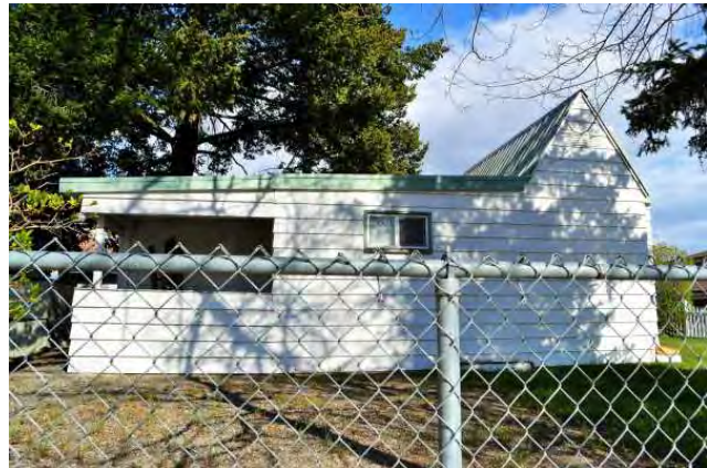
West elevation, 2021. View to east.
