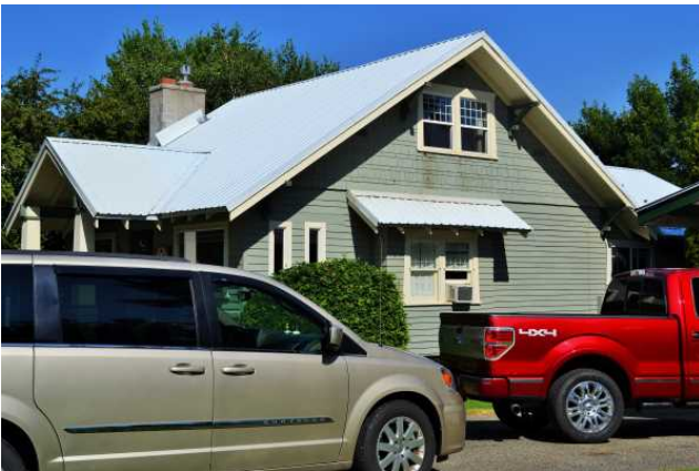
East side, 2021. View to NW.
