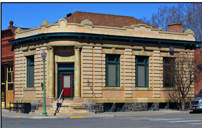
Figure A-8. Neoclassical style: Inventory Property #8, south and east sides.
