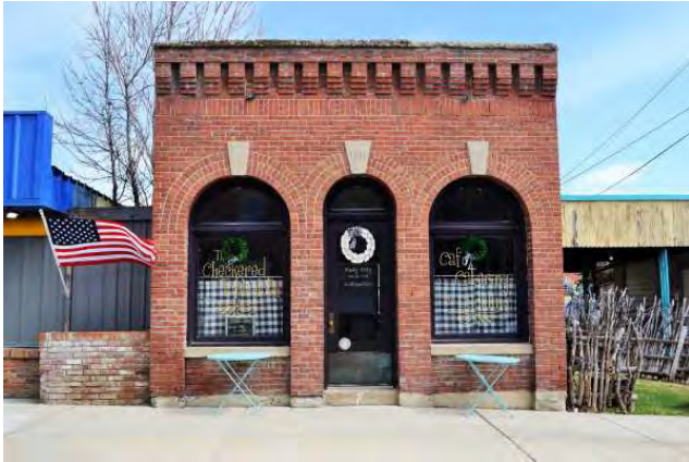
West (front) elevation, 2021. View to east.
