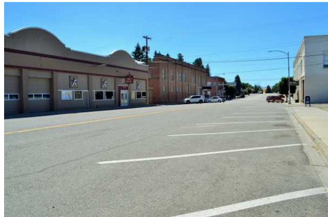
Overview from Locust-Baker intersection, 2021. To SW.
