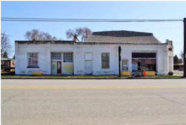
West elevation, 2021. View to east.
