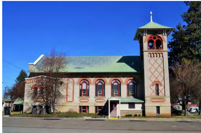
West elevation, 2021. View to east.
