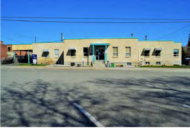
West (front) elevation, 2021. View to east.
