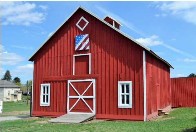
West (front) and south sides, 2021. View to NE.
