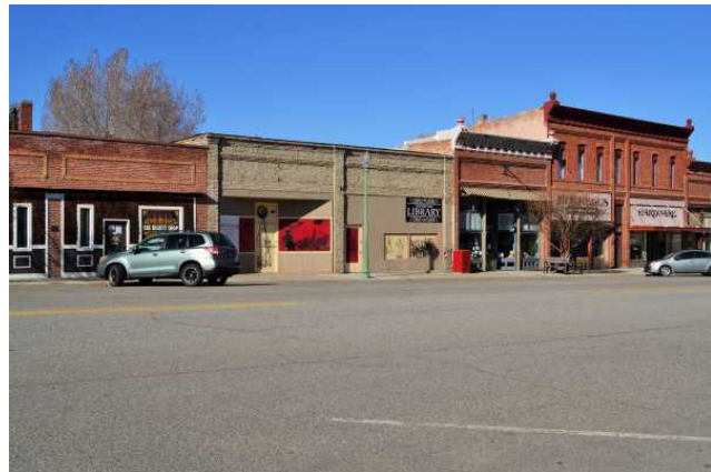
Overview from Locust St., 2021. View to NE.
