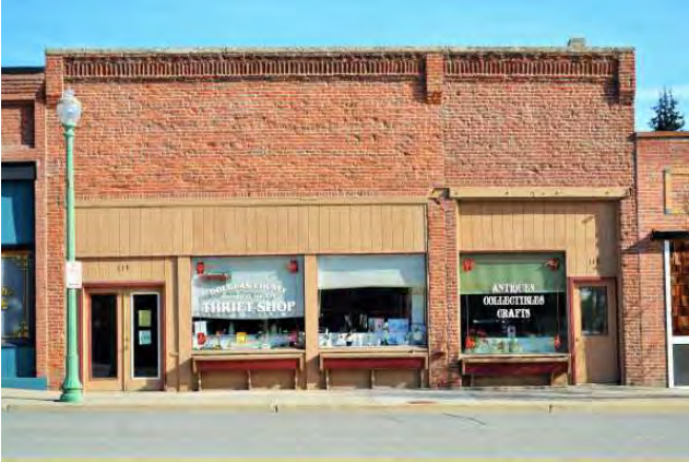
South (front) elevation, 2021. View to north.
