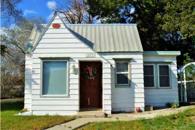
South (front) elevation, 2021. View to north.
