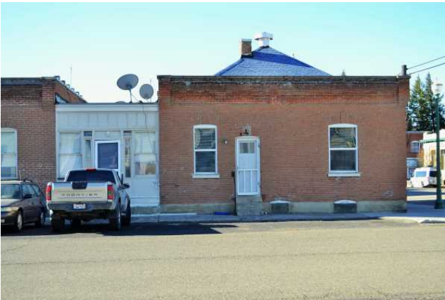
North side of front section, 2021. View to south.
