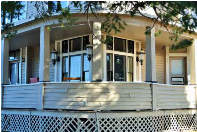
SE corner of front porch, 2021. View to NW.
