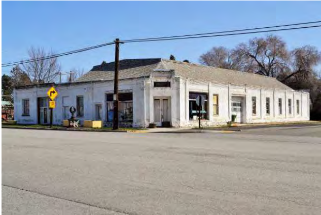
West and south sides, 2021. View to NE.
