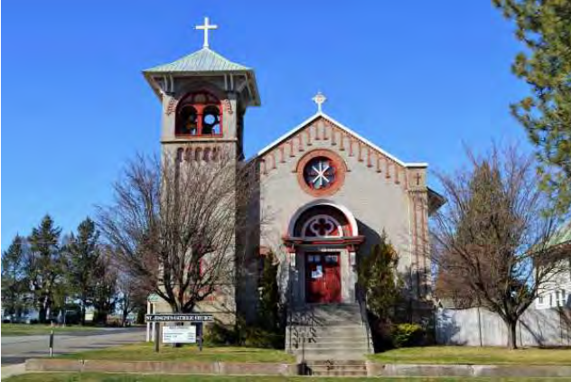
South (front) elevation, 2021. View to north.
