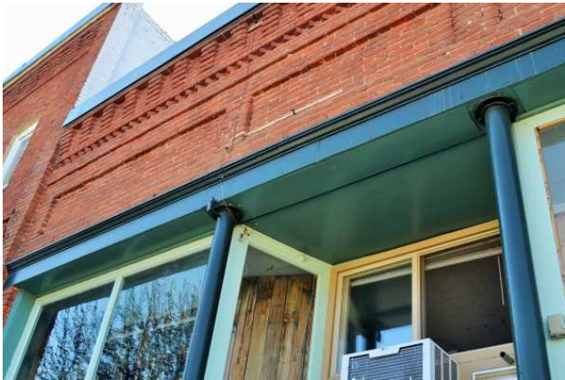
Columns and upper facade brickwork, 2021. To SE.
