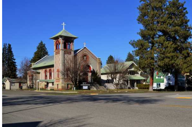
Overview from Chelan-Poplar intersection, 2021. To NE.
