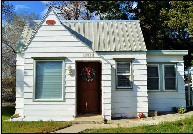
Figure A-7. Tudor Revival style: Inventory Property #33, south/front elevation.
