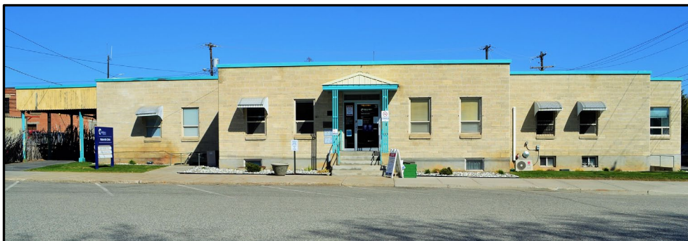
Figure A-13. Art Moderne style: Inventory Property #25, west/front elevation.
