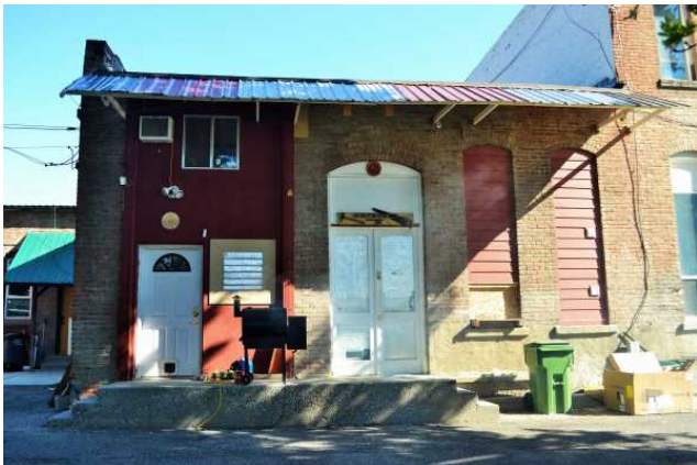
South (rear) elevation, 2021. View to north.
