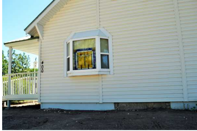
Remnant of original front porch, 2021. View to SE.
