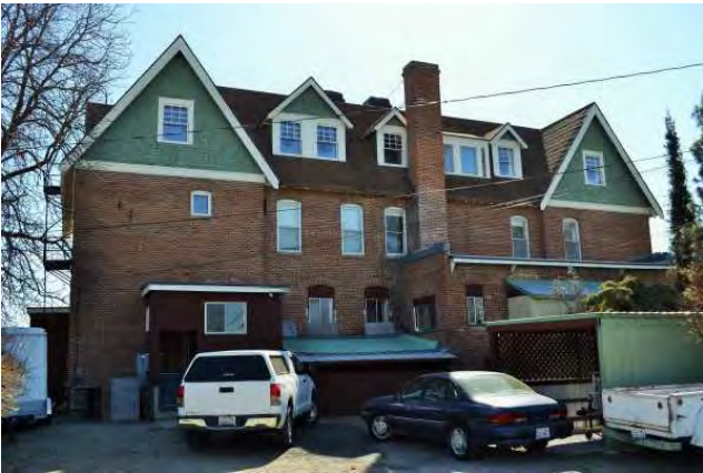
West (rear) elevation, 2021. View to SE.
