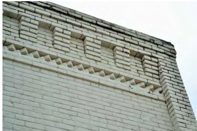
East side brick cornice, 2021. View to NW.
