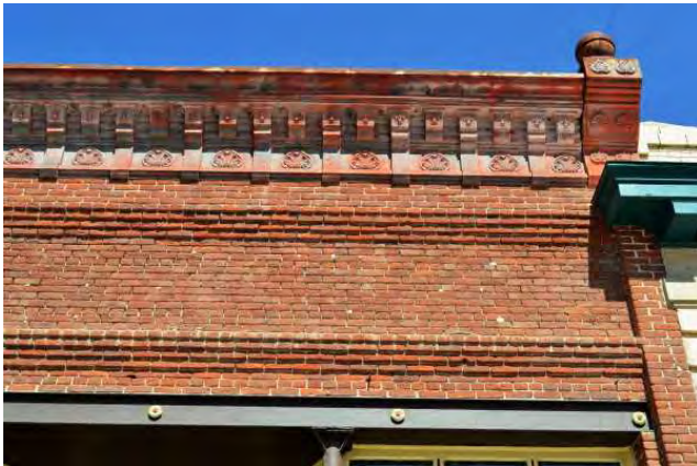
East upper wall and cornice, 2021. View to north.
