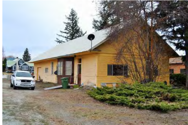
East (front) and north sides, 2021. View to SW.
