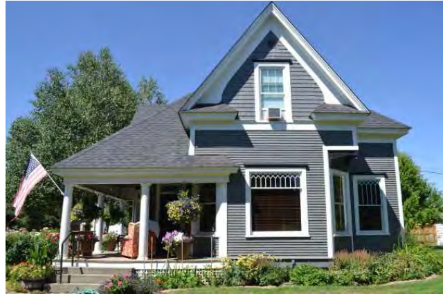
South (front) elevation, 2021. View to north.
