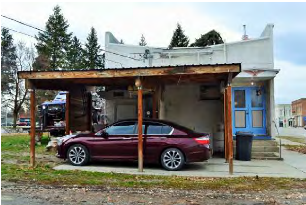
South (rear) elevation, 2021. View to north.
