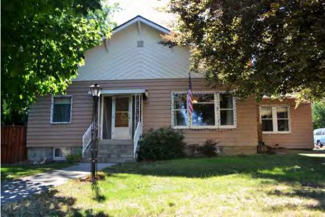
East (front) elevation, 2021. View to west.
