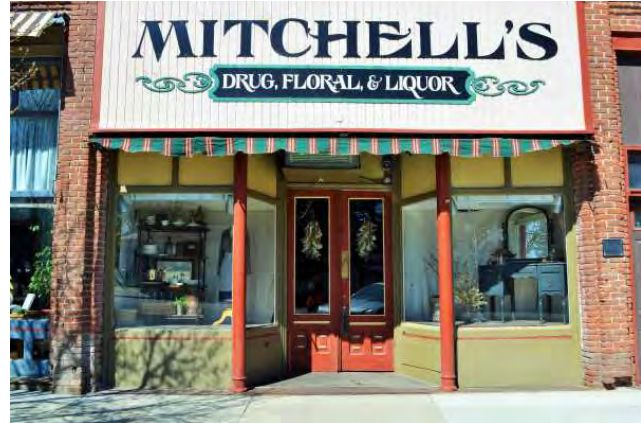
West storefront, 2021. View to north.
