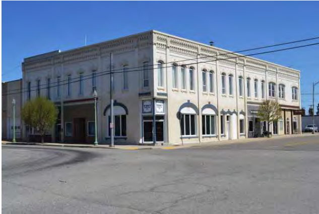
West and south sides, 2021. View to NE.
