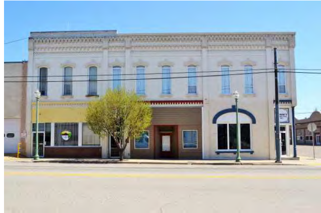
West elevation, 2021. View to east.
