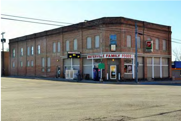
North and west sides, 2021. View to SE.
