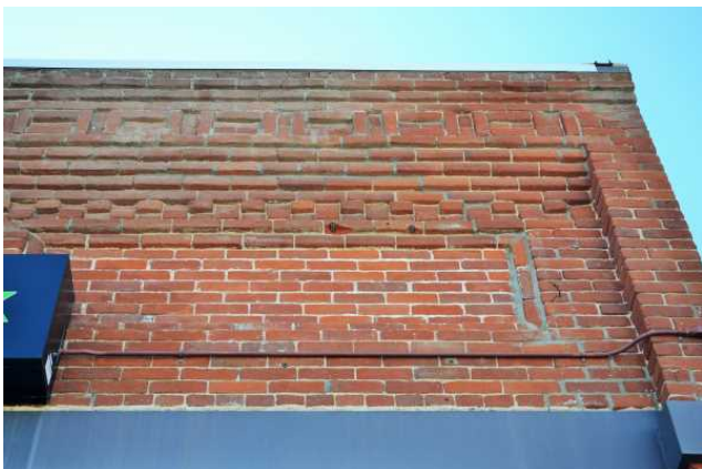
Upper facade brickwork and cornice, 2021. To south.
