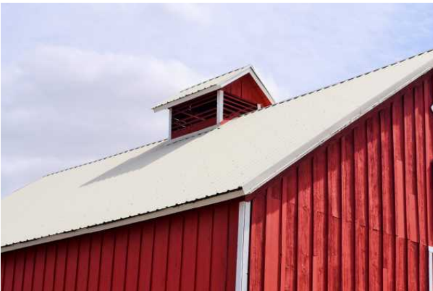
Cupola, north and west sides, 2021. View to SE.
