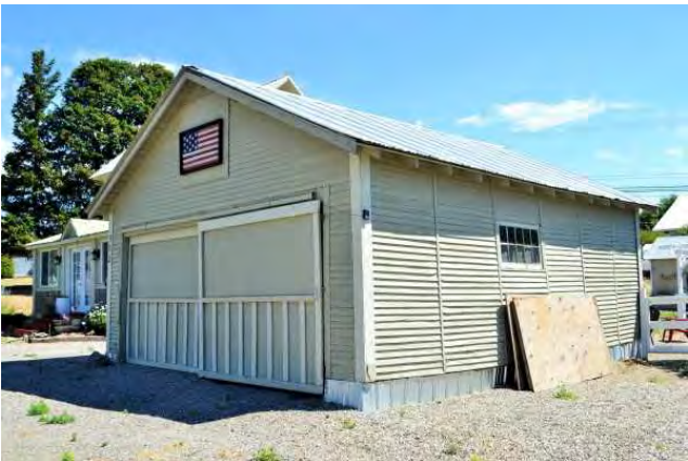
Garage, north (front) and west sides, 2021. To SE.
