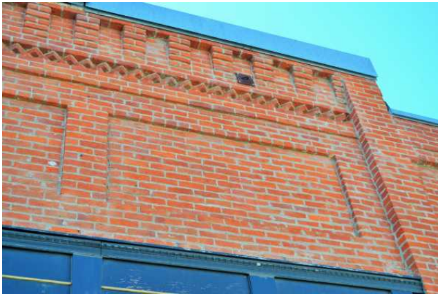
Upper facade brickwork and cornice, 2021. To SW.
