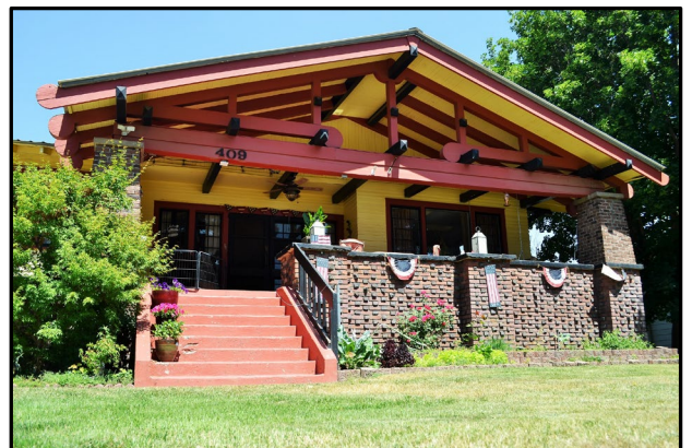
Figure 21. Ca. 1913 Craftsman residence (Inventory Property #52); view to northeast.
