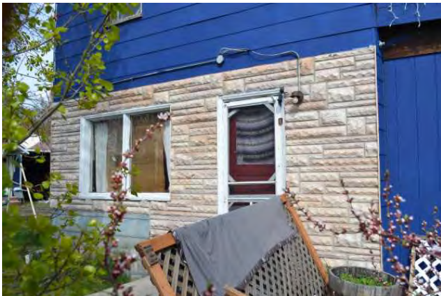
Main (west) entrance and window, 2021. View to NE.
