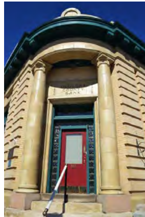
Canted corner entry, 2021. View to NW.
