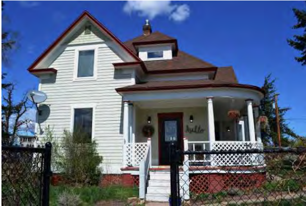
South (front) elevation, 2021. View to north.
