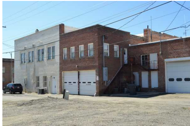
East and north sides, 2021. View to SW.
