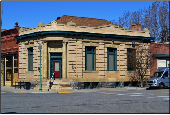
Figure 16. 1911 Neoclassical bank building (Inventory Property #8); view to the northwest.
