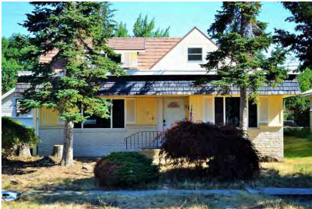
South (front) elevation, 2021. View to north.
