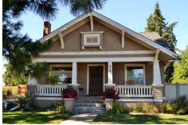
South (front) elevation, 2021. View to north.
