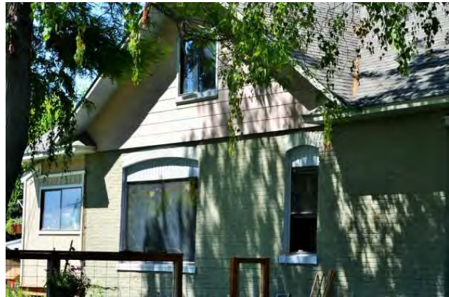
East side windows and gable, 2021. View to SW.
