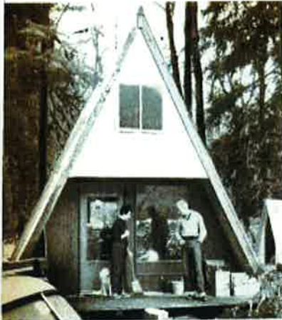
THIS PREFAB CABIN comes as a kit, has no structural beams except in the foundation. Floor and walls are stressed-skin panels of plywood over two-by-four frames with built-in insulation. Standard size is 16' by 24' with 9'-by-12" sleeping loft for $2,300. Additional panels are available for extending the cabin to any length. The kit is sold by Sandpoint Builders Supply, Mountlake Terrace, Seattle, Wash.
