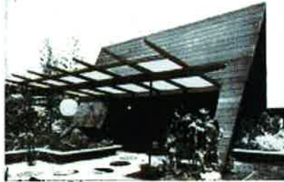
THIS PREFAB CABIN comes as a kit, has no structural beams except in the foundation. Floor and walls are stressed-skin panels of plywood over two-by-four frames with built-in insulation. Standard size is 16' by 24' with 9'-by-12" sleeping loft for $2,300. Additional panels are available for extending the cabin to any length. The kit is sold by Sandpoint Builders Supply, Mountlake Terrace, Seattle, Wash.
